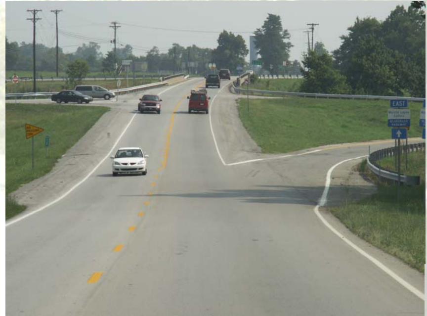
Very soon, the bridge at the Blue Grass Parkway Interchange will be widened to four lanes
