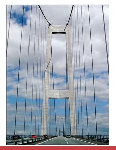
Portal Tower with Cables on Outside of Deck
