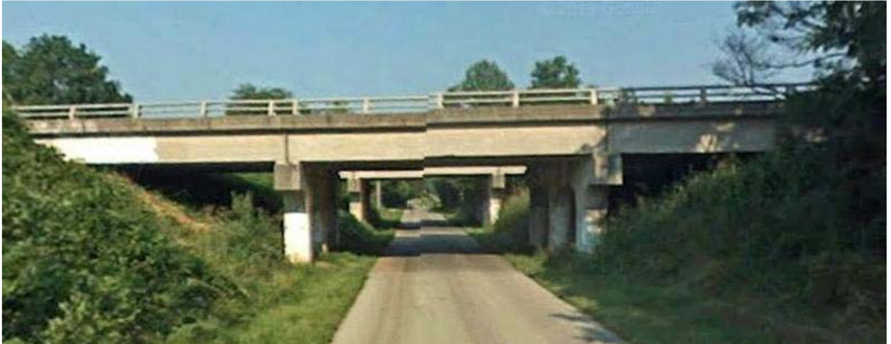
Existing Rhudes Creek Road Bridge
