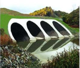
Examples of mitered culvert design
