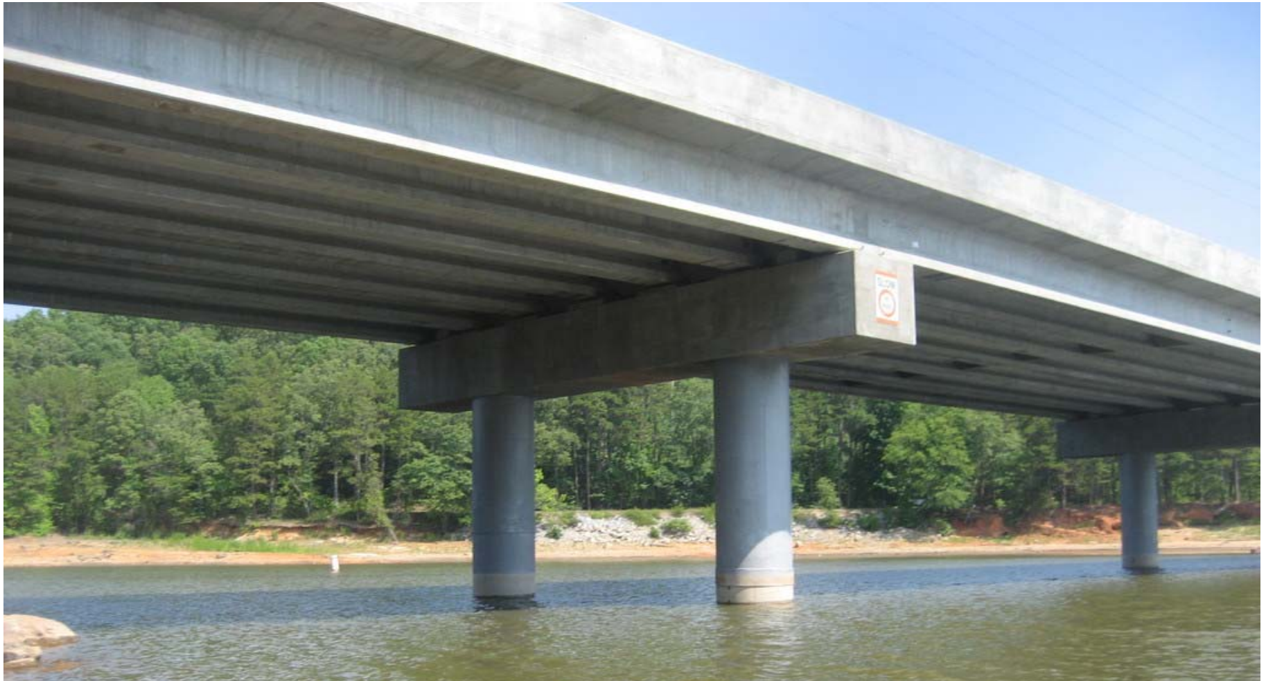
Photograph of Conventional Cap and Column Bridge Piers
