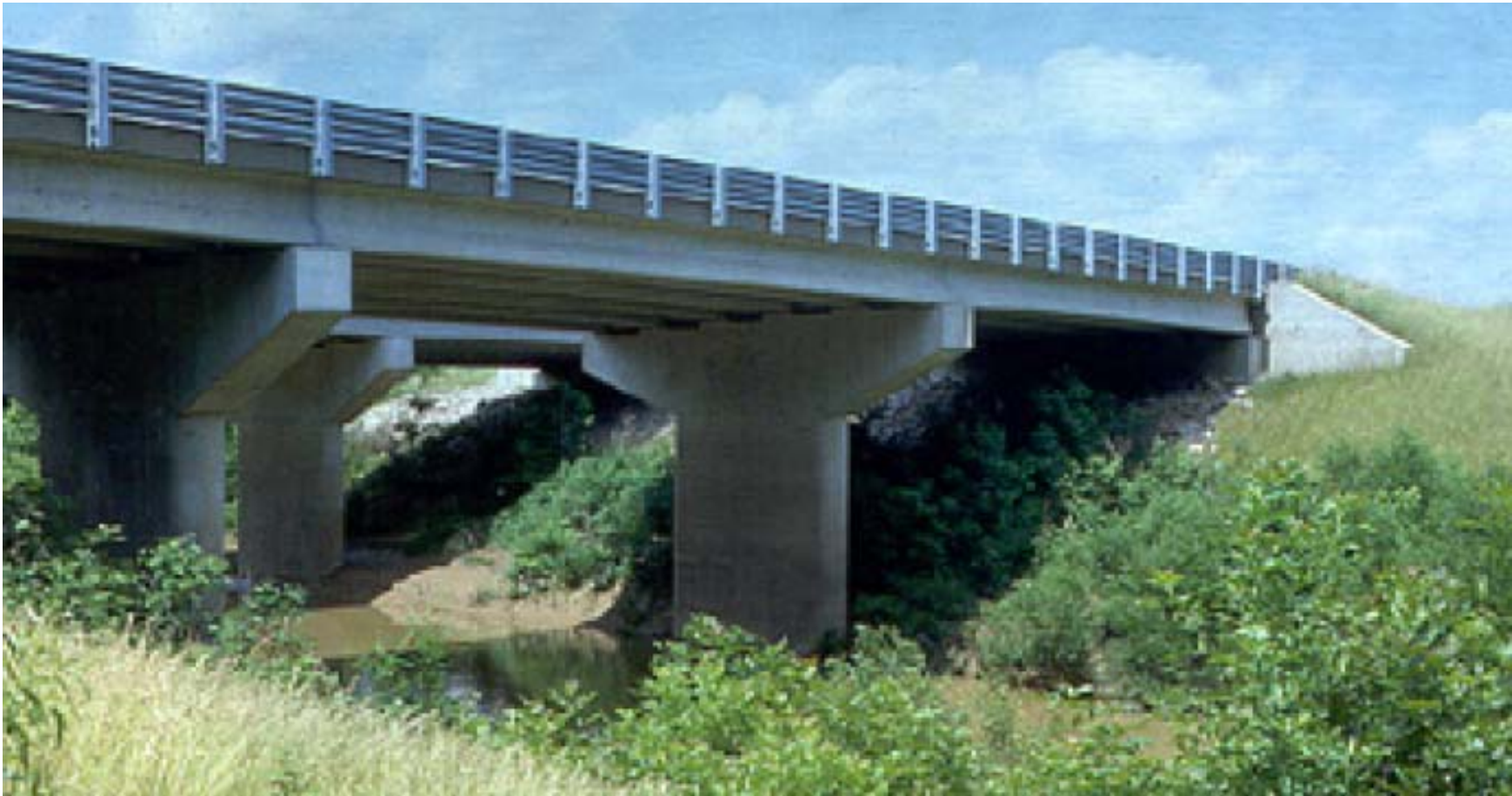
Photograph of Hammerhead Bridge Piers
