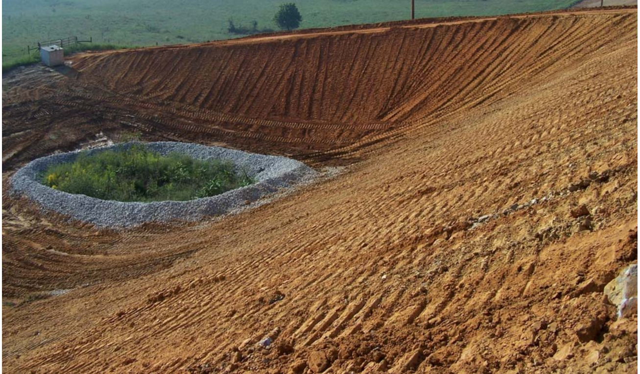
SINKHOLE WITH PROTECTION
