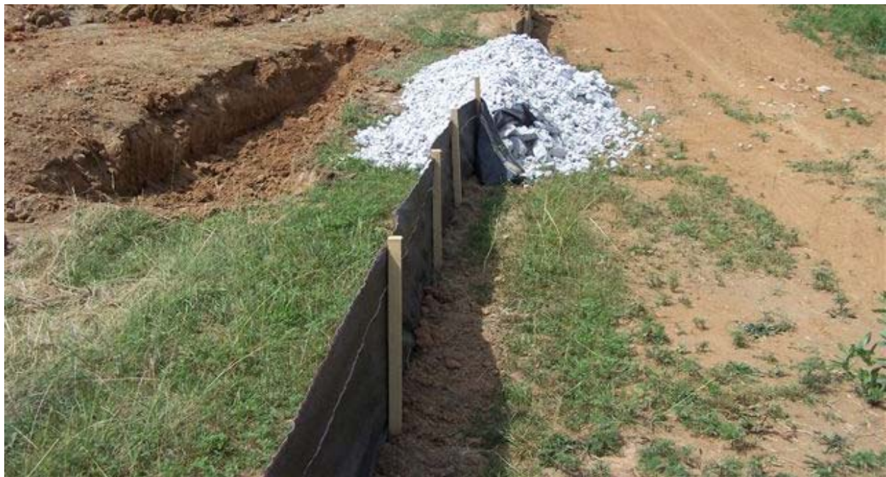
PLACING SILT FENCE AND COVERING WITH ROCK
