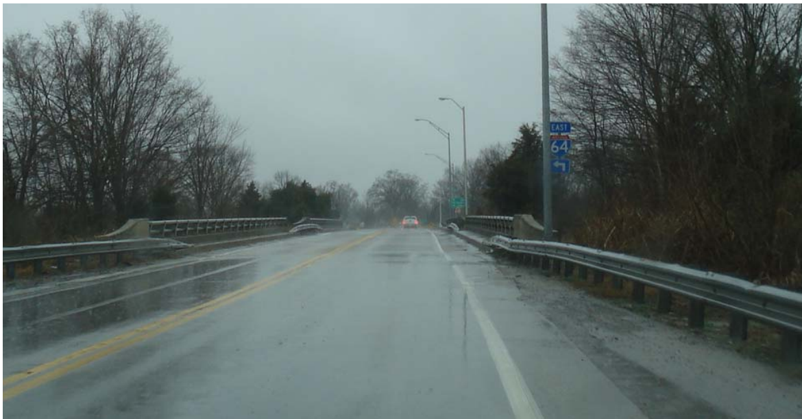
EXISTING KY 395 BRIDGE OVER I-64
