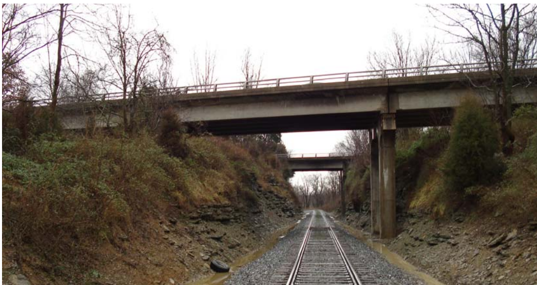
EXISTING I-64 BRIDGE OVER NORFOLK SOUTHERN RR (LOOKING NORTH)
