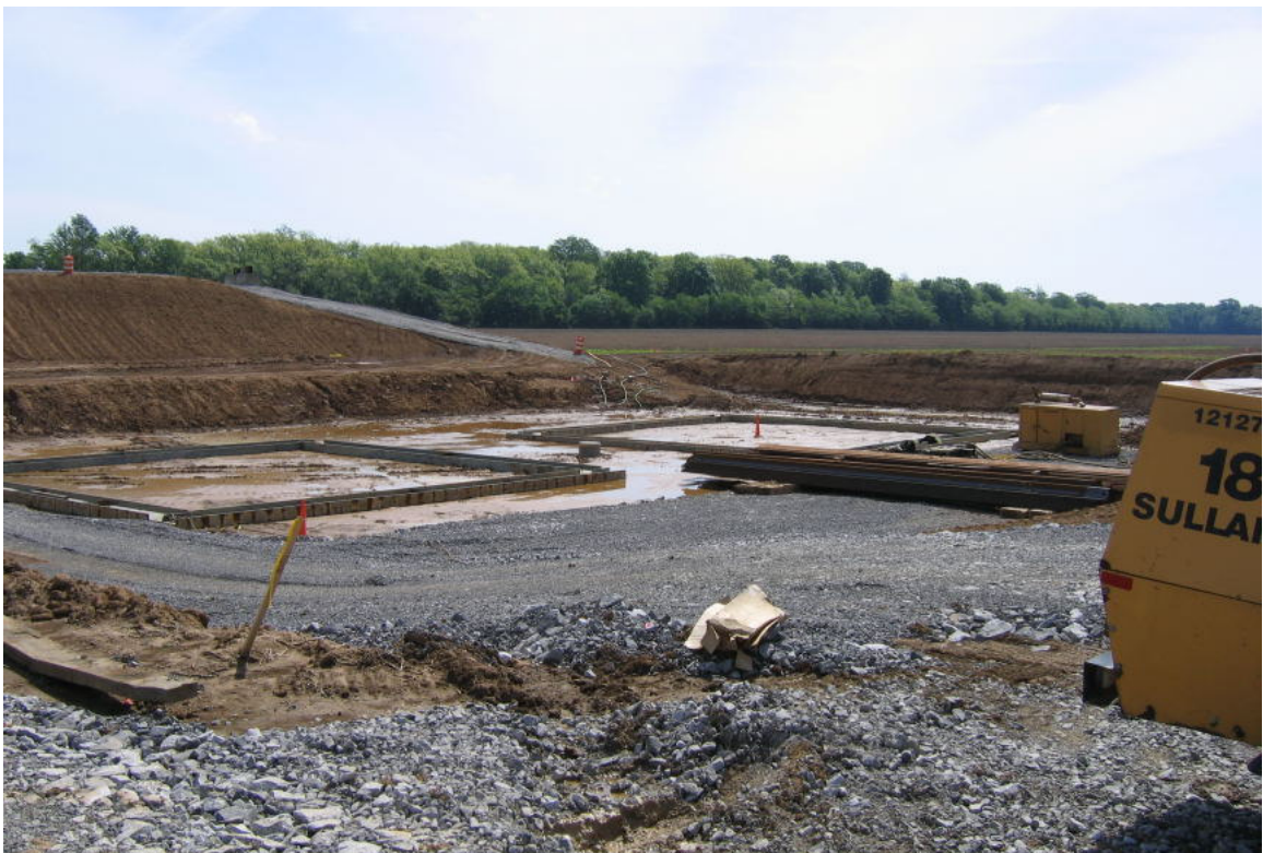
Site Picture 4: Cleared site ready for pier construction
