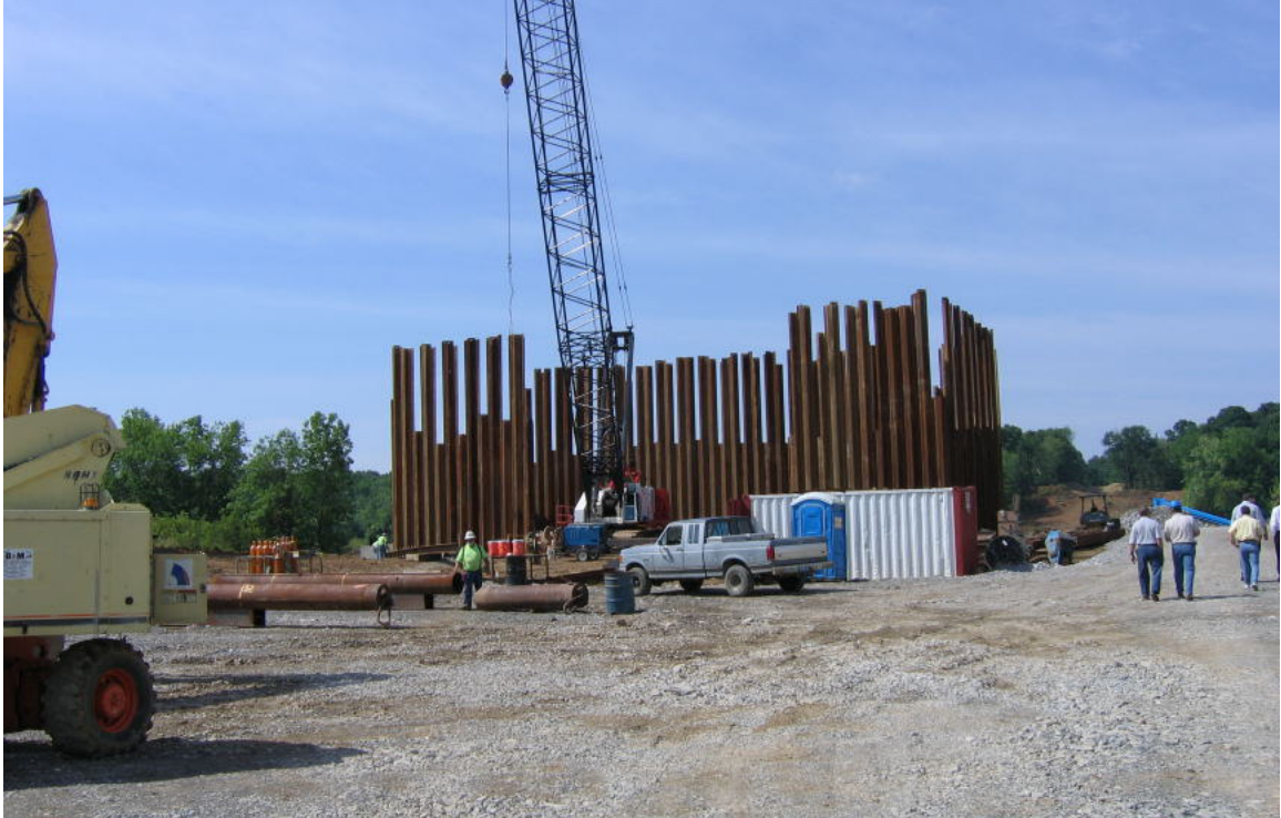
Site Picture 3: Driven piling for pier construction
