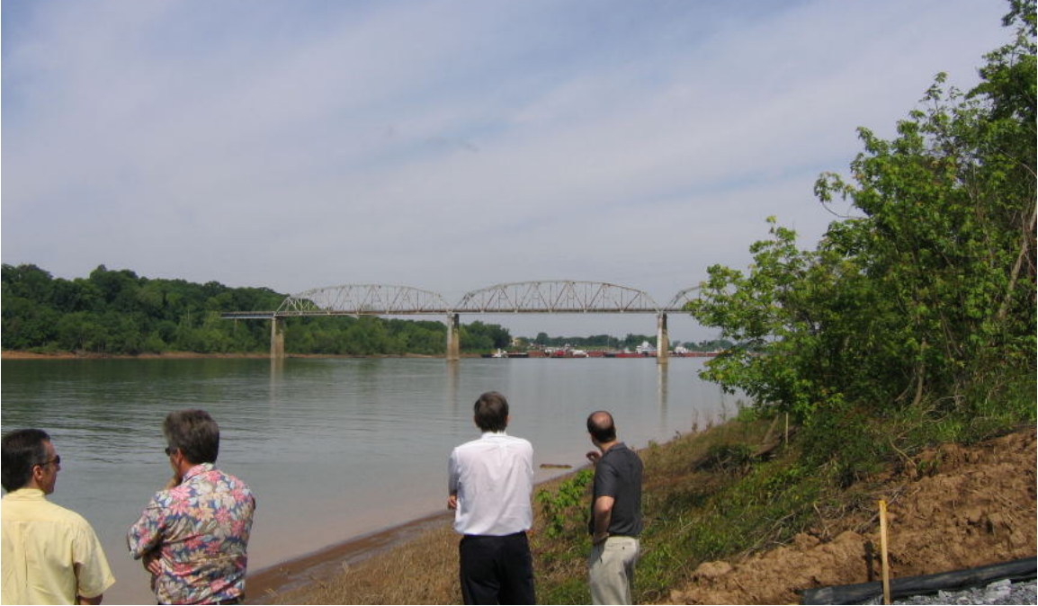
Site Picture 1: Existing US 60 Bridge over the Tennessee River
