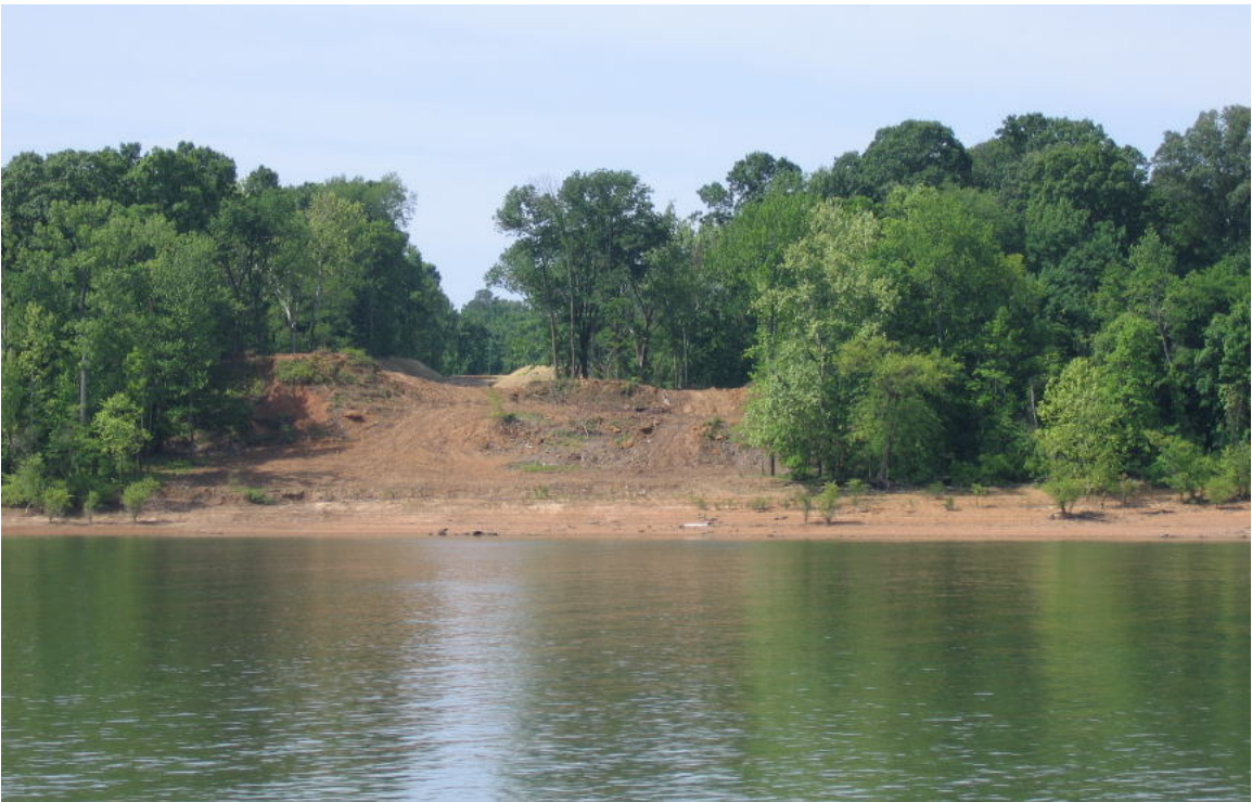
Site Picture 2: Ground breaking/clearing on riverbank in preparation for pier construction
