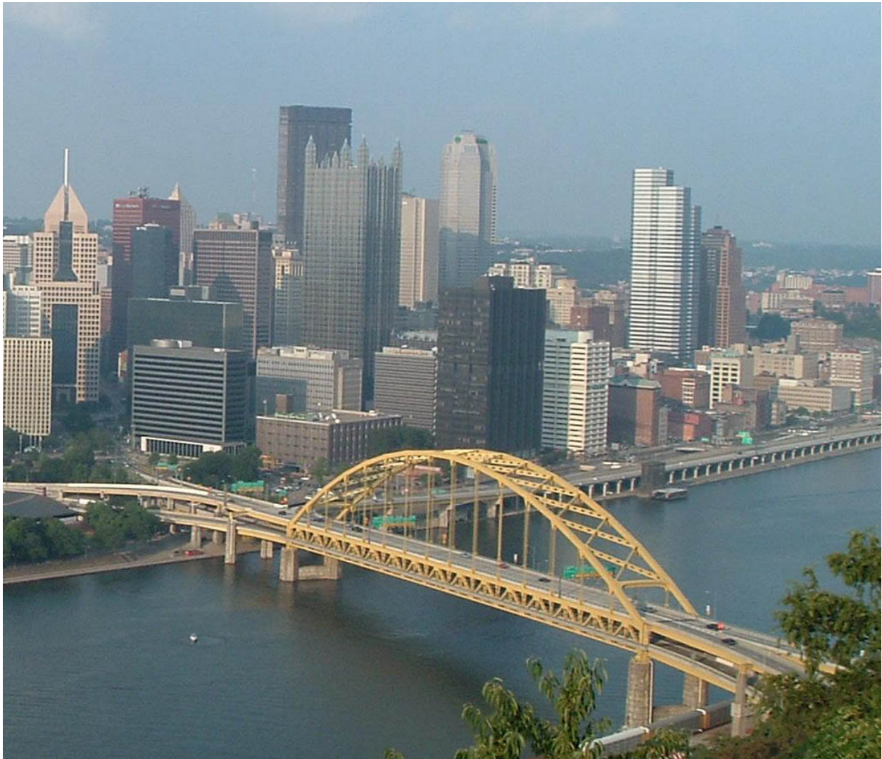
TIED ARCH MAINSPAN WITH STEEL PLATE GIRDER FLANKING SPANS (ALTERNATE 4)
