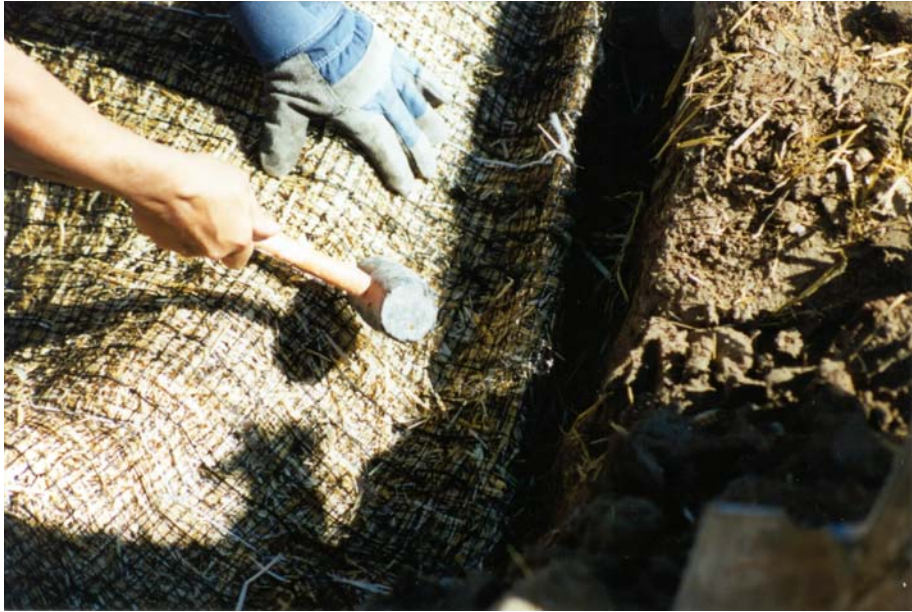
Slope Step Four – Secure the RECP in the Anchor Trench
