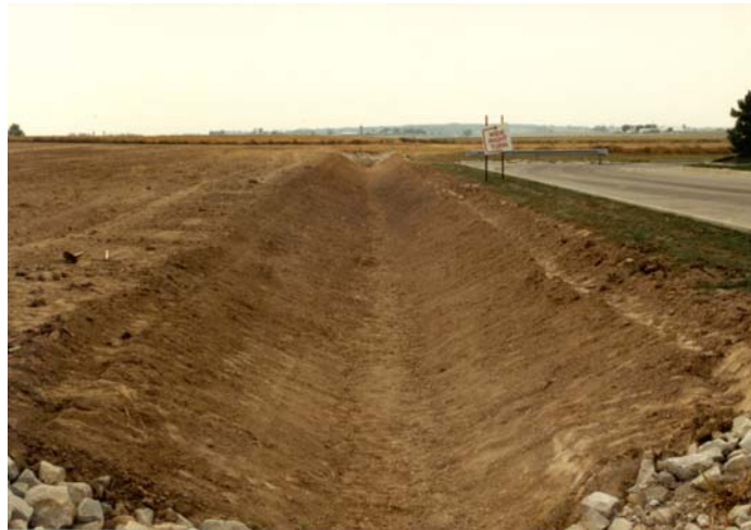
Channel Step One – Site Preparation
