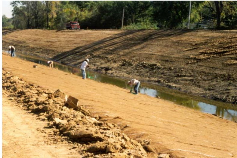
Alternative Channel Installation Method
