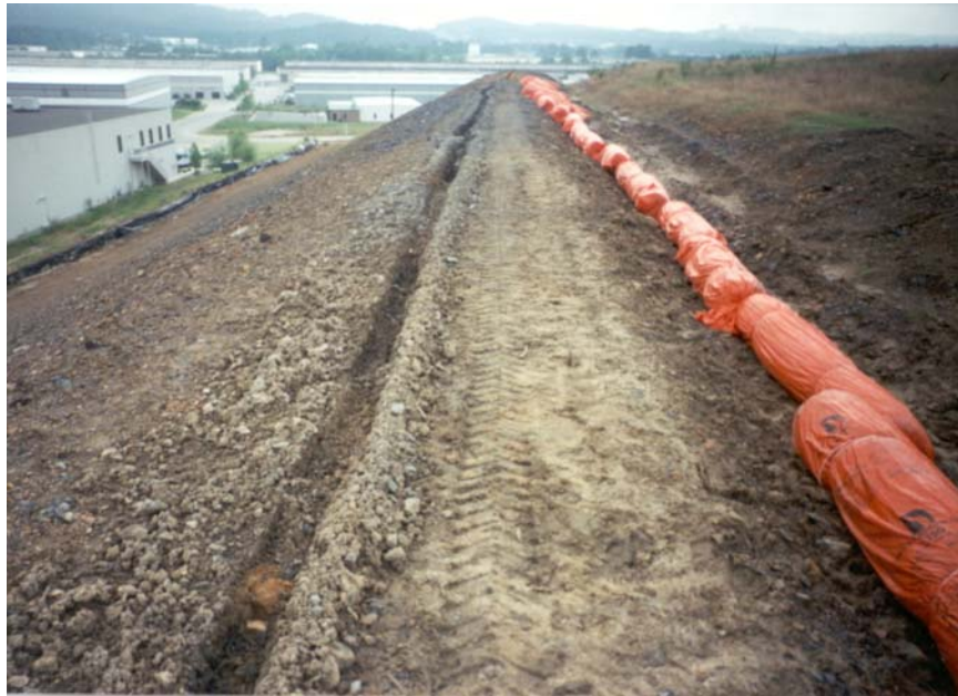
Slope Step Three – Prepare the Anchor Trench
