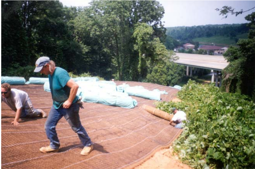
Slope Step Five –RECP Deployment
