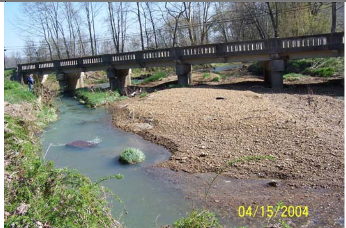
Loose rock and sediment may deposit at culvert and bridge openings and should be removed to prevent misalignment of the stream and erosion of the structures and nearby roadway.
