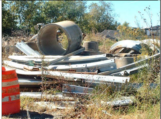
Concrete may be reused as road fill or in gabion baskets. Metal guardrails can be straightened.
