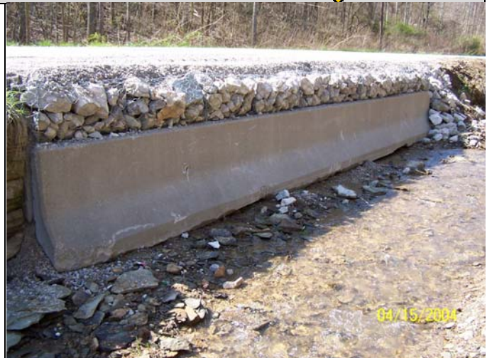
Embankment repair using movable concrete barrier walls and channel lining prevents erosion of the embankment and roadway collapse along a stream.
