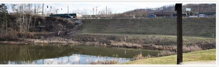
The west embankment separates the river from Panbowl Lake. Like the east embankment, there are different slope measurements on either side of the road. Fill material in the embankments includes topsoil, asphalt, rock, coarse grained alluvium, bedrock, shale/sandstone and groundwater.
