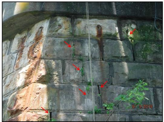
**Photo P5-5:** Vertical cracking on the east face of Pier 5 that extends from the pier cap, at the south edge of the truss beam seat, to the waterline with the crack width increasing to 7/8in wide at the waterline.
