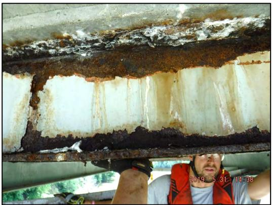
**Photo 113-5:** Section loss of the Stringer 4 web (0.3" thickness remains out of 0.305") and heavy corrosion of both flanges mid-span between FB 2 and FB 3.
