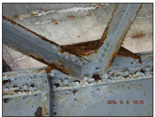
**Photo 850-3:** Typical top flange lateral bracing connection. There is active corrosion with section loss of the plates with pack rust between the lateral bracing members and the plates.
