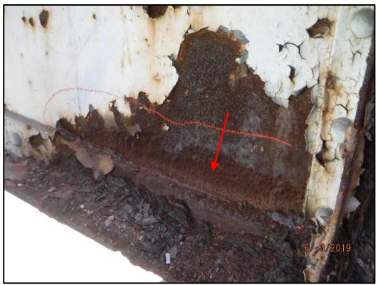
Photo 107-5: Section loss of the Span 4 Girder 1 web just above the bottom flange adjacent Pier 3. Minimum thickness remaining is 0.22" out of 0.5".
