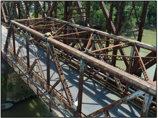
Photo 120-1: Overall condition of the truss with peeling paint and exposed metal throughout.
