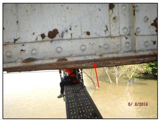
**Photo 107-7:** 1 1/8" of pack rust between the Girder 1 bottom flange cover plate and splice plate in Span 4.
