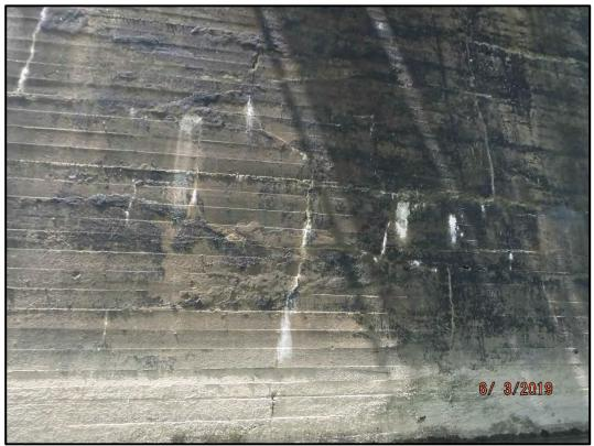
Photo P4-3: Close-up of the cracking with efflorescence on the south end of the Pier 4 east face.
