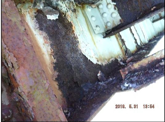
**Photo 152-7:** There is active corrosion with up to 100% section loss on the web and bottom flange of Floorbeam 4. There is 0.4" section remaining of the bottom flange.
