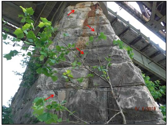
**Photo P5-11:** Vertical cracking on the south west face of Pier 5 that extends from the pier cap to the water line and the vegetation growing in the cracks.
