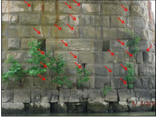
**Photo P5-14:** West face of Pier 5 has 3 full height vertical cracks, one in the middle and then one on each end. Note the vegetation and the heavy cracking of the bottom 3 rows of stones near the water
