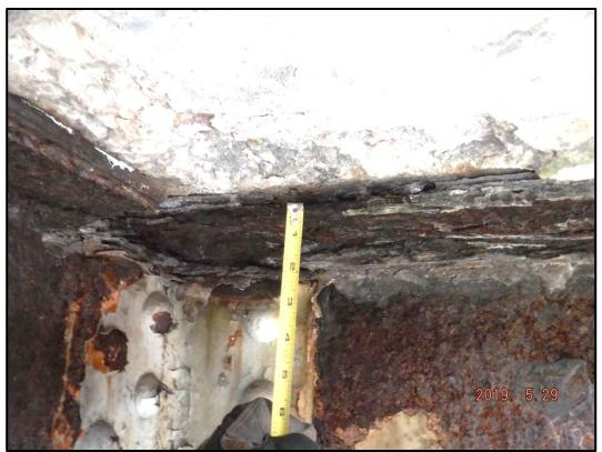
**Photo 152-8:** There is active corrosion with section loss of the top flange and web of Floorbeam 12 adjacent to Stringer 1. There is 0.25" remaining thickness of the top flange and 0.36" remaining thickness of the web.
