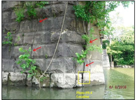
**Photo P5-3:** 3in diameter tree growing from a void in the north east face of Pier 5. Note the vertical crack in the stone under the tree and the vertical crack on the east face that extends from the pier cap to the water line.
