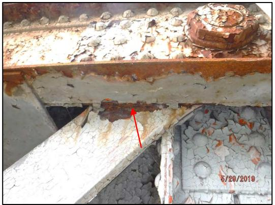
Photo 120-20: Outboard eyebar at panel point U12 on the downstream truss has 1/16" section loss due to fretting corrosion and pack rust between it and the upper chord member.
