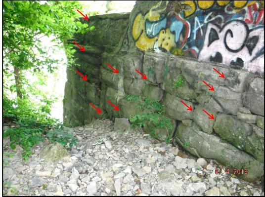
**Photo P6-16:** Cracking on the north end of the Pier 6 west face. Note the heavy efflorescence on the stone and the deterioration of the concrete cap.
