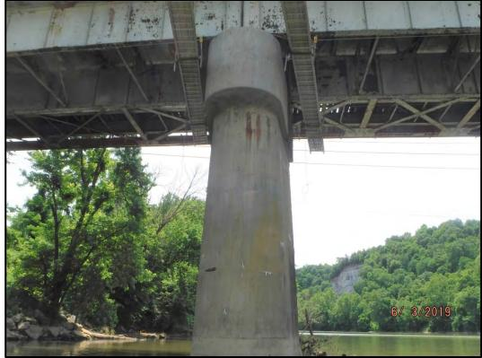
**Photo P4-6:** North face of Pier 4. There is rust staining on the pier wall directly below the pier cap. Note the 1ft wide honeycombing 10ft above the water line along with horizontal and vertical cracking with efflorescence.
