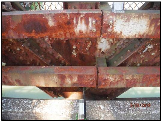
Photo 330-2: Up close view of corrosion on bridge railing. The downstream rail at L8 is shown.
