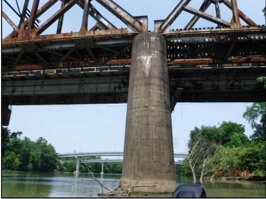
**Photo P4-4:** South face of Pier 4. Note the cracking with heavy efflorescence near the top of the pier and the debris collected on the upstream face of the pier.
