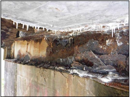
**Photo 152-2:** There is heavy laminar corrosion with up to 100% section loss in the web of the floorbeam at Abutment 1.
