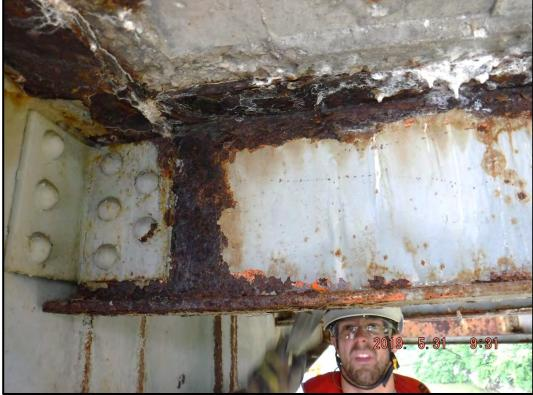
Photo 113-4: Heavy laminar corrosion of Stringer 4 at the connection to the west face of FB 10.
