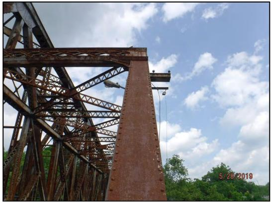
Photo 853-5: Utility line hanger and street light at downstream panel point U2 not functional.
