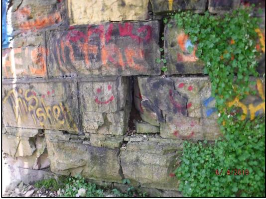
Photo Abt. 7-2: Close-up of the voids on the south end of the Abutment 7 east face.
