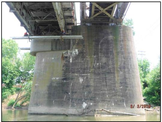
**Photo P4-5:** West face of Pier 4. Note the cracking with rust staining and efflorescence throughout and the debris collecting on the pier.
