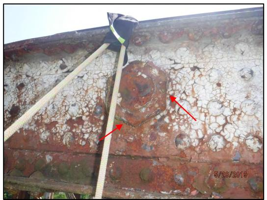
**Photo 120-28:** The washer on the outboard face of the pin at downstream truss panel point U6 has broken and only 50% of the washer is in contact with the pin nut.
