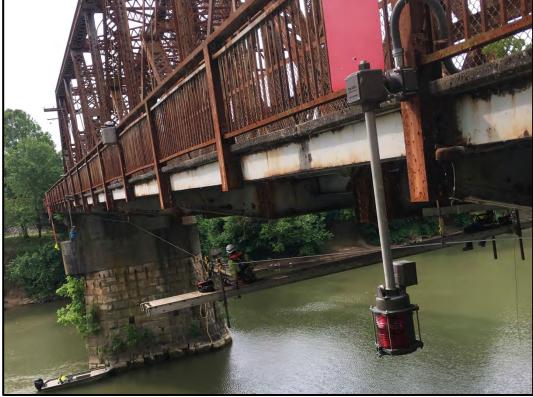
Photo 330-3: Pedestrian bridge railing on downstream side is in fair condition with widespread active corrosion.
