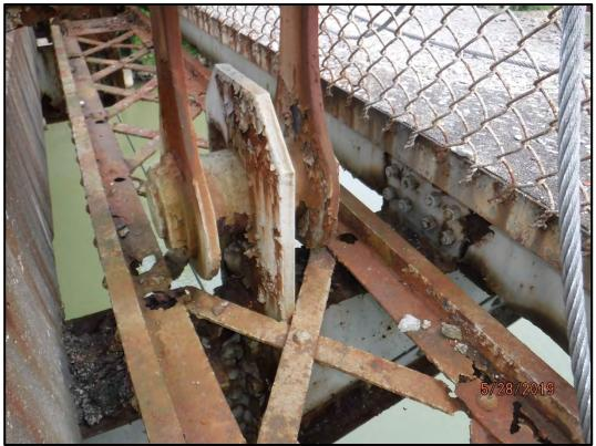
Photo 120-30: Corrosion holes in the lacing bars and connection angles of member L0-L2 on the downstream truss.
