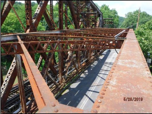
Photo 850-8: Typical active corrosion on the lateral bracing on the top chord of the truss.
