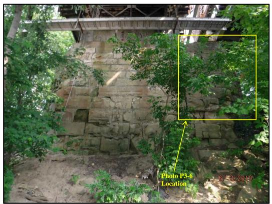
**Photo P3-6:** West face of Pier 3. Note the heavy cracking and deterioration of the bottom 8ft and exterior of the concrete beam seat. The top 10ft directly under the concrete beam seat is in fair condition with minor cracking.
