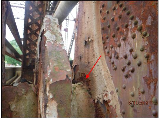
**Photo 120-13:** Active corrosion and pitting on the eyebar head at panel point L7 on the upstream truss. 9/16" out of 3/4" thickness remains.
