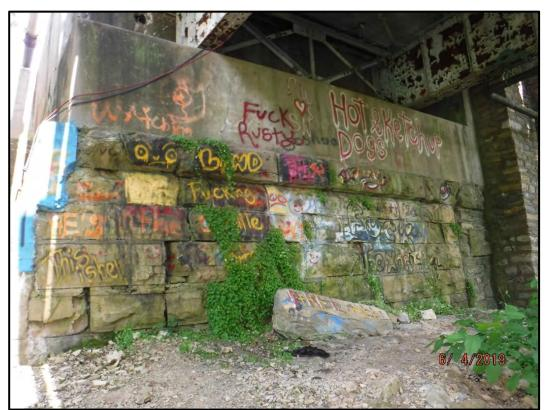
Photo Abt. 7-1: East face of Abutment 7. Note the cracking, mortar deterioration, and voids in the stone.
