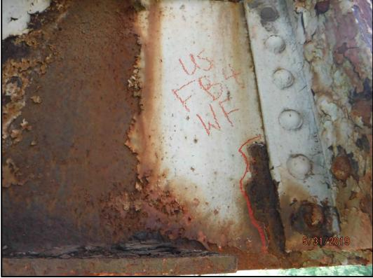
**Photo 152-9:** There is active corrosion with section loss on the upstream end of Floorbeam 8. The section loss measures 8.5"x2" and there is 0.18" thickness remaining.
