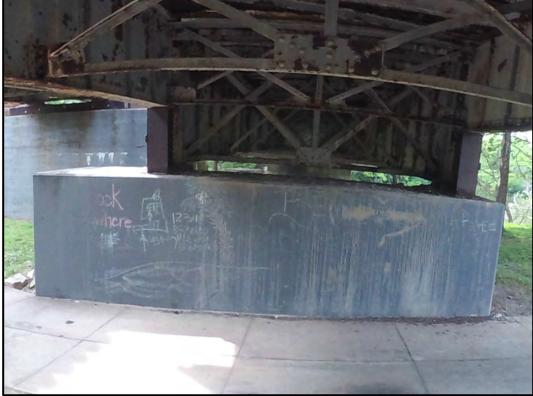
Photo P2-1: East face of Pier 2. Only minor deterioration is present.
