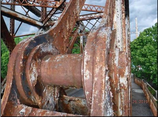
Photo 120-17: Eyebars at panel point M11 on the downstream truss have up to 1/16" deep pitting.
