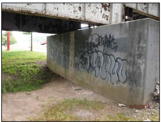
Photo P2-2: West face of Pier 2. Only minor deterioration is present.
