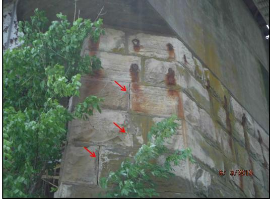
**Photo P5-16:** Vertical cracking on the northwest face of Pier 5 that extends the full height of the pier.
