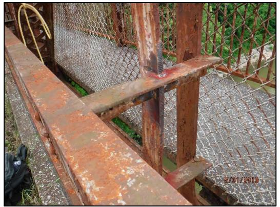
Photo 120-34: Impact damage to the inboard eyebar of downstream truss member L11-M11 after MT was performed. No crack indications were found.
