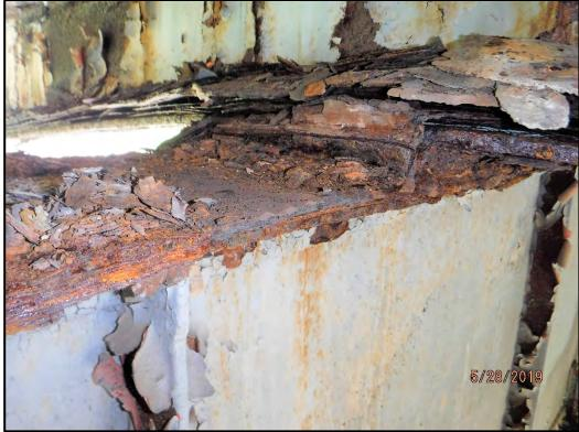
Photo 107-2: Top flange section loss on the Girder 2 at FB 5 in Span 1. 0.32" thickness out of 3/8" remains of the cover plate.
