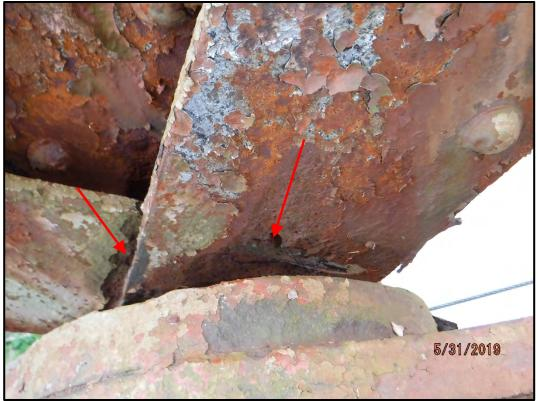
Photo 120-8: 100% section loss on the counter-diagonal pin connection plate at panel point L14 on the downstream truss.
