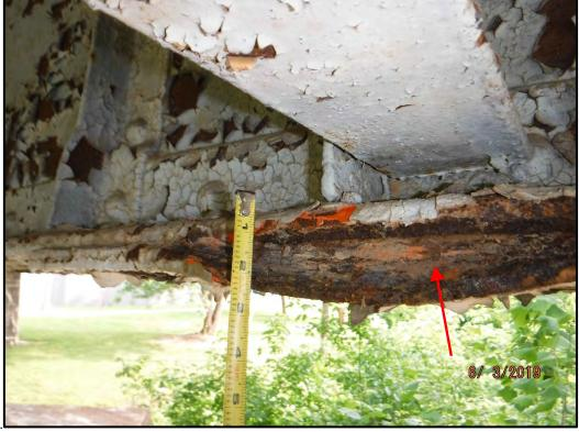
Photo 107-8: 1 <sup>1</sup>/<sub>2</sub>" pack rust between the Girder 1 bottom flange angles and cover plate in Span 3.
