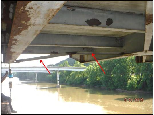
Photo 850-7: Deformation of the lateral bracing between L8 and L7.
