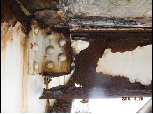
Photo 113-2: Stringer 1 has failed at its connection to the east face of FB 12.
