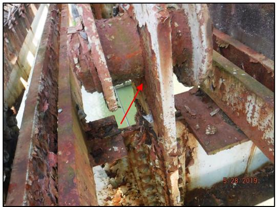
**Photo 161-6:** 3/8" deep pitting of the floorbeam hanger at panel point L7 downstream. The depicted pitting is typical beneath the pins.
