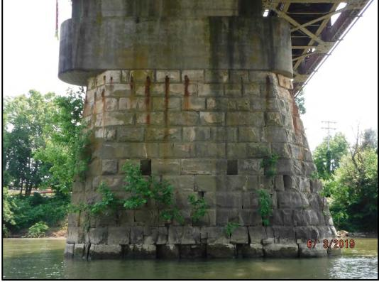
**Photo P5-12:** West face of Pier 5 has rust staining from the top row of stones and 3 full height vertical cracks, one in the middle and then one on each end. Note the vegetation and the heavy cracking of the stones near the water line. The voids near the middle of the pier appear to be from shoring when the superstructure was built.
