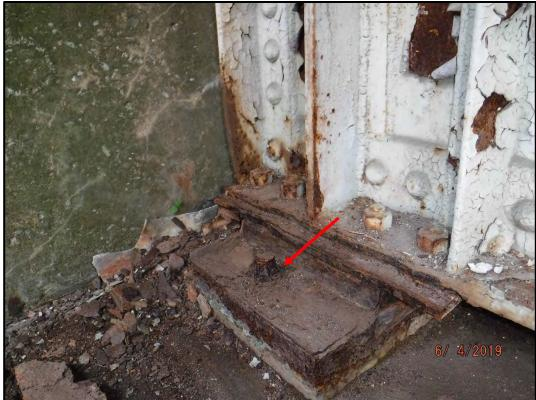
BRG-2: Abutment 7 bearing. There is section loss of the anchor bolt head.
