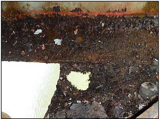
Photo 850-5: Active corrosion with corrosion hole in the lateral bracing gusset plate at the downstream end of Floorbeam 8.
