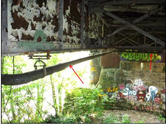
Photo 853-8: Suspected 5" diameter gas line hanging from Girder 2 in Span 6, across the west face of Pier 6, and then along the upstream side of the truss
