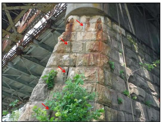
**Photo P5-9:** Rust staining from the top stones on the southeast face of Pier 5. Note the vertical cracking that extends from the pier cap to the water line and the vegetation growing in the cracks.
