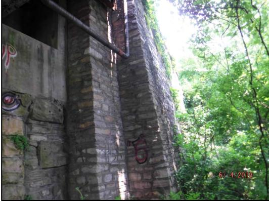
Photo Abt. 7-4: Retaining wall north of Abutment 7 is in good condition.
