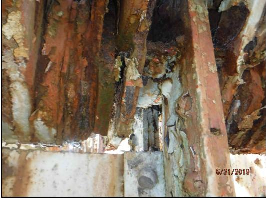
Photo 120-15: Pack rust and section loss on the lower chord pin connection at L8 on the upstream truss.
