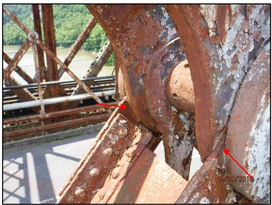
Photo 120-16: Eyebars at panel point M3 on the downstream truss have up to 1/16" deep pitting. Note the 50% section loss of the counter-diagonal pin connection plates.
