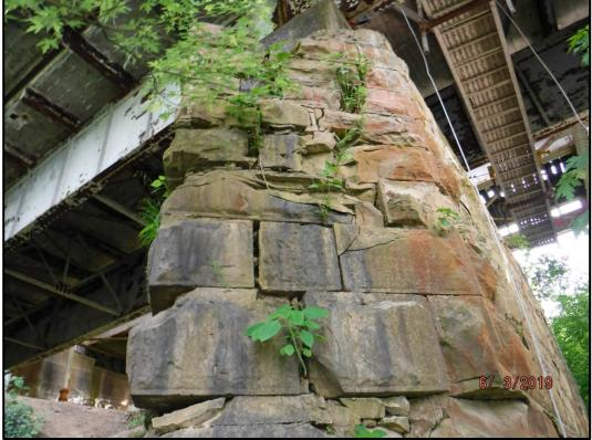
**Photo P3-9:** Northwest face of Pier 3. With heavy cracking and delamination throughout. Note the vegetation growing in the voids.
