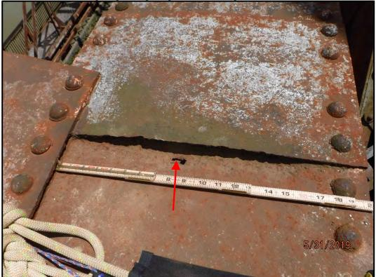
**Photo 120-24:** 7/8" pack rust and 7/16" deep pitting of the upstream U6-U8 upper chord at panel point U6. The pitting is 1 1/2" wide and extends 15" across the top flange plate with a 1" diameter corrosion hole. The nominal plate thickness is 1/2". This is the worst-case upper chord pitting.
