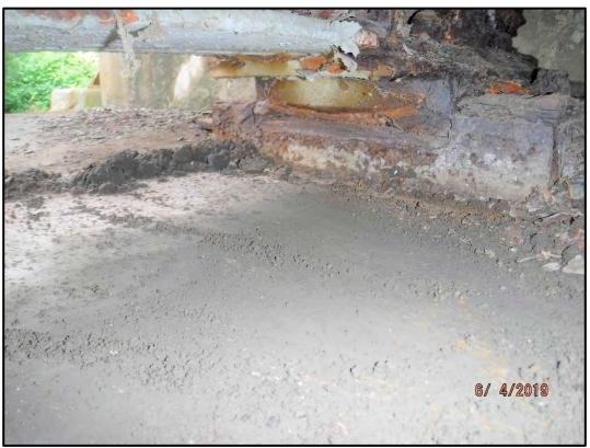
BRG-3: Abutment 7 bearing. There is pack rust on the bearing rocker.
