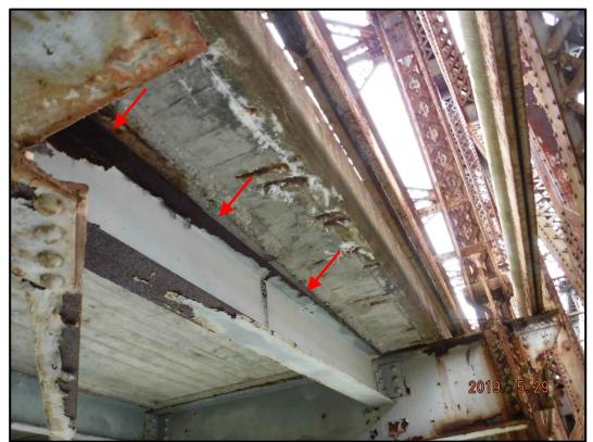
Photo 113-3: Stringer 1 has separated from the deck between FB 11 and FB 12 due to its failure adjacent FB 12. The stringer is only being supported as a cantilever by the connection at FB 11.
