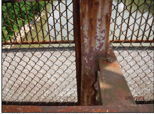
**Photo 120-33:** Impact damage has distorted the inboard eyebar of downstream truss member L11-M11 1 1/2" to the east at the traffic rail welded connection (which is a fatigue-prone detail in and of itself).
