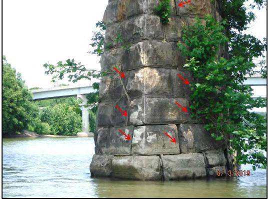
**Photo P5-10:** Vertical cracking on the south face of Pier 5 that extends from the pier cap to the water line and the vegetation growing in the cracks.
