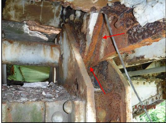
Photo 120-11: 15% section loss of the outboard eyebar head at panel point L16 on the downstream truss. The inboard eyebar is in similar condition.
