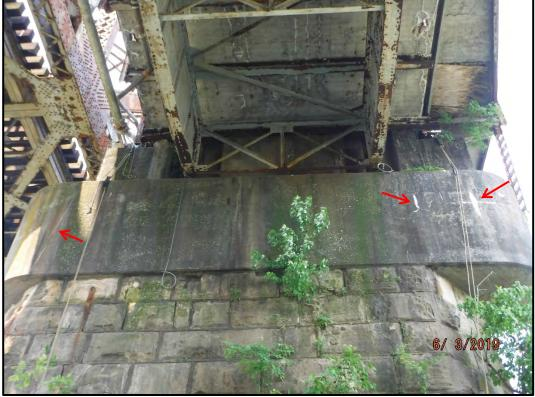
Photo P5-18: Minor cracking with efflorescence on east face of the Pier 4 cap, typical throughout.
