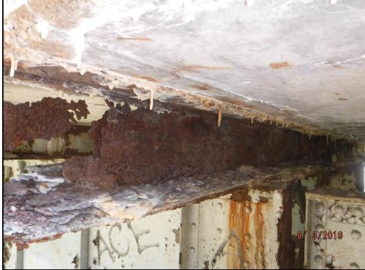
Photo 152-1: Severe section loss and multiple holes in the web of the Span 4 floorbeam at Pier 3. Other floorbeams over the piers have similar section loss.
