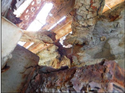
Photo 120-31: Corrosion holes in the lacing bars and connection angles of member L14-L16 on the downstream truss.
