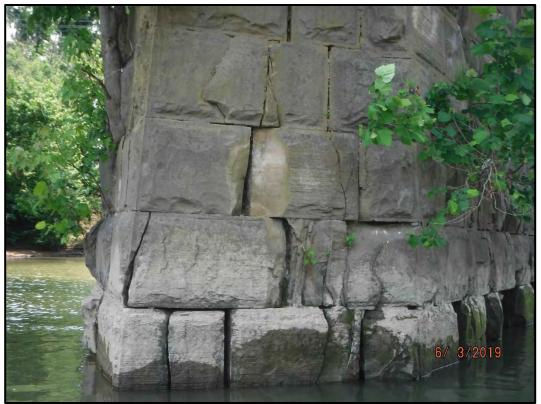
**Photo P5-17:** Heavy vertical cracking and mortar deterioration on the northwest face of Pier 5 at the water line that extends the full height of the pier.
