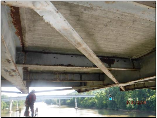
Photo 113-1: Typical active corrosion of the truss stringers.
