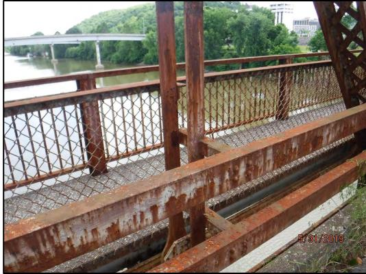
**Photo 330-1:** Typical condition of the downstream metal bridge rail. Active surface corrosion with minor pitting corrosion is typical along both bridge rails for the entire length of the bridge.
