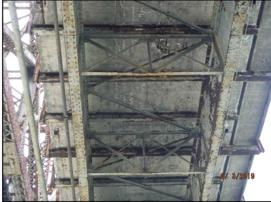
Photo 152-3: Typical active corrosion of the floorbeams. The floorbeams in Span 3 are shown.
