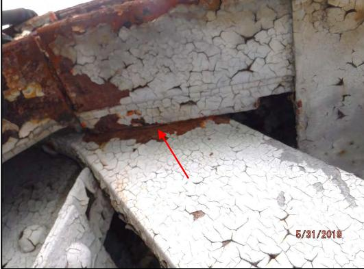
**Photo 120-21:** Outboard eyebar at panel point U14 on the upstream truss has 1/16" section loss due to fretting corrosion and pack rust between it and the upper chord member.
