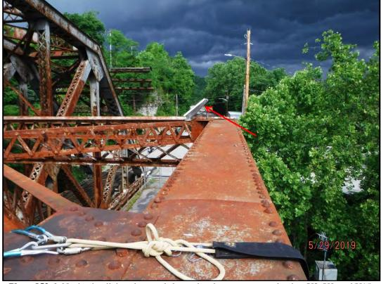
Photo 853-6: Navigation light solar panels located at downstream panel points U2, U8, and U15.
