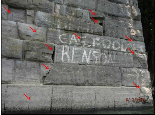
**Photo P6-4:** Minor cracking throughout the north end of the Pier 6 east face. Note the 2 sections of partial missing stones and that the stones at the waterline are encased in concrete. The stones at the waterline have vertical cracks spaced at 2ft.
