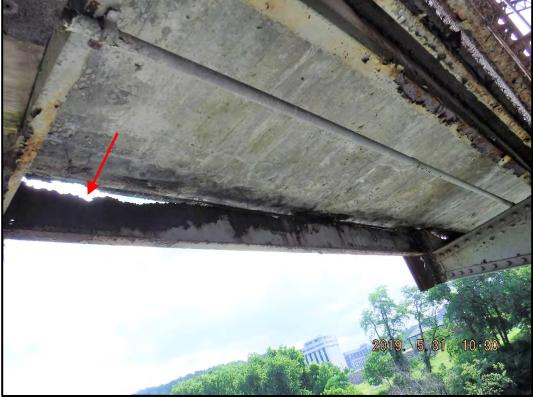
**Photo 113-8:** The sidewalk stringers exhibit 100% section loss in the web and flanges throughout. Many of the stingers are no longer in contact with the concrete sidewalk above.
