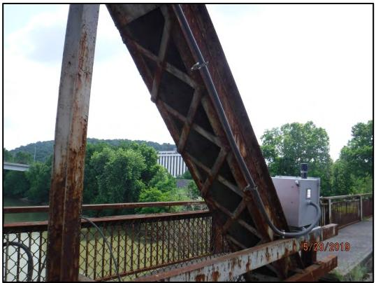
**Photo 853-3:** Navigation light electric service panel at panel point L0 on the downstream truss. The same type of service panel is present at panel point L8 and L16.
