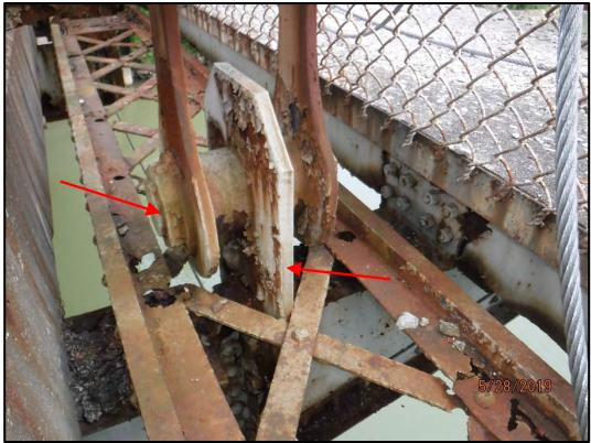
Photo 161-1: Typical truss pin and floorbeam hanger. Panel point L1 on the downstream truss is shown.
