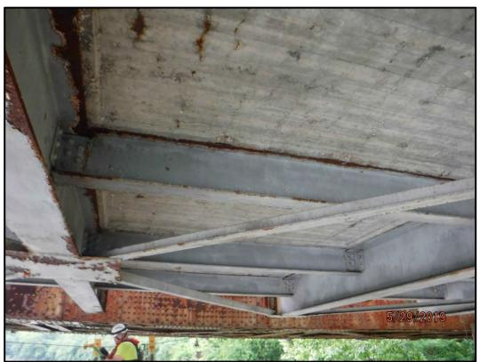
Photo 12-4: Map cracking with rust staining on the underside of the deck between FB 13 and FB 14 of Span 5.
