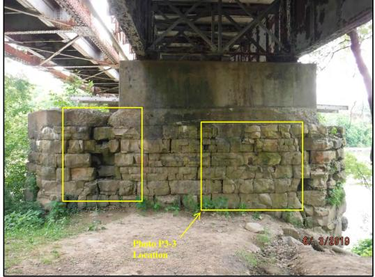
**Photo P3-1:** East face of Pier 3. Note the heavy cracking of the stones throughout and the large 2ft wide x 5ft tall x 2.5ft deep void at the south end of the concrete beam seat.
