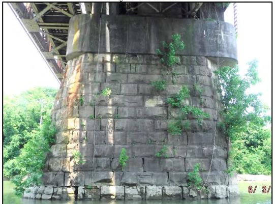
**Photo P5-1:** East face of Pier 5 with vertical cracks extending the full height of the masonry. Note the large amount of vegetation on the pier and the heavy deterioration of the masonry at the water line.
