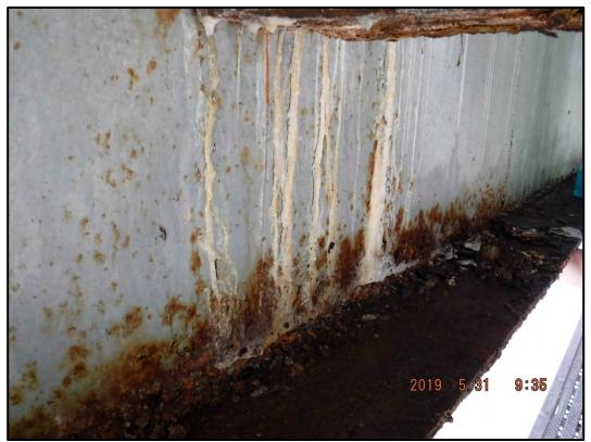
**Photo 152-10:** There is efflorescence and active corrosion on the web and bottom flange of Floorbeam 10 under Stringer 4. There is 0.4" remaining on the bottom flange.
