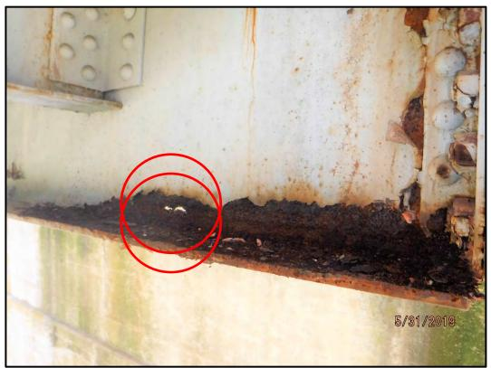
**Photo 152-6:** There is active corrosion with section loss at the bottom of the web of Floorbeam 1. There is a corrosion hole in the web 2.5' from the upstream end of the floorbeam.
