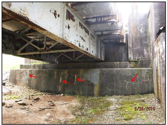
**Photo Abt. 1-1:** Face of Abutment 1. Note full length horizontal cracks with scaling and pop outs throughout the entire face of abutment along with a few vertical cracks with efflorescence.
