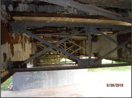
Photo 850-2: Typical lateral bracing in Span 1.
