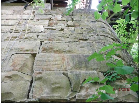
**Photo P3-7:** Close-up of the typical heavy masonry cracking and deterioration of the mortar on the south end of the Pier 3 west face. Note the higher concentration of cracking in the top 8ft that is exterior of the concrete beam seat.
