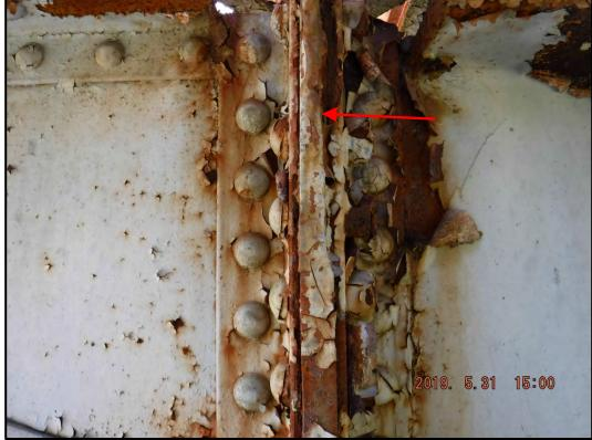
Photo 161-5: Floorbeam hanger at panel point L1 on the downstream truss exhibits worst case section loss with 0.28" remaining out of 1" nominal thickness.
