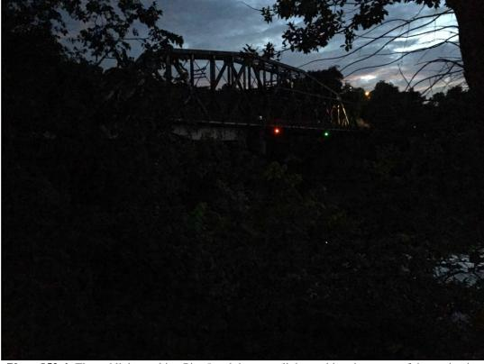
**Photo 853-4:** The red light marking Pier 5 and the green light marking the center of the navigation span are illuminated at dusk. The red light marking Pier 6 is not illuminated.
