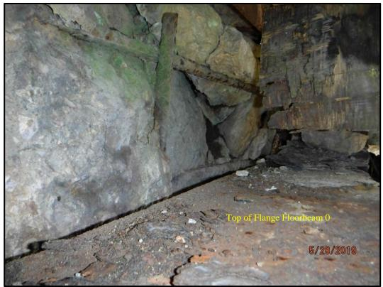
**Photo Abt. 1-3:** Spalling with exposed reinforcement at the top of the Abutment 1 back-wall on the exterior face of Girder 2.
