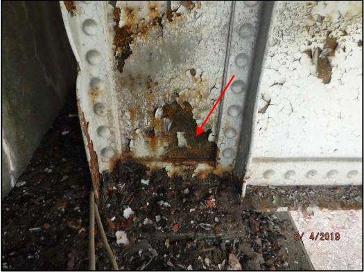
Photo 107-6: 0.11" deep pitting of the Span 6 Girder 1 web at Pier 6.
