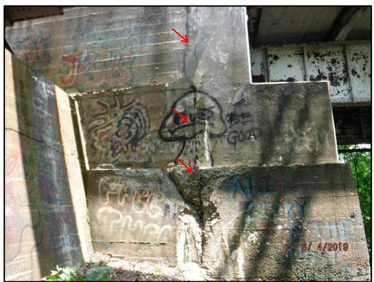
Photo Abt. 7-3: Vertical crack and large 4in deep spall on the south face of Abutment 7 where the backwall meets the wing wall.
