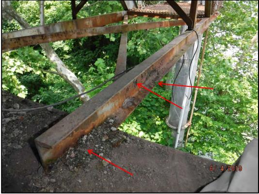
**Photo 853-2:** Channels supporting the USGS station have pack rust and laminating corrosion at their bearings on Pier 6, and there are corrosion holes in the webs and bottom flanges.
