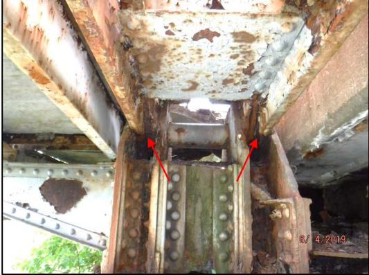
Photo 120-9: 10% section loss of the eyebar heads at panel point L0 on the downstream truss.
