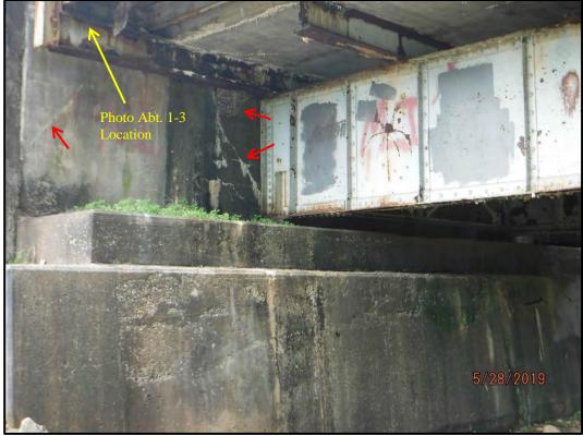
Photo Abt. 1-2: Cracking with heavy efflorescence and spalling in the Abutment 1 backwall behind Girder 2. Note the scaling on the face of the abutment.
