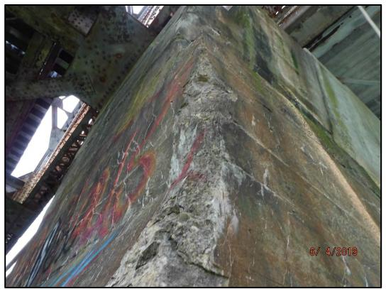
**Photo P6-11:** Spalling and deterioration on the south east corner of the Pier 6 concrete cap. Note the map cracking with efflorescence throughout. The north east corner of the concrete cap is similar.
