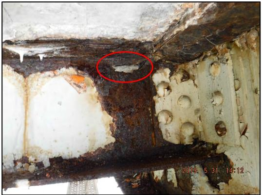
**Photo 113-7:** 6" x 4" hole in the Stringer 4 web at the west face of FB 4. A similar condition also exists on Stringer 4 west of FB 6.
