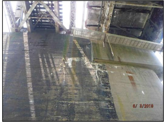
**Photo P4-2:** Close-up of the cracking with heavy efflorescence on the east face of Pier 4 under the pier cap. Notice the horizontal cracking is consistent with the masonry joints that are encased in concrete.
