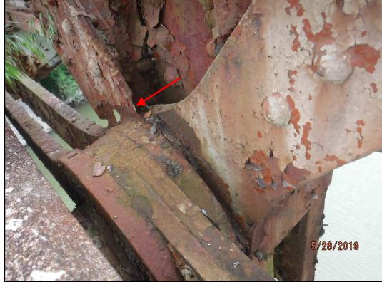
**Photo 120-4:** 100% section loss of the counter-diagonal pin connection plate at panel point L6 on the downstream truss.
