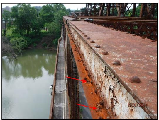
**Photo 120-26:** Typical 1/8" deep pitting that is collecting debris on the upper chord bottom flange angle. Picture is of the downstream truss between panel points U10 and U12.
