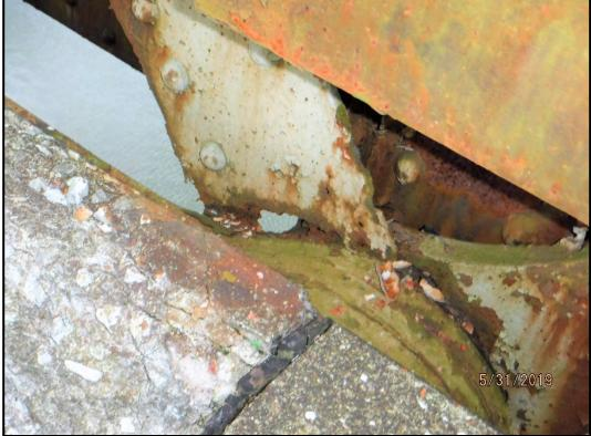
Photo 120-7: 100% section loss on the counter-diagonal pin connection plate at panel point L12 on the upstream truss.
