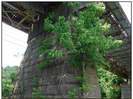
**Photo 859-1:** 3" diameter tree and other vegetation growing in the mortar joints on Pier 5. This is the worst case of the substructures.
