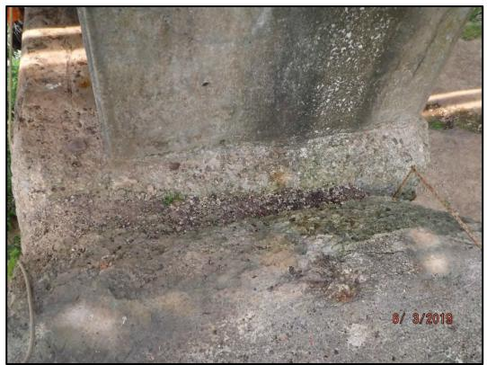
**Photo P3-2:** A drainage issue has caused heavy deterioration on the south end of the Pier 3 cap adjacent to the beam seat. This deterioration has formed a ditch in the cap that is 30in wide by 18in deep at the east edge of the cap.
