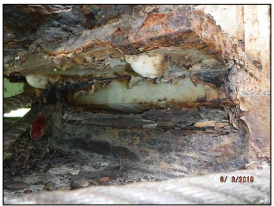
BRG-4: Span 3 bearing at Pier 3. There is pack rust on the bearing rocker.
