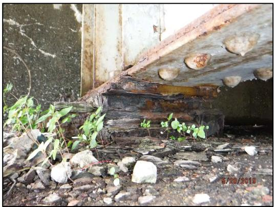
**BRG-1:** Abutment 1 bearing. There is pack rust on the bearing rocker.
