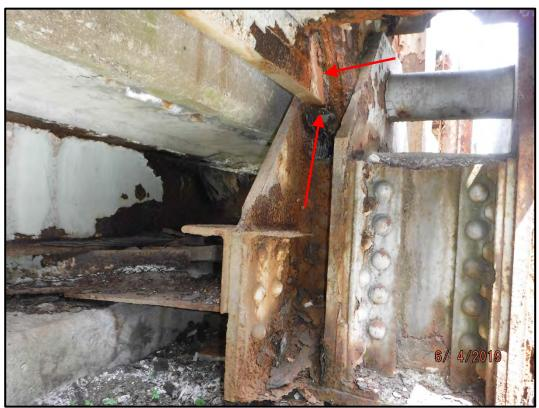
Photo 120-10: 10% section loss of the inboard eyebar head at panel point L0 on the upstream truss. The outboard eyebar is in similar condition.
