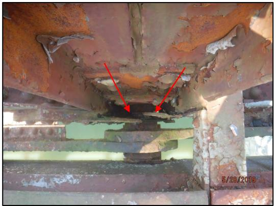
Photo 161-4: Pin at panel point L2 of the downstream truss has 1" of section loss. 4" diameter remains out of a 5" nominal diameter.
