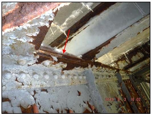
**Photo 107-3:** Typical pack rust causing deformation of the top flange cover plate. Girder 2 in Span 3 is shown.
