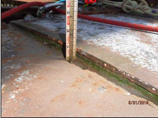
**Photo 120-23:** Typical 9/16" pack rust and 1/4" pitting of the upper chord along the top flange splice plate at panel point U8 on the upstream truss.
