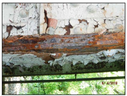
**Photo 107-9:** Section loss of the Girder 1 bottom flange in Span 6. 0.35" out of 3/8" splice plate thickness remains, 0.46" out of 9/16" cover plate thickness remains, and 0.47" out of 5/8" double angle thickness remains. (Girder 2 is similar)
