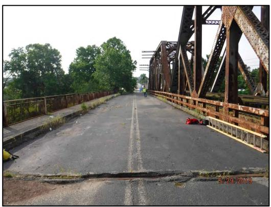
Photo 12-2: 6" long x 3" vertical x full width transition between Spans 4 and 5.
