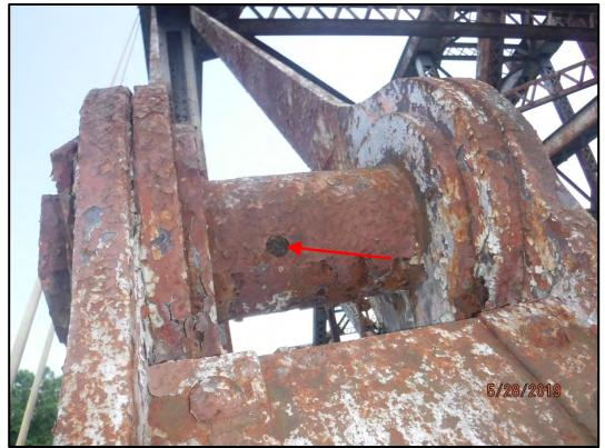
Photo 161-2: Typical mid-height panel point pin and collar. Note the hole in the collar that appears to have been drilled, perhaps to measure the collar thickness and pin diameter.
