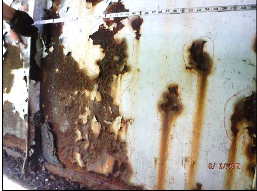
**Photo 107-4:** Section loss in the Span 4 Girder 1 web at Pier 3. Minimum thickness remaining is 0.185" out of 0.5".
