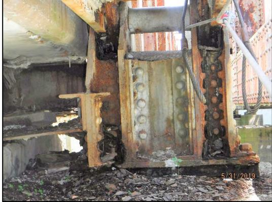
**BRG-5:** Bearing of the upstream truss. There is active corrosion with section loss of the rivet heads and pitting on the bearing plates.
