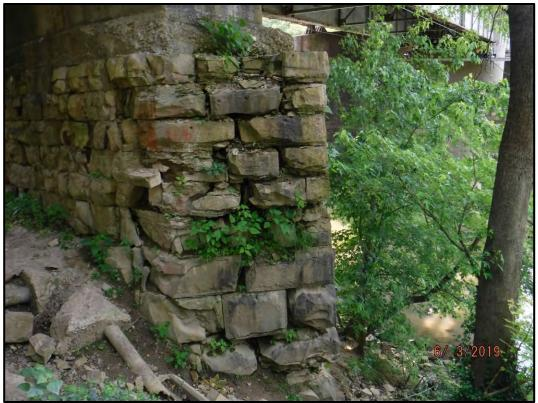
**Photo P3-4:** Northeast face of Pier 3. Note the heavy cracking and voids that are 3in wide and up to 2.5ft deep.
