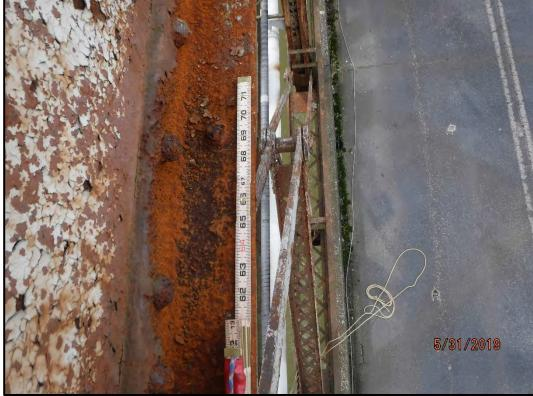
**Photo 120-27:** 7/16" deep pitting of the upstream truss upper chord member U2-U4 bottom flange angle located 4 feet from panel point U2. The nominal angle thickness is 5/8".
