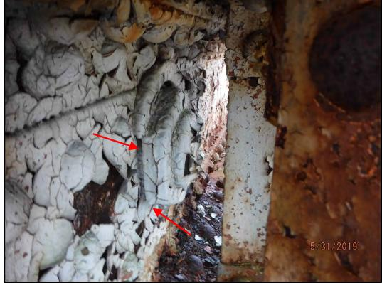
**Photo 120-29:** The washer on the inboard face of the downstream pin at U10 has broken and only 20% of the washer is in contact with the pin nut.
