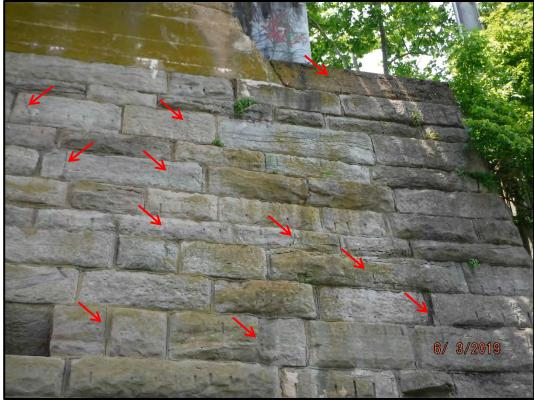
Photo P6-2: Minor cracking throughout the north end of the Pier 6 east face.
