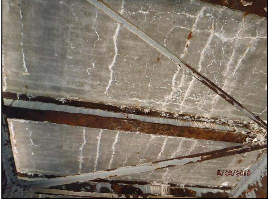
Photo 12-3: Heavy map cracking with efflorescence on the underside of the deck in Span 1.
