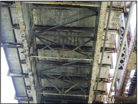
Photo 850-1: Typical underside of Span 4 showing lateral bracing and steel diaphragm. Moderate corrosion is apparent on the lateral bracing.
