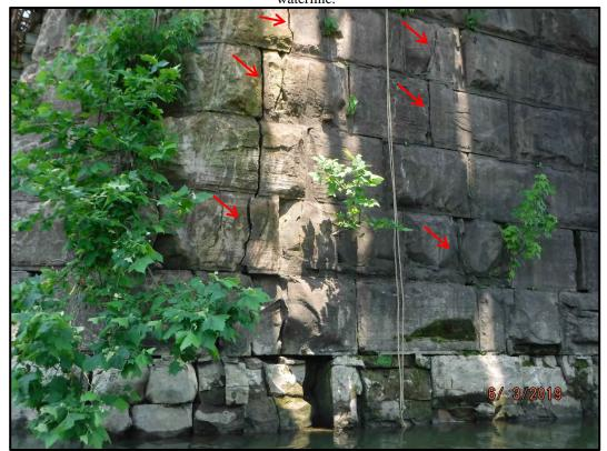
**Photo P5-7:** Vertical crack on the east face of Pier 5 that extends from the pier cap, at the south edge of the truss beam seat, to the waterline with the crack width increasing to 7/8in wide at the waterline. Note the typical heavy cracking of the stone at the waterline.
