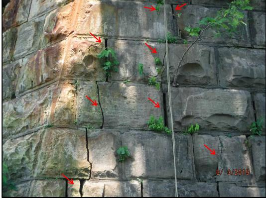
**Photo P5-6:** Vertical cracking on the east face of Pier 5 that extends from the pier cap, at the south edge of the truss beam seat, to the waterline with the crack width increasing to 7/8in wide at the waterline.
