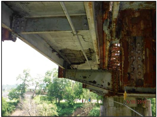
Photo 12-6: Heavy spalling with exposed reinforcement on the underside of the sidewalk in Span 5. The poor condition of the sidewalk concrete is a risk to the public beneath the bridge due to falling of spalled concrete.
