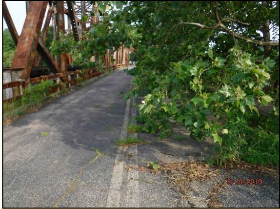
**Photo 859-2:** Vegetation is growing the full length of the bridge in both gutter lines. There is also a large tree overgrowing across the deck near Pier 3.
