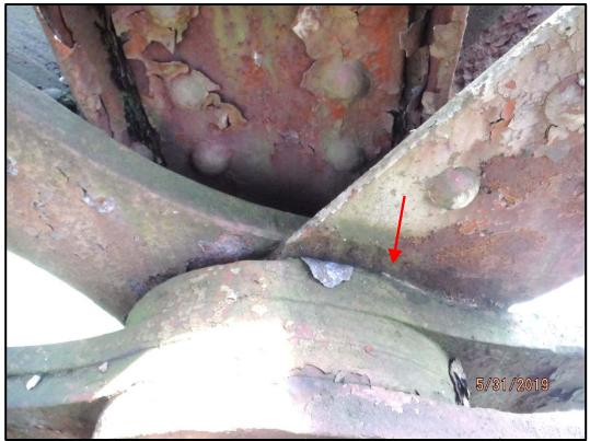
**Photo 120-6:** 1/16" out of 1/2" thickness remains on the counter-diagonal pin connection plate at panel point L10 on the downstream truss.
