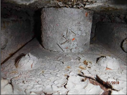
Photo 161-3: Typical upper chord pin and collar. Note there is less corrosion than the mid-height and lower chord panel points.
