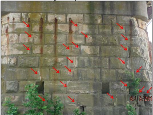
**Photo P5-13:** West face of Pier 5 has rust staining from the top row of stones and 3 full height vertical cracks, one in the middle and then one on each end.
