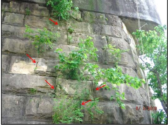
**Photo P5-2:** Vertical cracking on the east face of Pier 5 under Girder 2 that extends from the pier cap to the water line. Note how the cracks get wider as they extend downward and the amount of vegetation on the pier.
