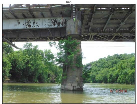
**Photo P5-15:** North face of Pier 5. Note the 3in diameter tree growing from the pier and the large cracks near the water line.
