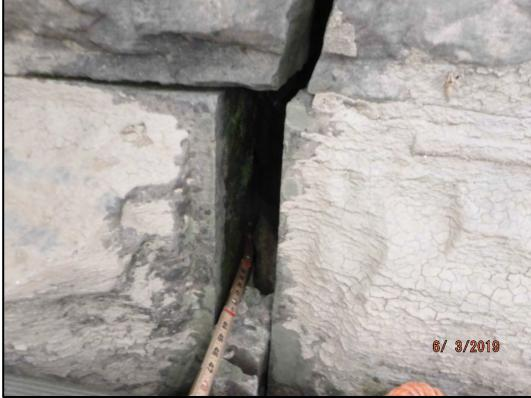
Photo P5-4: A 3in wide by 43in deep void between stones at the water line on the north east face of Pier 5 under the 3in diameter tree.
