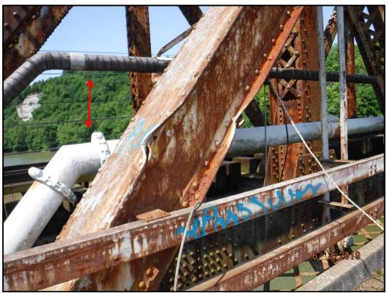
Photo 853-7: Suspected gas lines hanging from the upstream side of the truss. Pipe diameters are 5" and 8.5".
