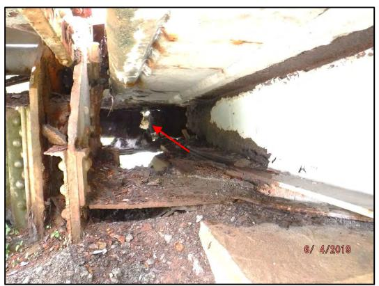
Photo 152-4: Floorbeam 0 in the truss span is severely deteriorated with failure imminent.
