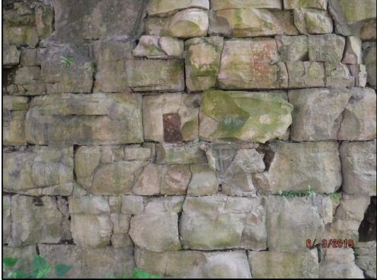
Photo P3-3: Close-up of the typical masonry cracking and heavy deterioration of the mortar on the north end of the Pier 3 east face.
