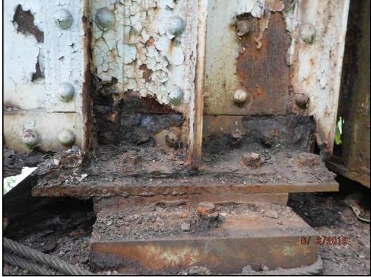
BRG-4: Span 3 bearing at Pier 3. There is section loss of the anchor bolt head.
