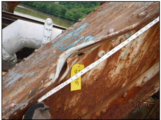
**Photo 120-32:** Impact damage to member L0-U2 on the upstream truss just above the traffic rail. One rivet is severed and there is a tear in the top flange plate connection angle.
