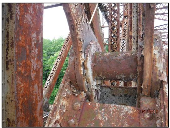
Photo 120-18: Eyebars at panel point M5 on the upstream truss have up to 1/16" deep pitting.
