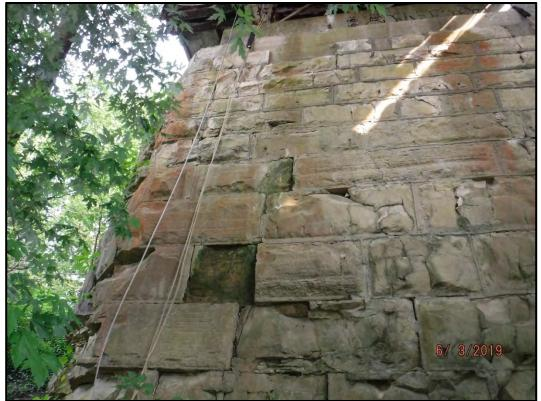
**Photo P3-8:** Minor to moderate cracking and delamination on the north end of the Pier 3 west face. Note the higher concentration of cracking exterior of the concrete beam seat.
