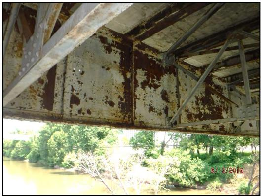
Photo 107-1: Typical condition of the protective coating on the steel girders. The inside face of Girder 2 in Span 3 is shown.
