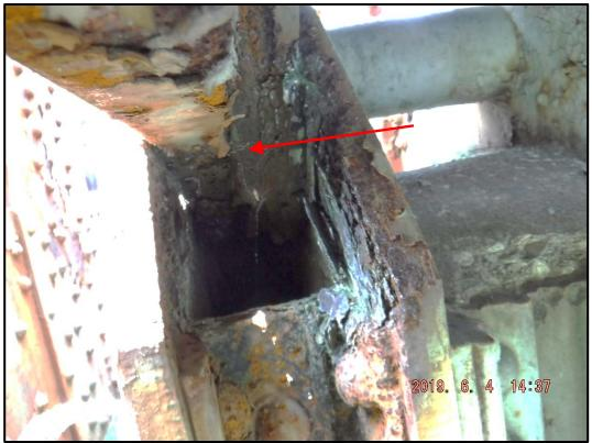
**Photo 120-12:** 15% section loss of the outboard eyebar head at panel point L16 on the upstream truss. The inboard eyebar is in similar condition.
