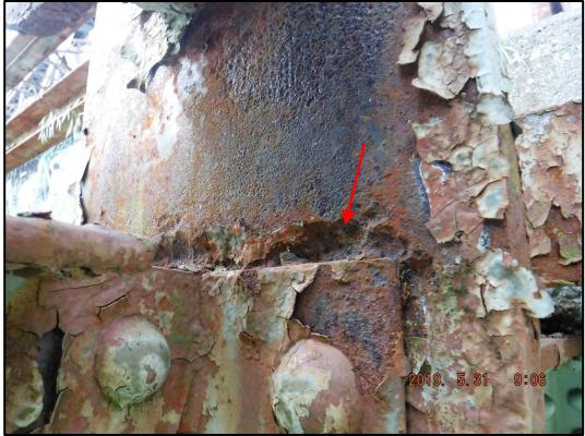
**Photo 161-7:** 5/16" deep pitting of the floorbeam hanger at panel point L11 downstream. The depicted pitting is typical along the top of the floorbeam connection angles.
