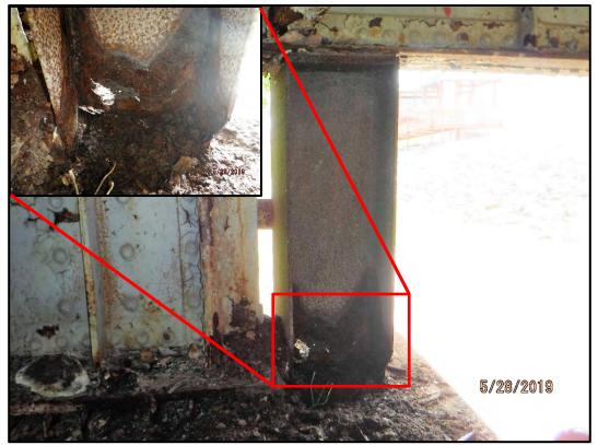
**BRG-7:** Typical stub column at Pier 2 under Girder 2 of Span 1. There is active corrosion and section loss up to 100% at the base of the column.
