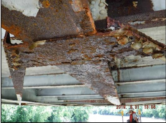
Photo 850-6: Active corrosion on the lateral bracing connection on the downstream end of Floorbeam 4.
