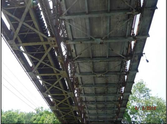
Photo 850-4: Typical underside of Span 5 looking east showing lower lateral bracing in the truss spans.
