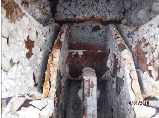
Photo 120-19: No measurable section loss of eyebar members and plates inside the upper chord at panel point U2 on the upstream truss.
