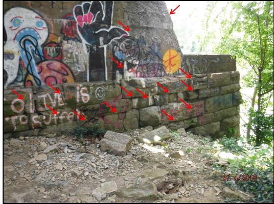
**Photo P6-14:** West face of Pier 6. Moderate cracking on the south end with delamination of the stone face around the cracks. Note the heavy deterioration of the pier cap concrete and heavy efflorescence, where the outer cement layer is flaking off.
