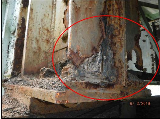
**Photo 107-10:** Active corrosion with 100% section loss of the bottom 6" of the Girder 1 end bearing stiffeners over Pier 3.
