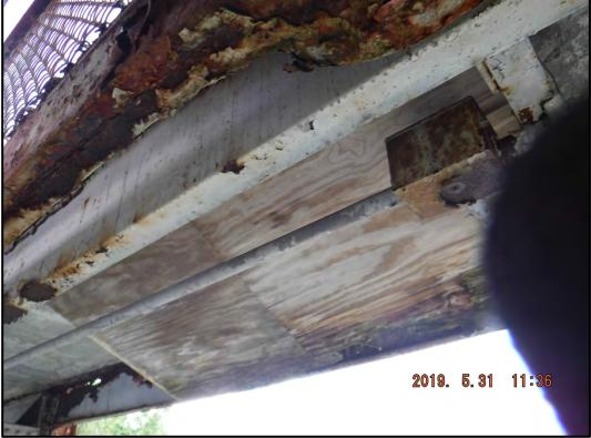
**Photo 12-7:** Plywood protection for spalling concrete under the sidewalk that has become a hazard to boat traffic underneath; the location is around mid-span of span 5 near the blue navigation light.
