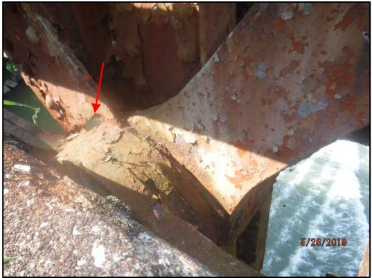
**Photo 120-3:** 100% section loss of the counter-diagonal pin connection plate at panel point L4 on the downstream truss.
