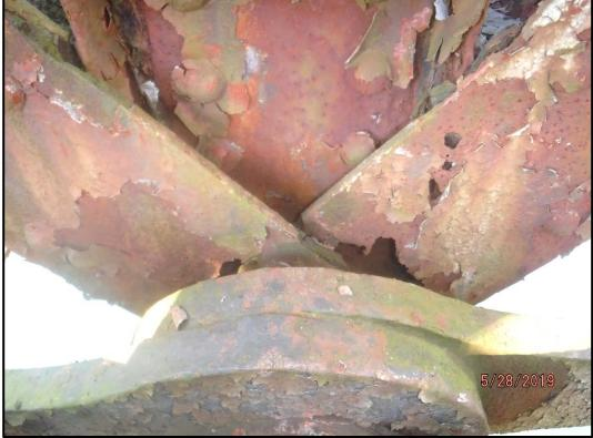
**Photo 120-2:** 100% section loss of the counter-diagonal pin connection plates at panel point L2 on the downstream truss.
