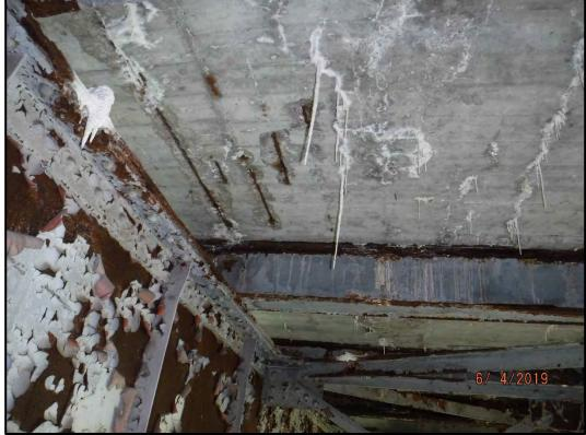
Photo 12-5: Heavy map cracking with efflorescence and exposed rebar on the underside of the deck in Span 6.
