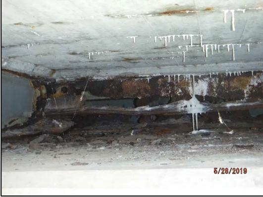
Photo 152-5: Floorbeam 16 of the truss span is severely deteriorated with failure imminent.
