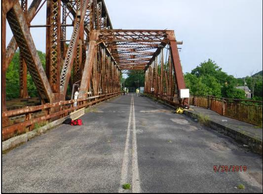
Photo 12-1: Typical cracking and rutting of the asphalt wearing surface with vegetation growth.
