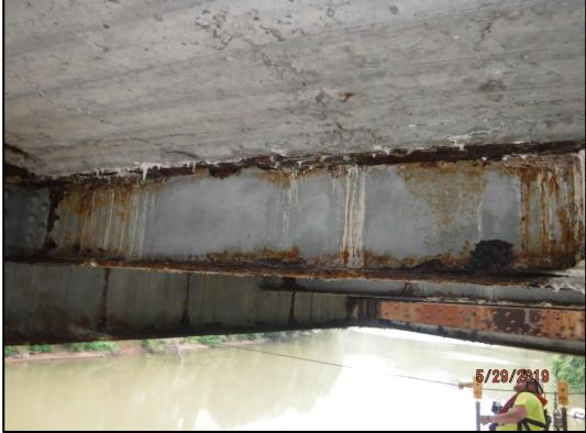
**Photo 113-6:** Minor corrosion of the Stringer 3 web and section loss of the bottom flange (0.45" thickness remains out of 0.54") between FB 12 and FB 13.
