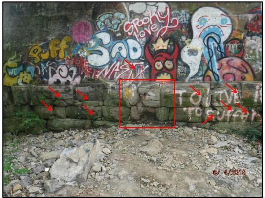
**Photo P6-15:** Heavy cracking of the stones at the centerline of Pier 6 on the west face. Note the moderate cracking throughout the remaining stones and the graffiti on the concrete face.
