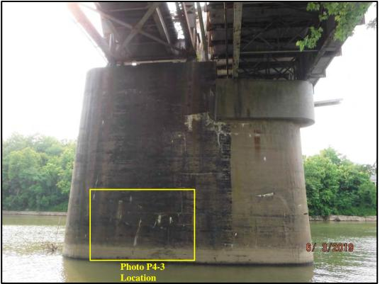
Photo P4-1: East face of Pier 4 has horizontal and vertical cracking with efflorescence throughout.
