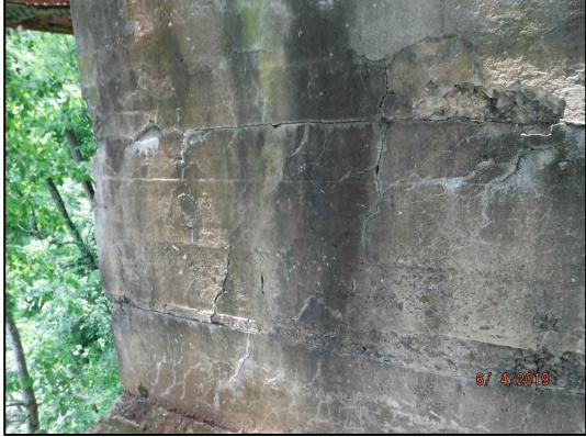
**Photo P6-10:** 6ft by 6ft area on the south end of the Pier 6 concrete cap east face has heavy map cracking with efflorescence and is delaminated.
