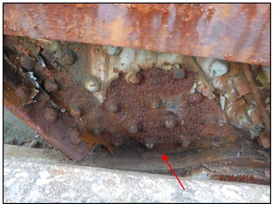
**Photo 120-22:** Pitting of the  $\frac{3}{4}$ " stiffening plate on the inboard face of downstream truss member L0-U2 at panel point L0. Note the 50% section loss of the rivet heads directly above the eye bar.
