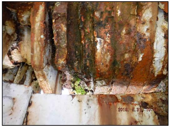
Photo 120-14: Pack rust and section loss on the lower chord pin connection at L8 on the downstream truss.
