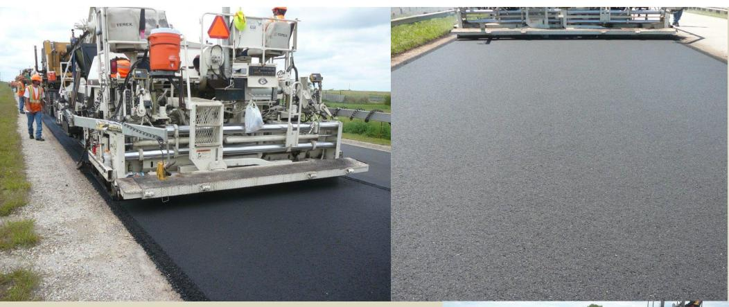
The recycled asphalt mix is then placed with the paver with a vibratory screed and then compacted.
