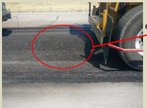
The material is windrowed to expose the next lift of material for heating.
