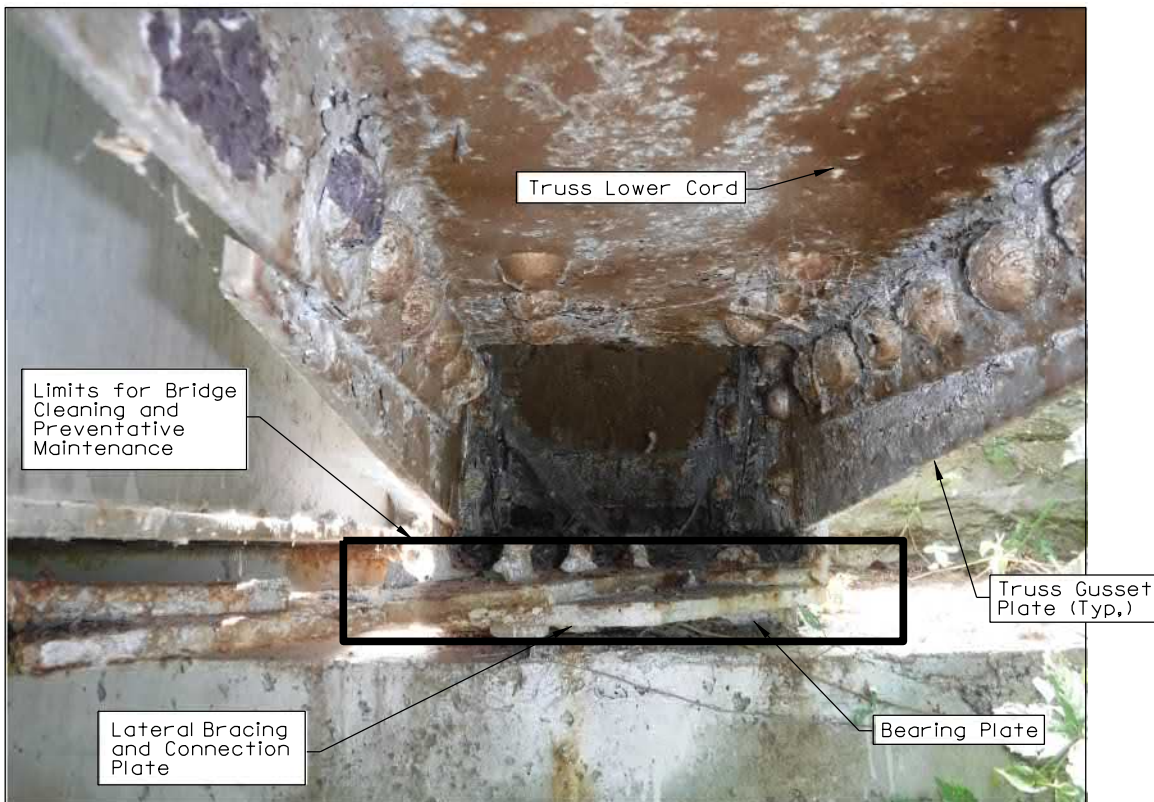
Photo 2 - Cross section view of typical bearing at abutment
