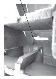
Broken Weld Between Grid and Top Flange of FBI in Southbound Lane
