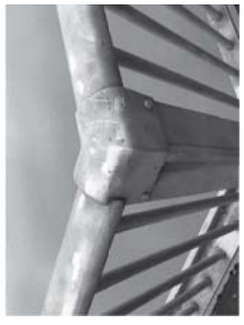
HANDRAIL SPLICE REPLACEMENT AT UPSTREAM FB22'
