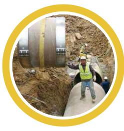
**Note:** When using mechanical joints, torque bolts to the minimum needed for sealing - maximum 25 ft-lbs.
