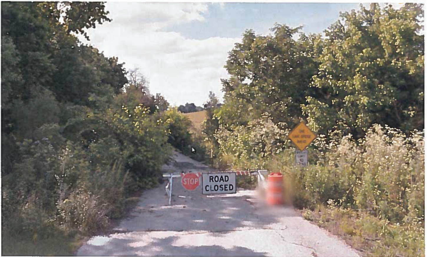
Closed bridge over Hays Fork.
