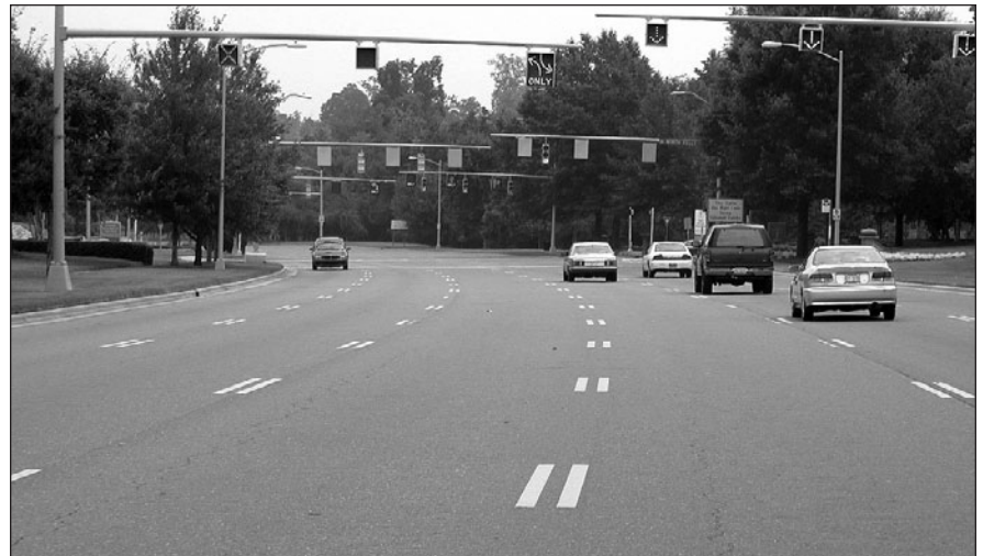
Figure 2. Overhead lane signals on Tyvola Road in Charlotte, NC.
