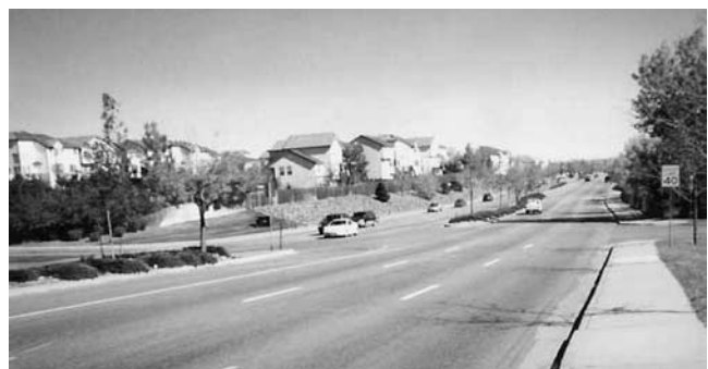
Figure 17. Conventional median opening at four-leg intersection.
