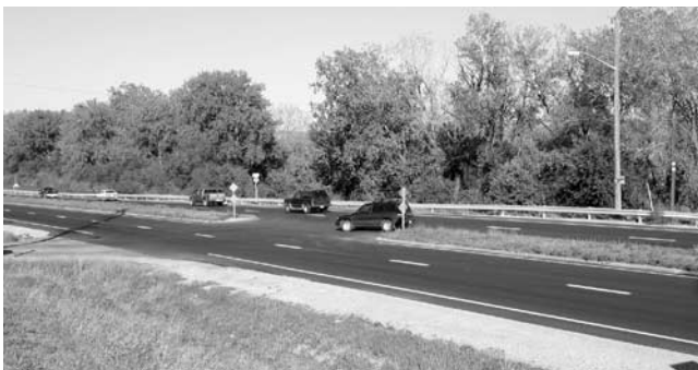
Figure 15. Conventional median opening at three-leg intersection.
