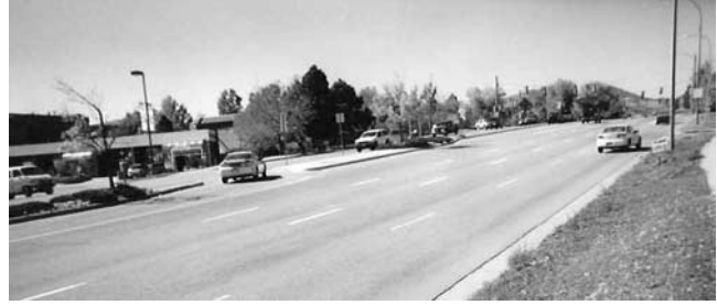
Figure 16. Directional median opening at three-leg intersection.
