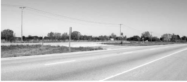
Figure 14. Conventional midblock median opening.
