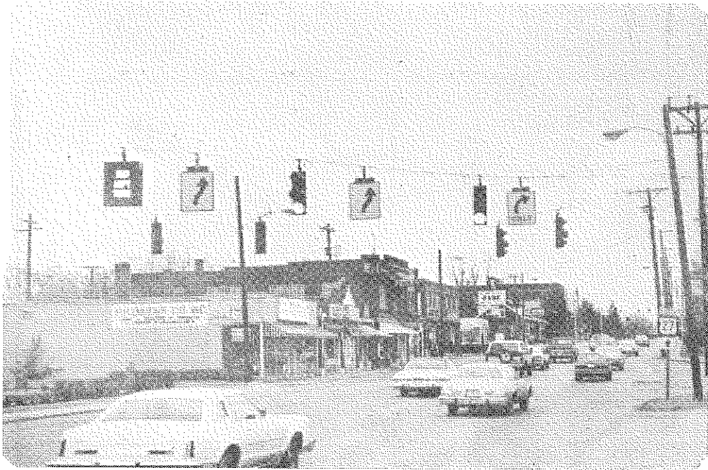
Figure 14a. Signing Added to North End of Reversible-Lane Section; Sign in AM Peak Position.
