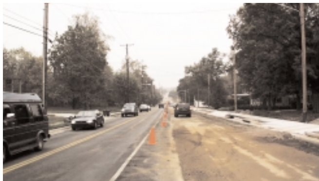
U.S. 27 Widening - Expanding roadway capacity
