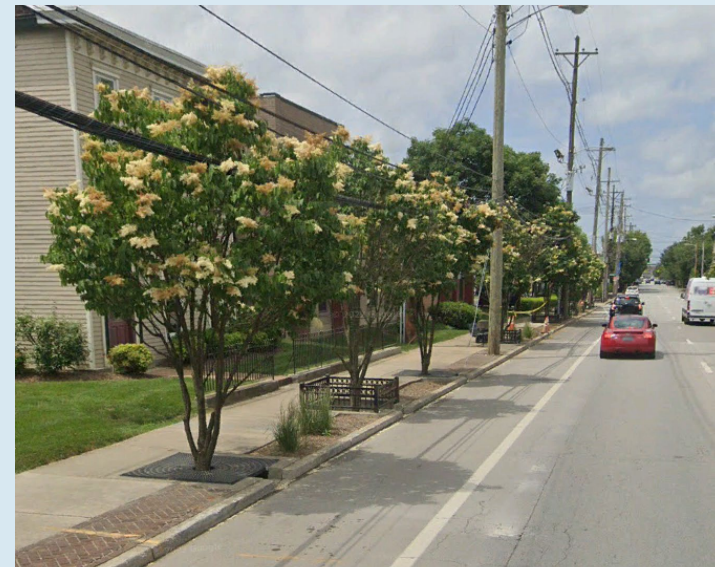
Figure 19: Green Sidewalk Infrastructure along US 60 (Story Ave) in Louisville
