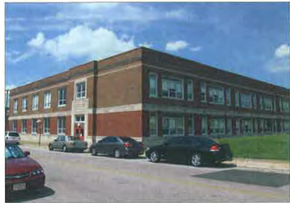
Jeffersonville High School Gymnasium Wing at 601 E. Court Avenue
