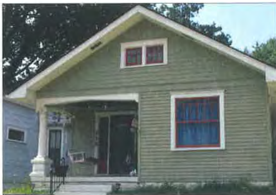
Residence at 713 E. Seventh Street
