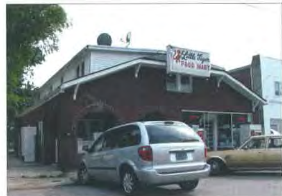
Commercial Building at 228 Stansifer Avenue
