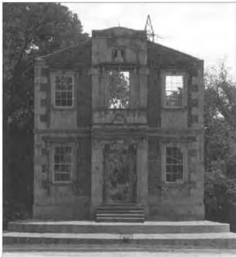
Heigold House Façade at Frankfort Avenue and River Road
