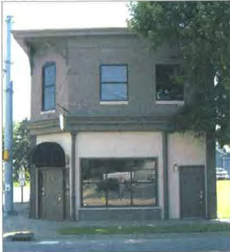
Commercial Building at 428 Vincennes Street
