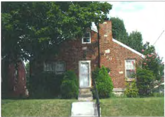
120 North Randolph Street
