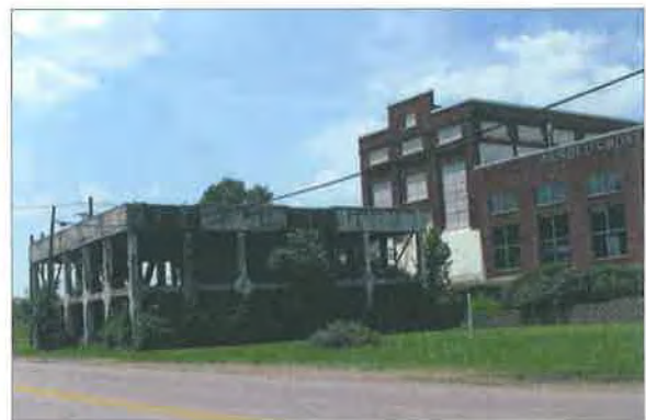
Industrial Complex at 2035–2039 River Road
