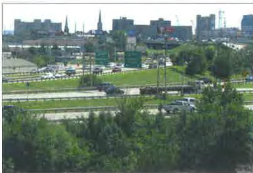
Kennedy Interchange in Downtown Louisville
