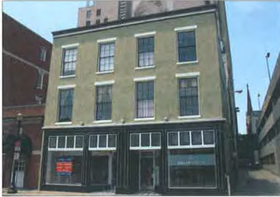
Commercial Building at 438 S. Third Street
