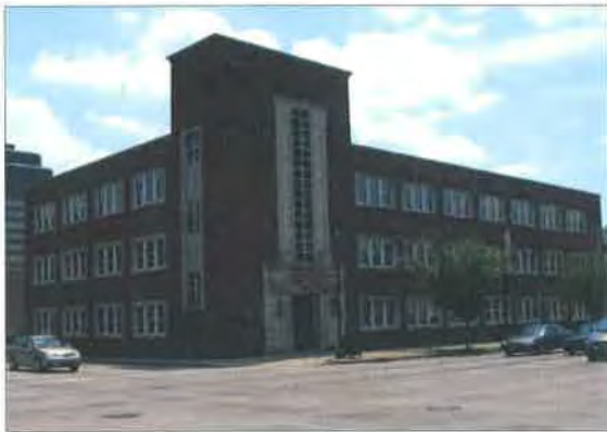
Office Building at 501 S. Second Street
