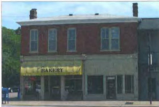
Commercial Building at 332-334 E. Court Avenue
