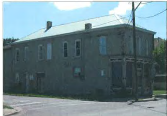
Commercial Building at 624 Vincennes Street
