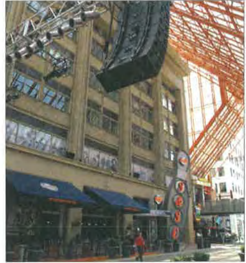
Kaufman-Strauss Building by Local Architect Mason Maury
