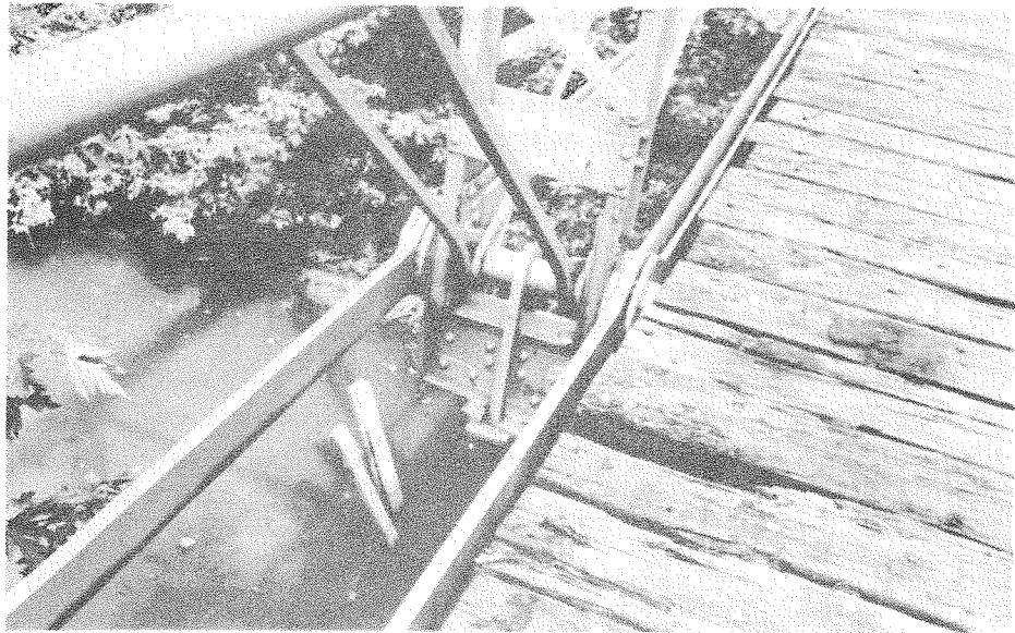
Metal truss bridge with pin-connected bottom chord panel point. (SF #18)
