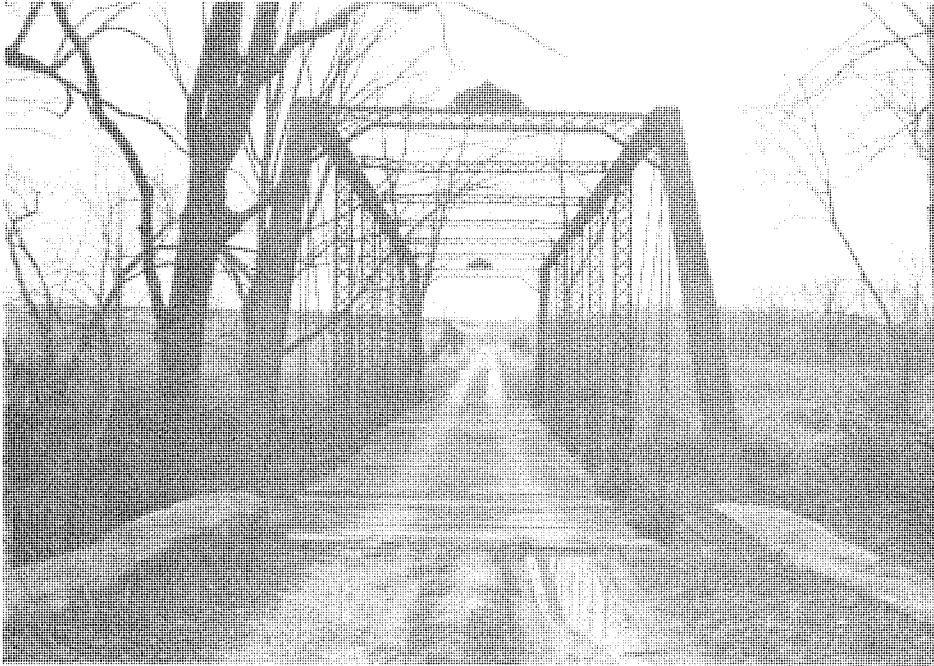
1886 Pratt through truss by the King Bridge Company of Cleveland, Ohio. This little used bridge in Breckinridge County has the familiar builder/date plate and delicate portal bracing found on most King trusses. (SF #13).
