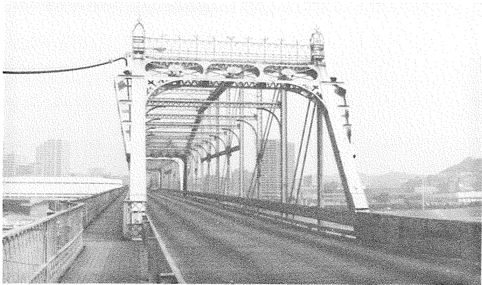
Portal view of elaborate finials and decorative work on the portal strut of the Central Bridge between Newport, Kentucky, and Cincinnati, Ohio. (SF #30)
