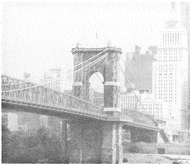
View of Cincinnati and north tower of the Covington-Cincinnati Suspension Bridge over the Ohio River. Stone for the towers was quarried in Portsmouth by the Buena Vista Stone Company and floated downstream to the erection site. (SF #34)
