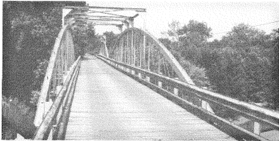
Roadway view of two spans of the three span 423 foot bowstring arch bridge over Barren River near Bowling Green. This bridge was built by the King Iron Bridge and Manufacturing Company of Cleveland, Ohio. The three panel bracing truss outside the arch is probably a later addition. (SF #12)
