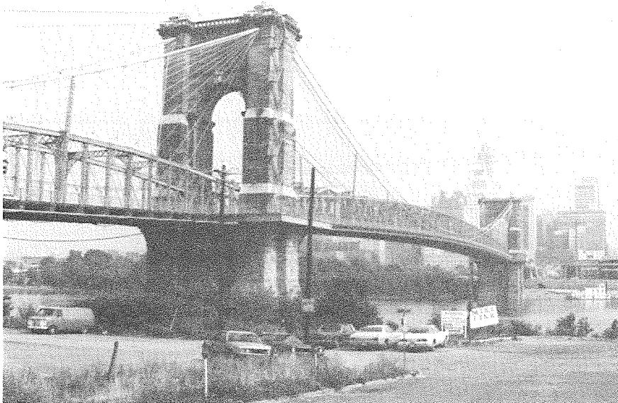
The Covington-Cincinnati Suspension Bridge was designed and built by the noted engineer and architect John Roebling. When completed in 1866, it was the longest suspension bridge in the world. (SF #34)
