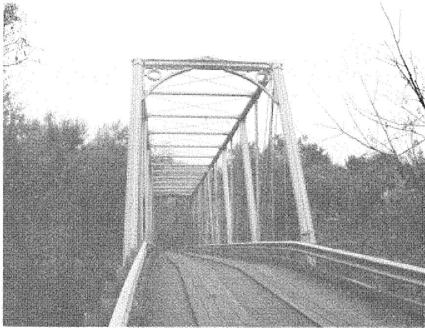
End perspective of Four Mile Bridge over Cumberland River in Bell County. This 1873 Warren through truss has cast iron top chords and eyebar diagonals, factors that made early Warren through trusses susceptible to failure. (SF #54)
