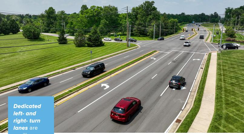
left- and right- turn lanes are auxiliary lanes that allow vehicles to safely turn at intersections without interfering with through traffic.
