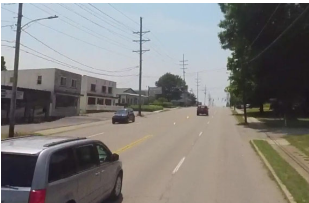
Before Road Reconfiguration
