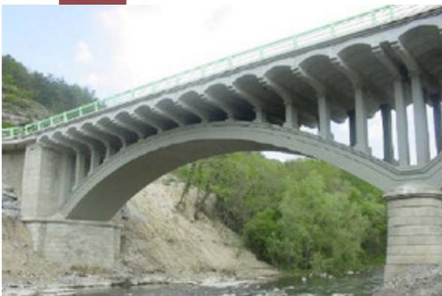
The haunched deck beam image of River Road shown on the right was compared to the straight deck beam and the open spandrel arch designs. The haunched and open spandrel arch generally scored higher than the straight deck beam design sketches.
