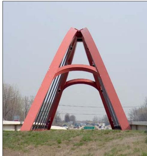
Inclined Arch Rib & Cables
