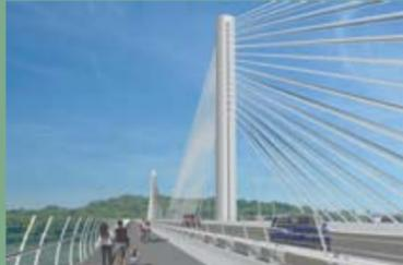
The pedestrian walk-and-bike path along the East End Bridge features a curved 6' fence with horizontal cables, which provide safety as well as an unobstructed view.
