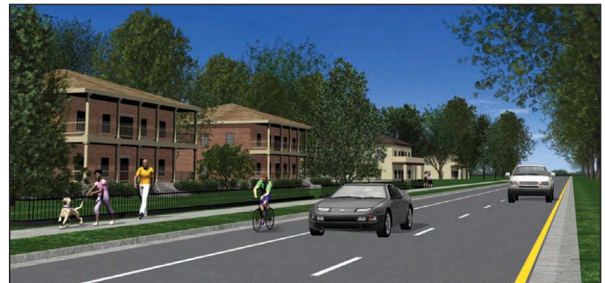
Newtown Pike Extension will include wide sidewalks, bicycle lanes and on-street parking in locations.
