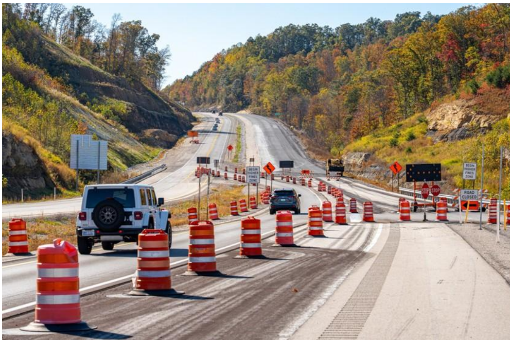
Part of the Mountain Parkway Expansion
