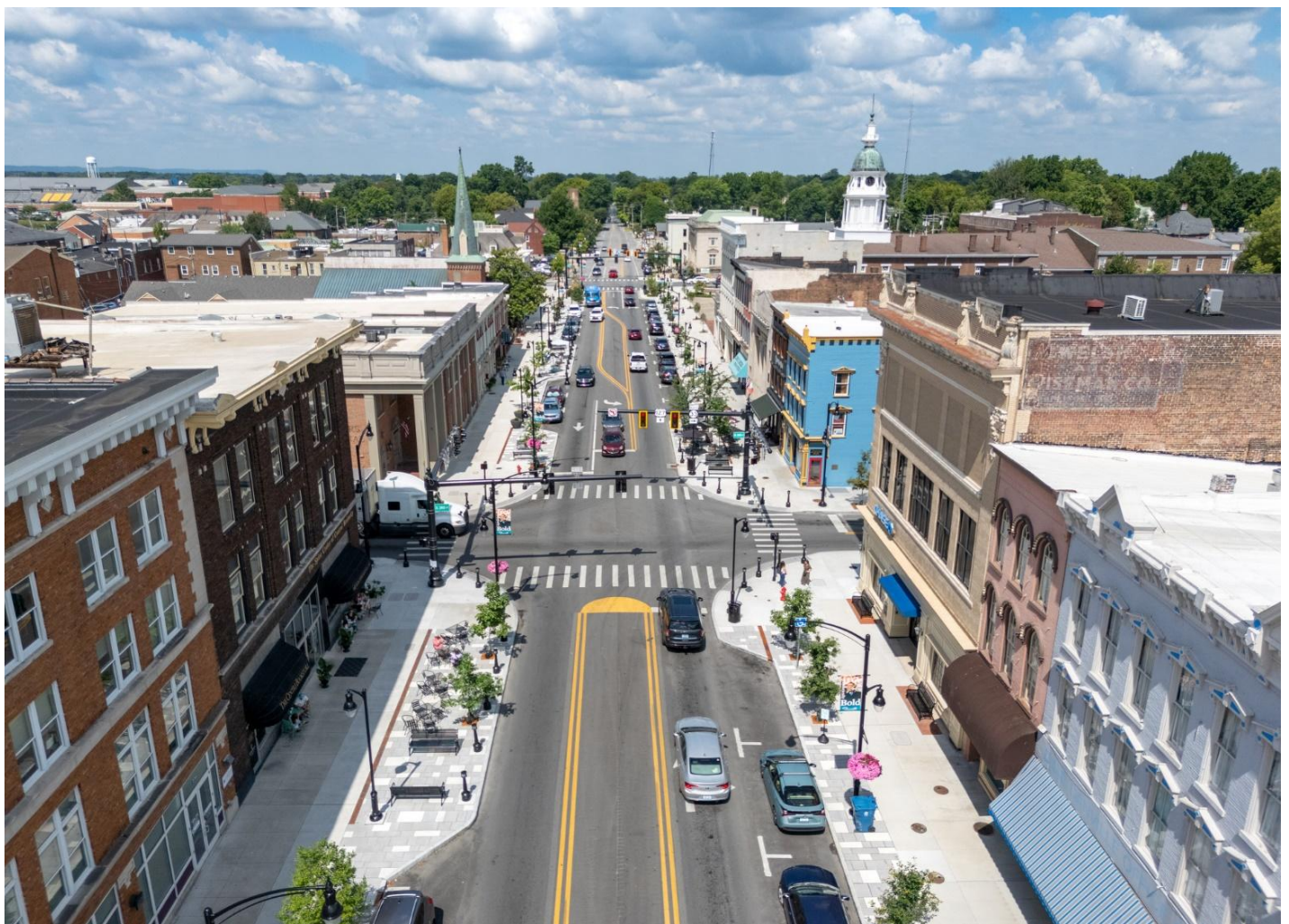
Main Street Reconstruction Project in Downtown Danville, Kentucky
