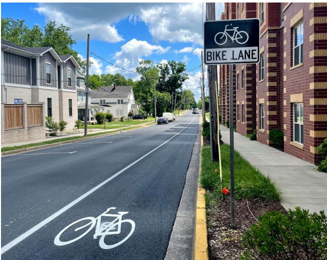
Complete Streets Project - Kentucky Street in Bowling Green
