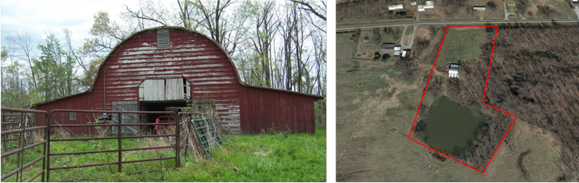
Figure 4: BA-180, NRHP-eligible barrel-vault mule barn
