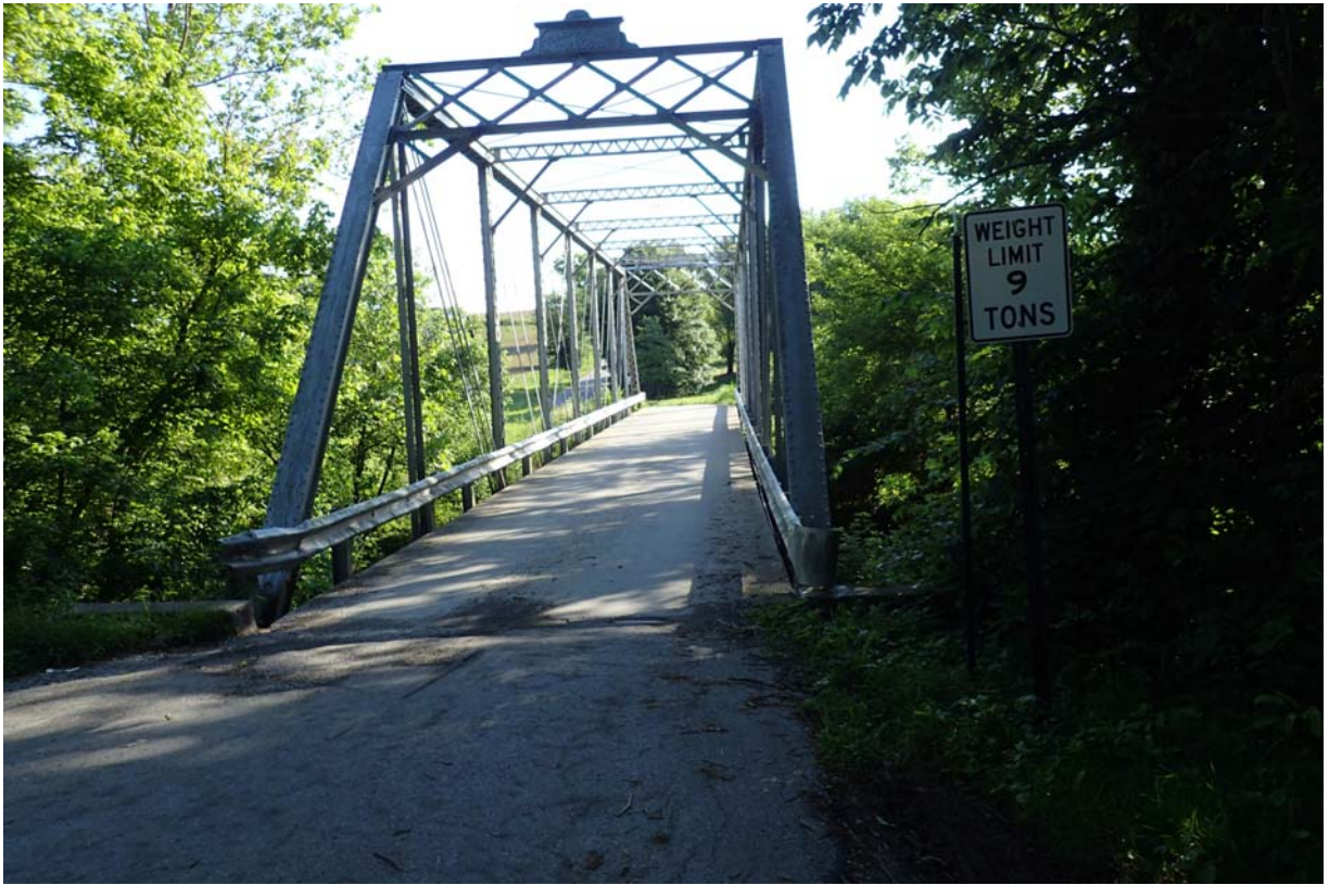
View of the west 9 tons posting.
