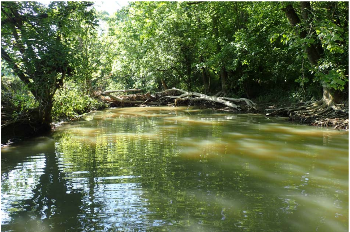
View of heavy drift blocking the channel~ 75' upstream of the bridge.
