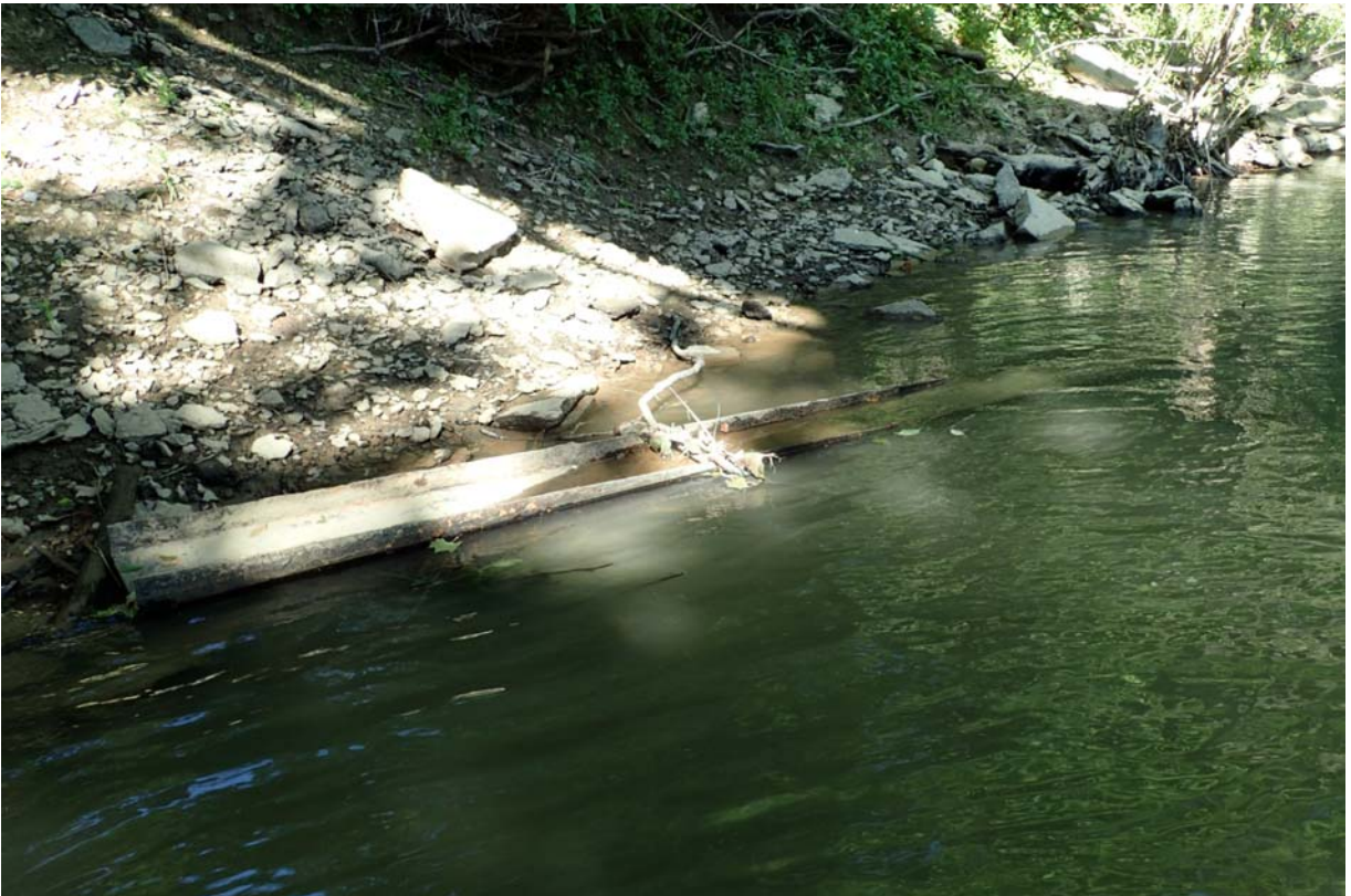
View of the retrofitted floorbeam that WAS welded to the bottom flange of the original floorbeam at L2. It has fallen off.
