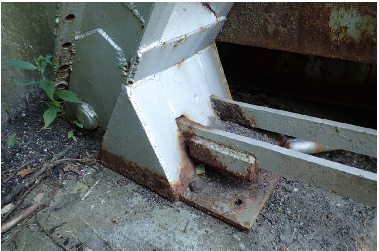
Typical view of the upstream bearing at the west abutment.
