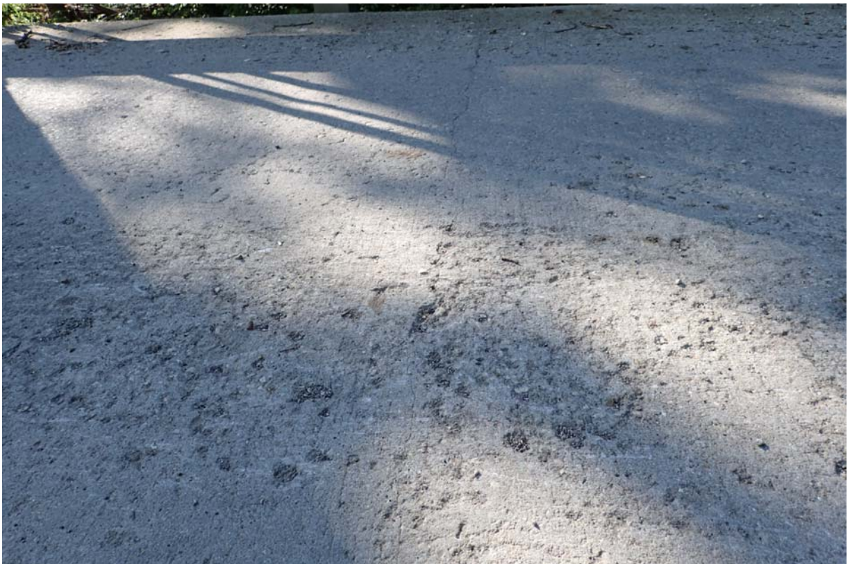
View of a minor sized full width transverse crack in the wearing surface between the L1 and L2 connections.
