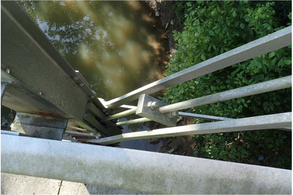
View of retrofit at upstream L2.
