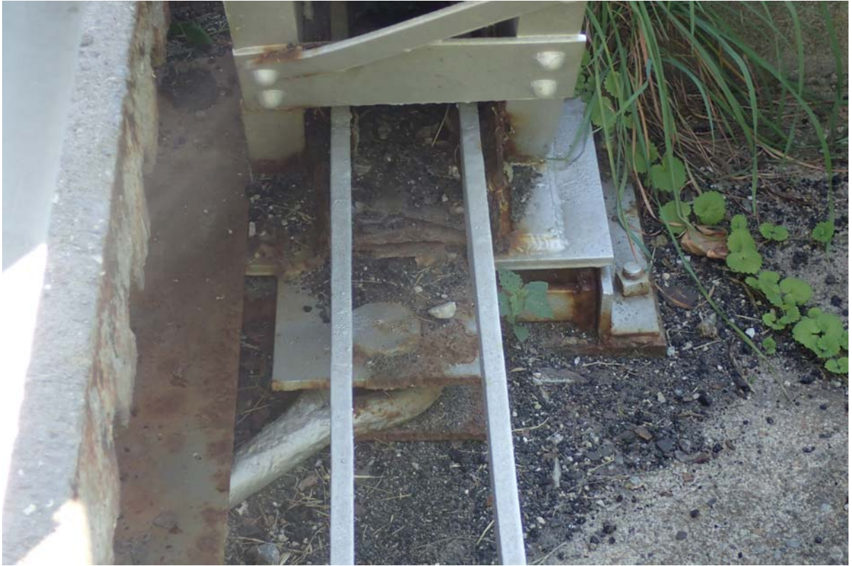
View of the upstream east bearing.
