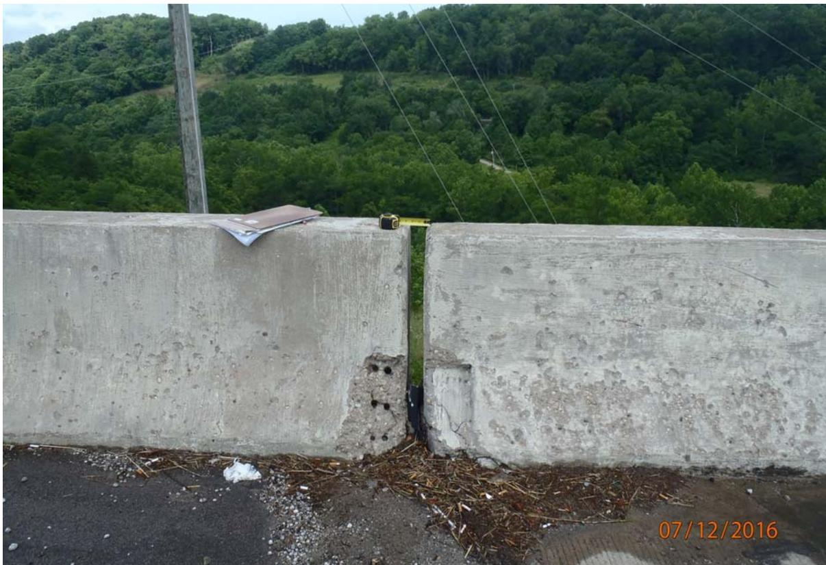
View of lateral offset between the downstream barrier wall at abutment 1. Note the barrier wall sliding plates have torn off due to the horizontal movement.
