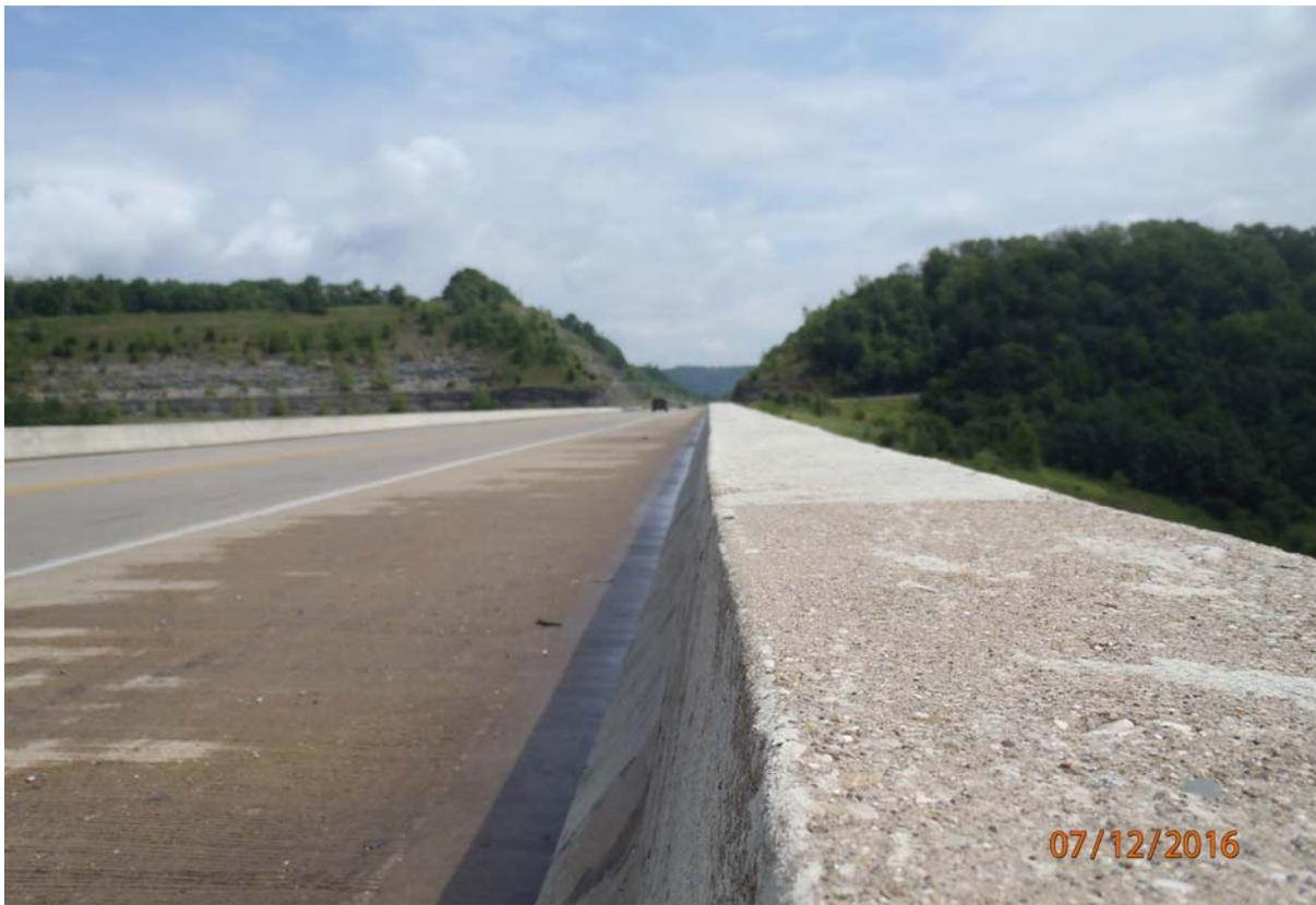
View sighted along the upstream barrier wall looking from abutment 1. Note the top of the wall appears to be wavy throughout, this is consistent with the driving surface; traffic appears to bounce while crossing the structure in both directions.
