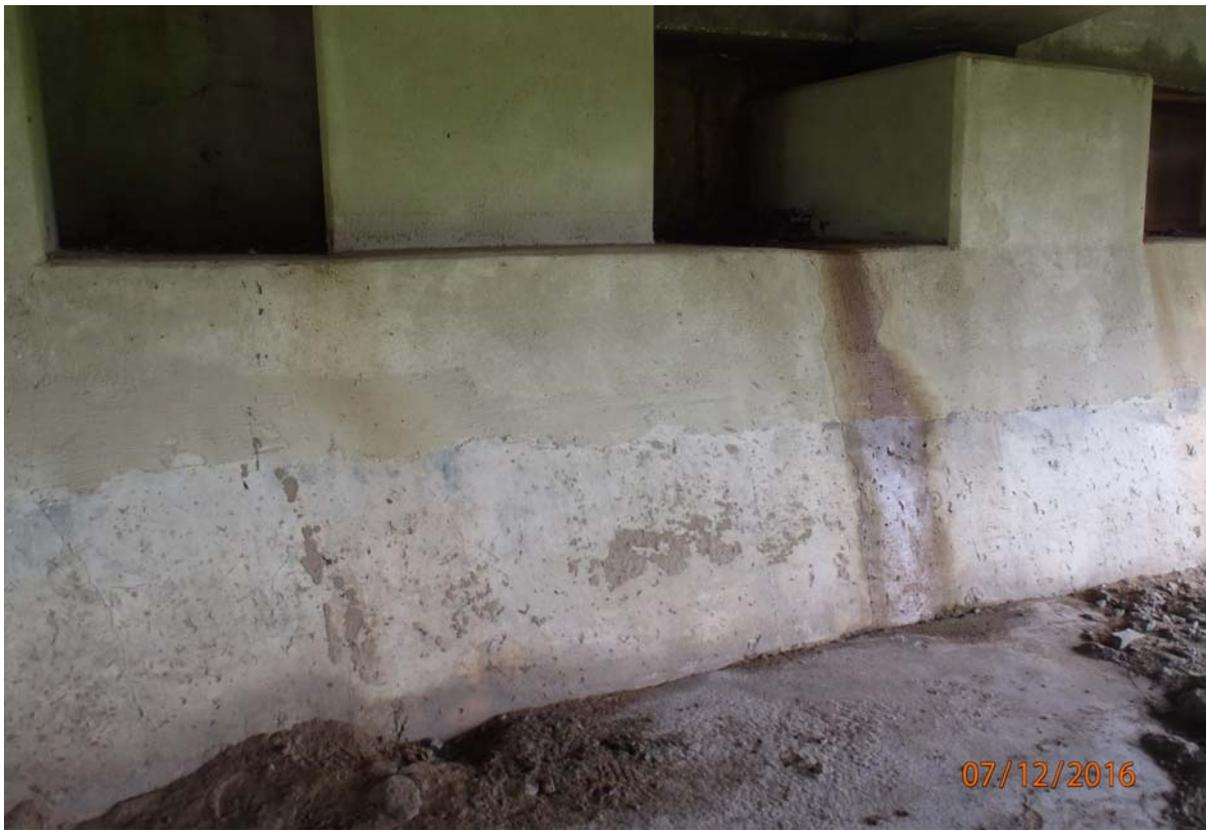
View of cracking in the face of abutment between beams 2 and 3.
