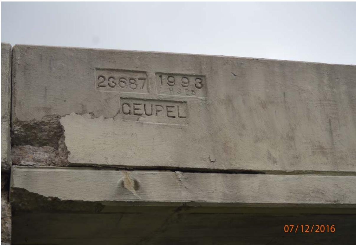
View of the date, design loading, plan number, and contractor stamp located on the upstream face of the downstream barrier wall at abutment 6.
