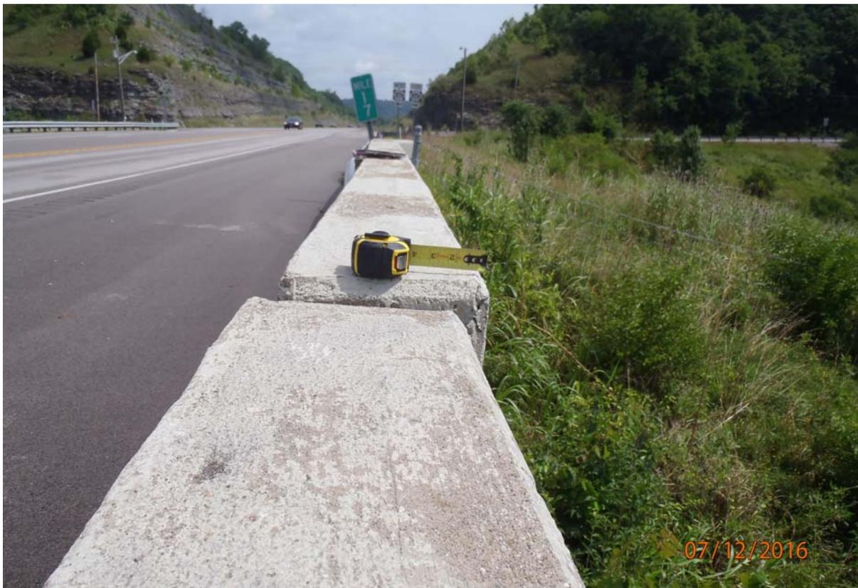
View of the horizontal offset between the upstream barrier wall at abutment 6. Note the entire superstructure appears to have moved towards the downstream at this location. **16/75**
