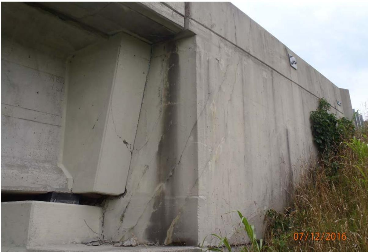
View of shear cracking with efflorescence and rust staining extending from the downstream wingwall (Wingwall A per plans) into the back-wall of the upstream face of abutment 1.
