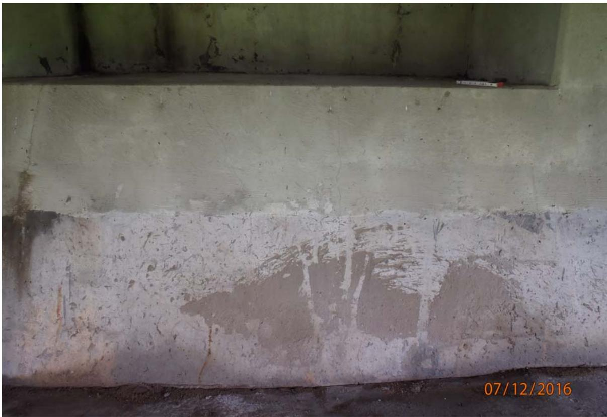
View of cracking in the face of abutment 6 between beams 3 and 4.
