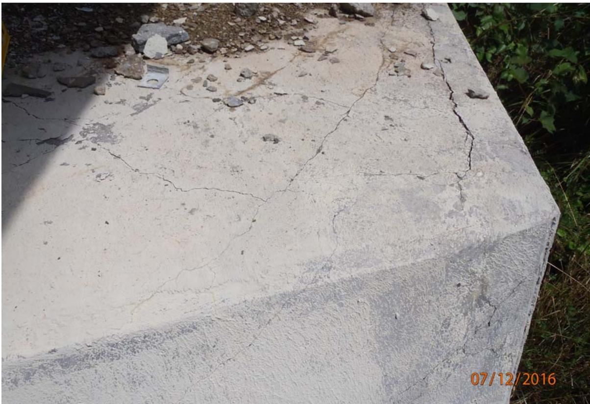
View of cracking present on the abutment seat upstream of beam 1.
