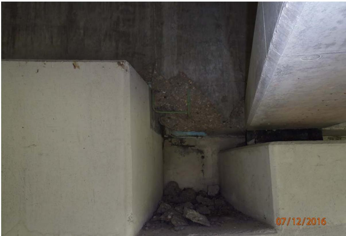
View of the diaphragm and shear block between beams 4 and 5 (beam 5 on right). Note the diaphragm is spalled with exposed reinforcing steel without section loss. In addition note the superstructure is pressed tight against the abutment back-wall the entire length of the abutment.
