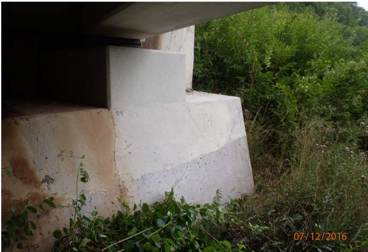
View of cracking under beam 1, upstream of beam 1, and downstream of beam 1 in the face of abutment 6.
