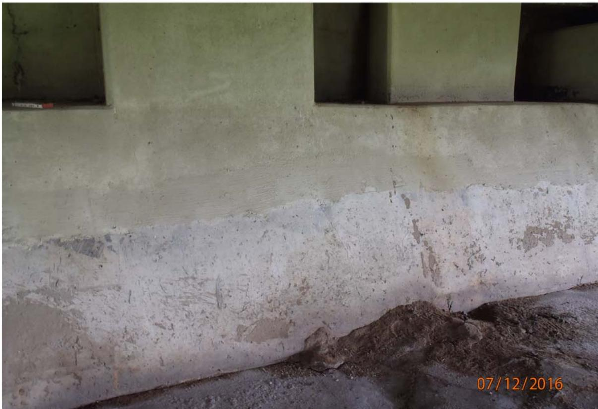
View of cracking in the face of abutment 6 under beam 3.
