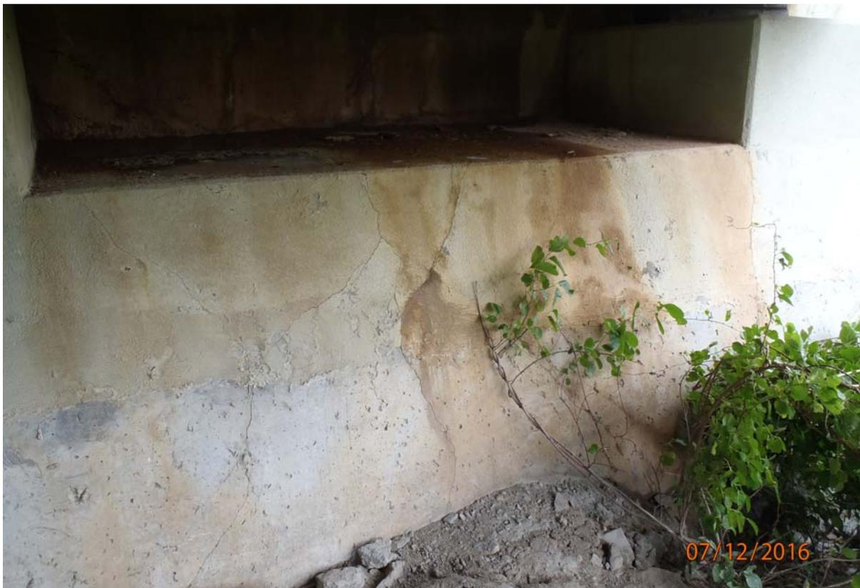
View of cracking in the face of abutment 6 between beams 1 and 2.
