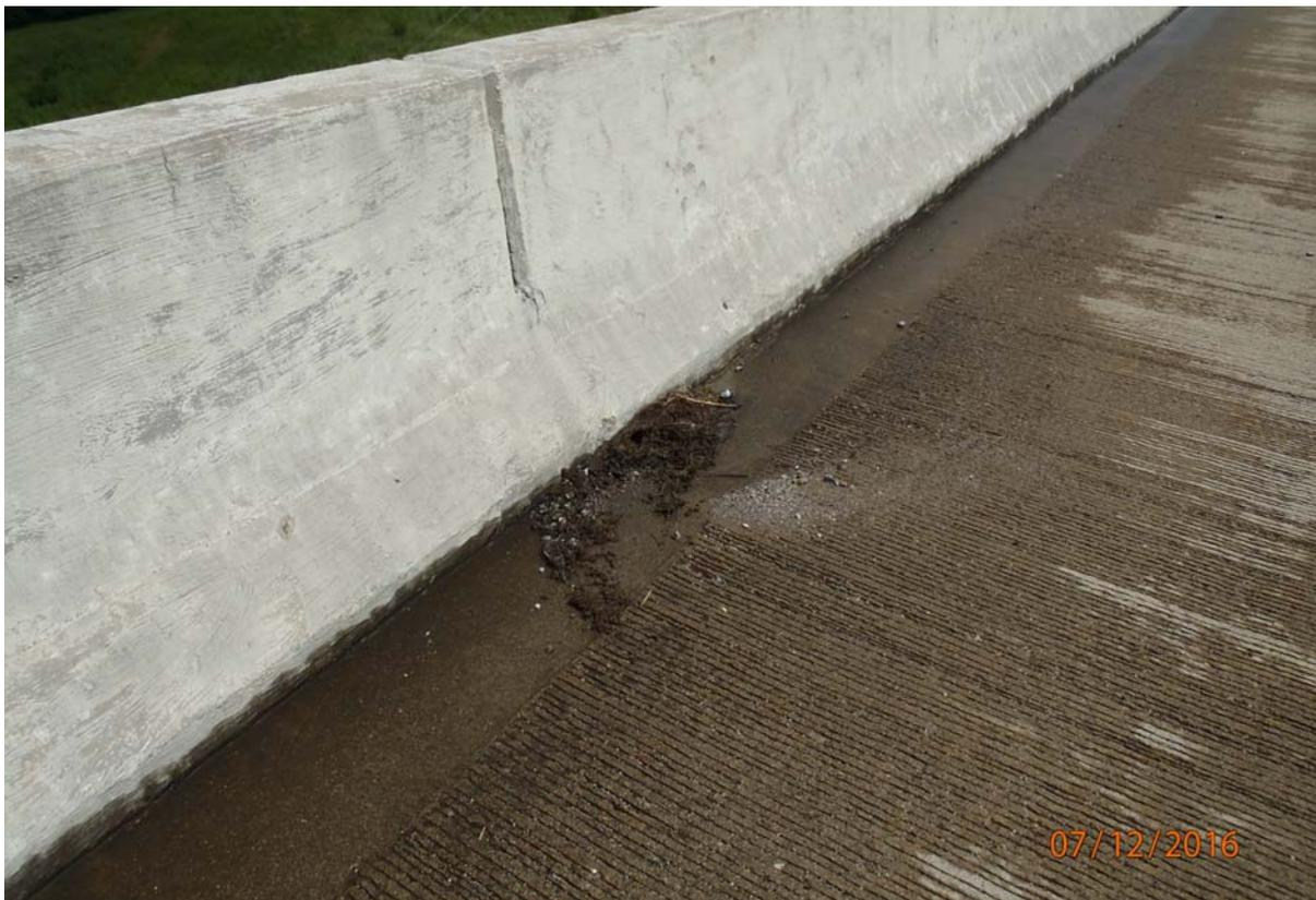
Some of the deck-drains are open, however a large number are 100% blocked with debris as shown above.
