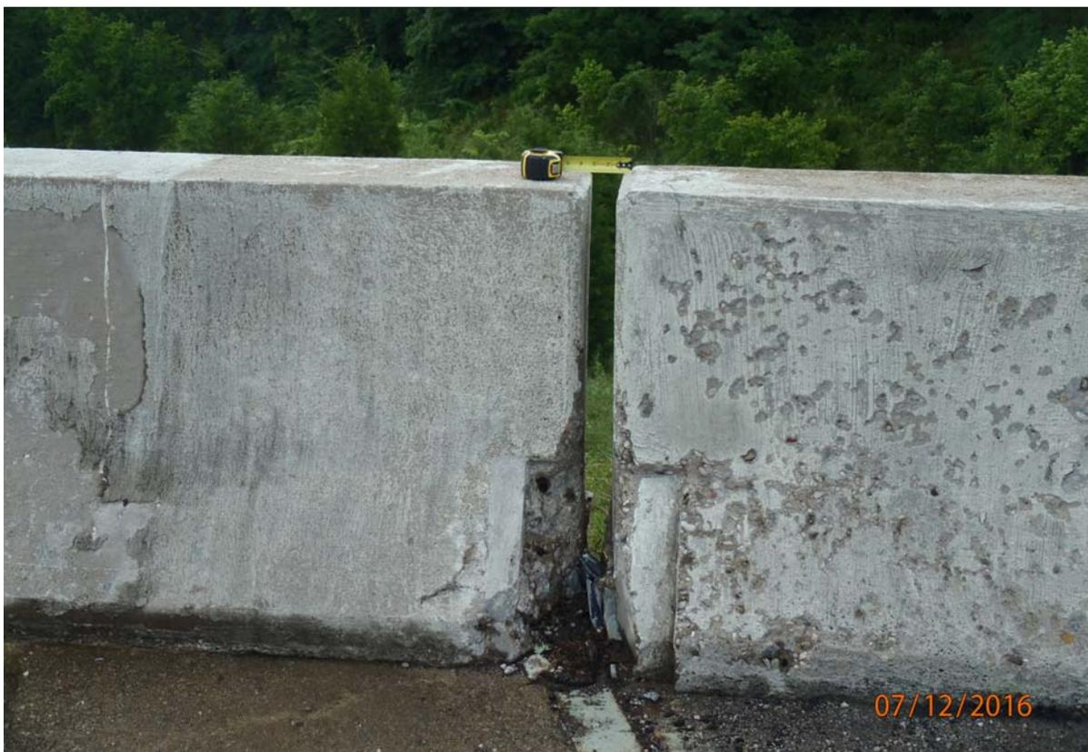
View of lateral offset between the upstream barrier wall at abutment 1. Note the barrier wall sliding plates have torn off due to the horizontal movement.
