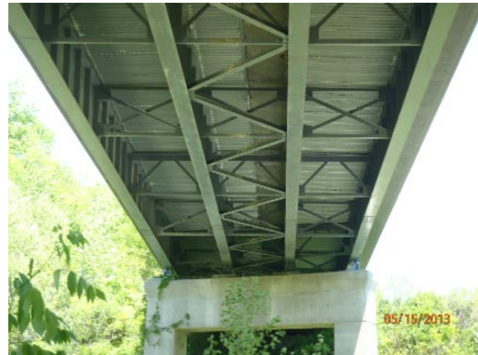
View of span 2.
