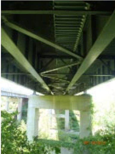
View of span 3 and pier 3.
