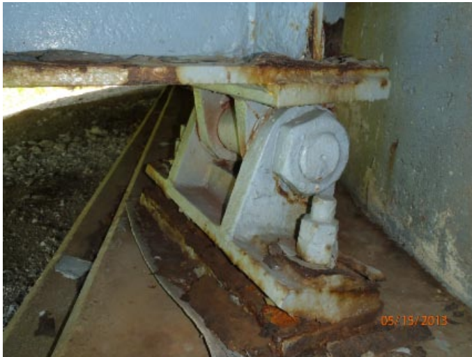
View of the north bearing at abutment 1.
