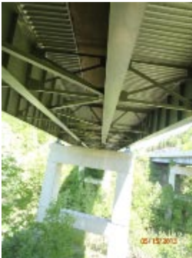
View of span 1 and pier 2.
