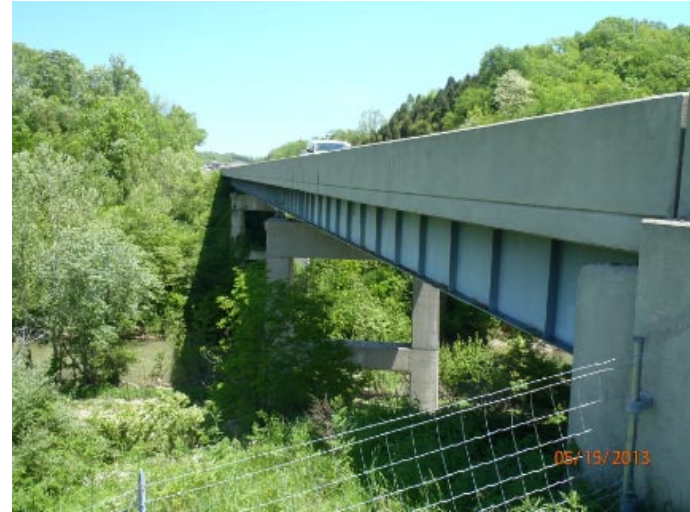
View from the north near abutment 1.
