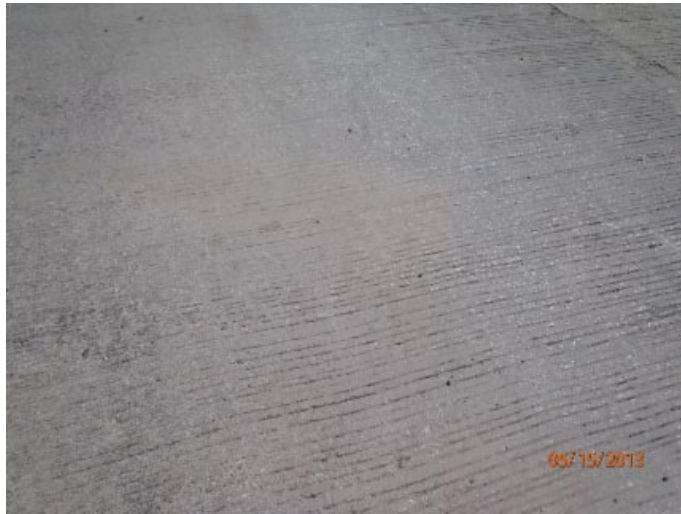
Typical view of the wearing surface.
