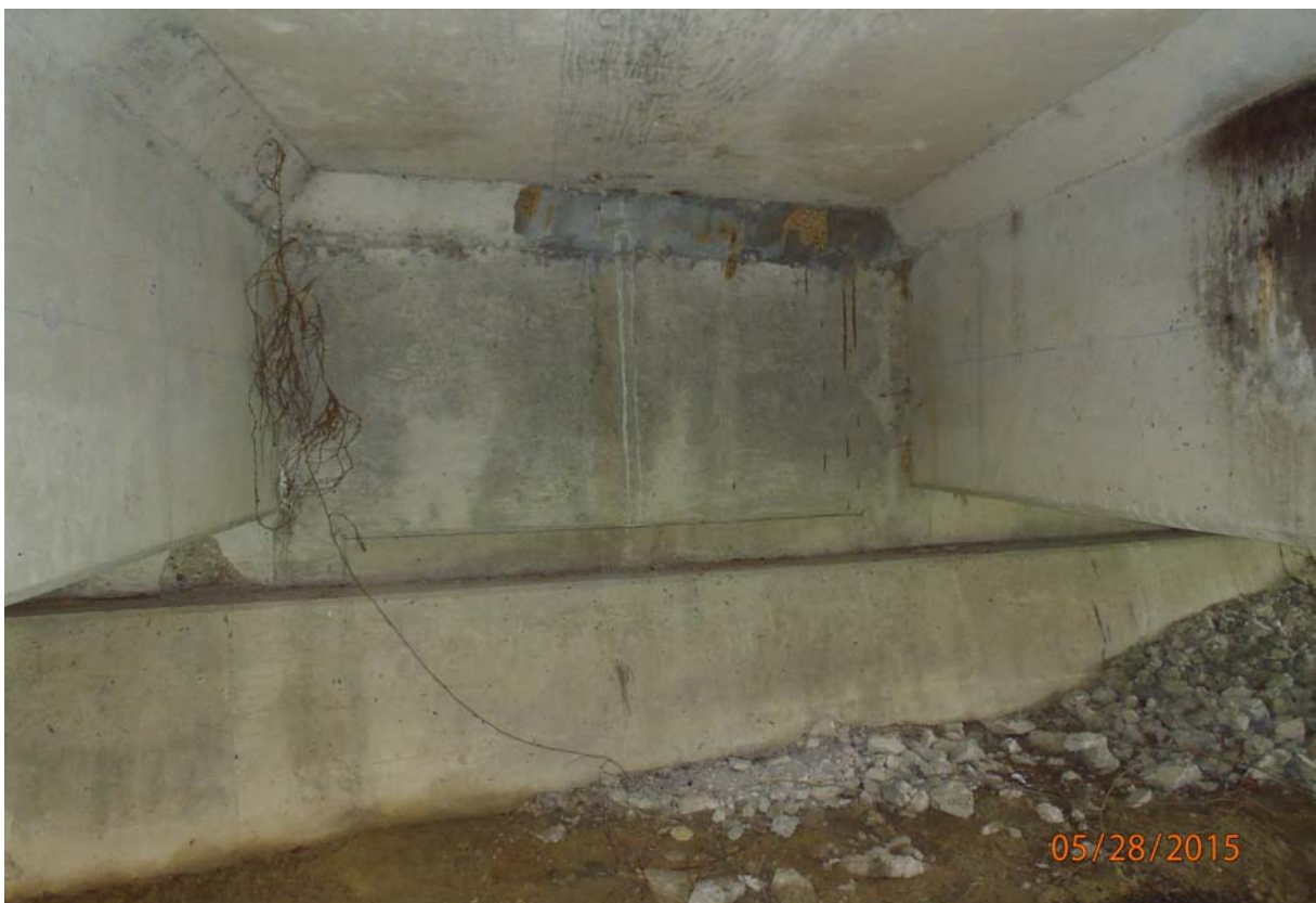
View of the abutment and diaphragm between beams 2 & 3 @ abutment 1.
