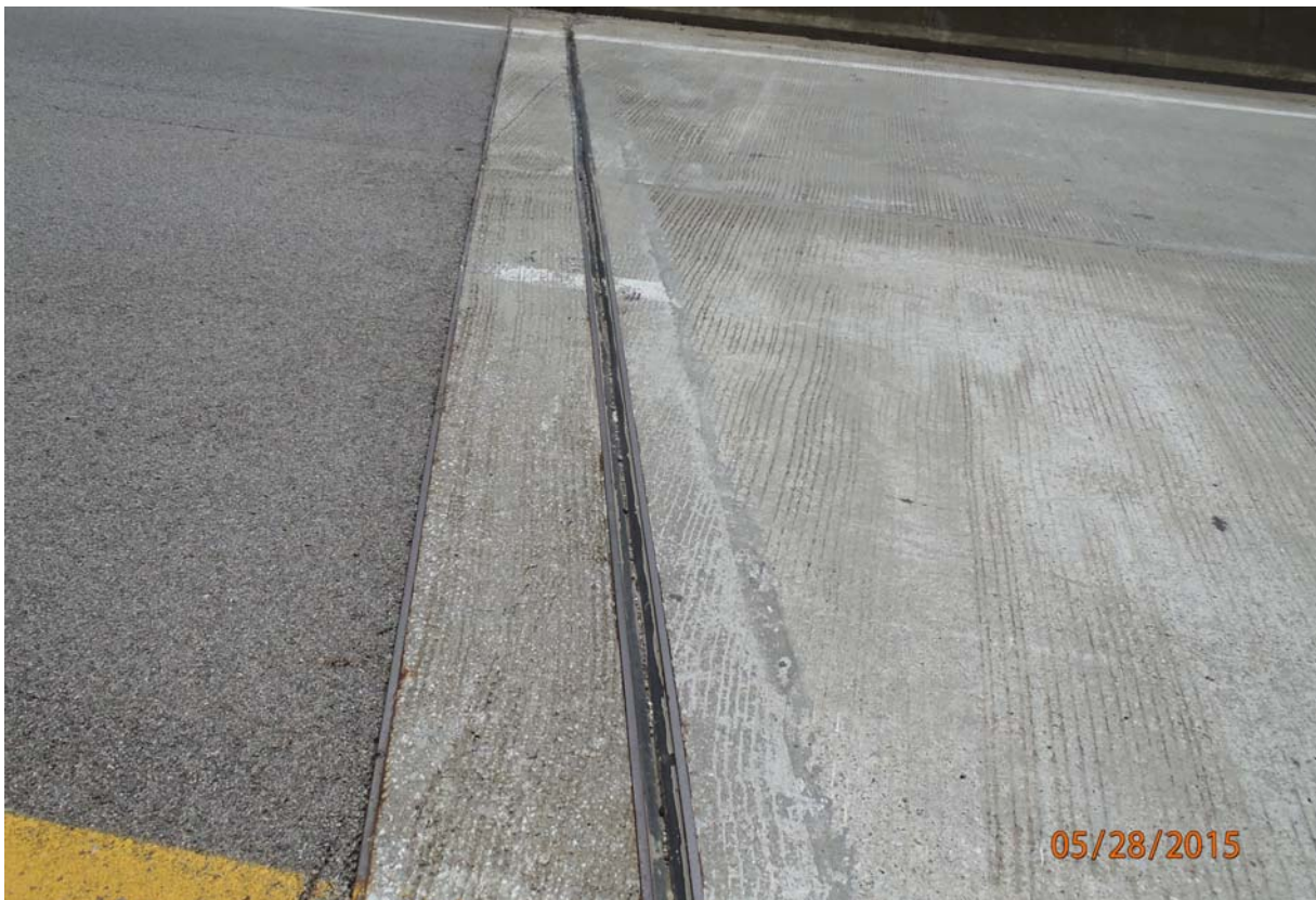
View of the deck joint at abutment 5.
