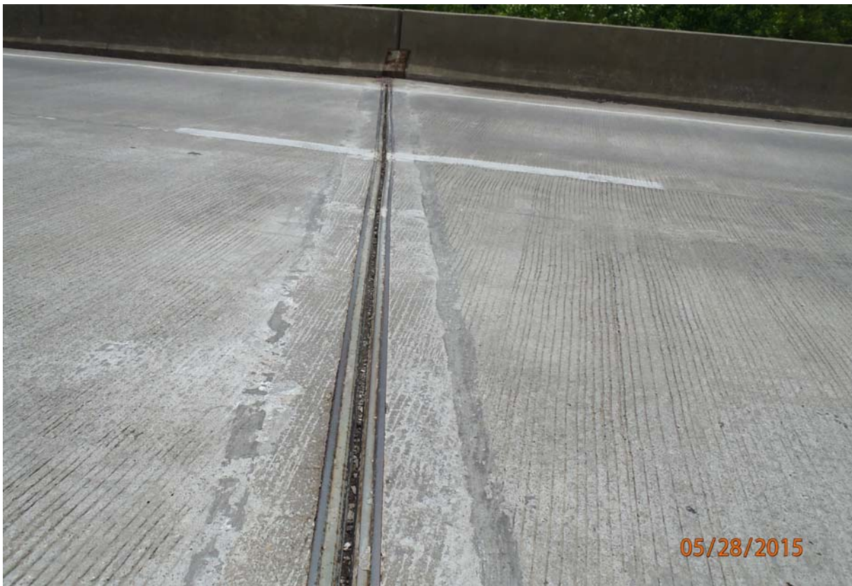
Deck joint over pier 2.
