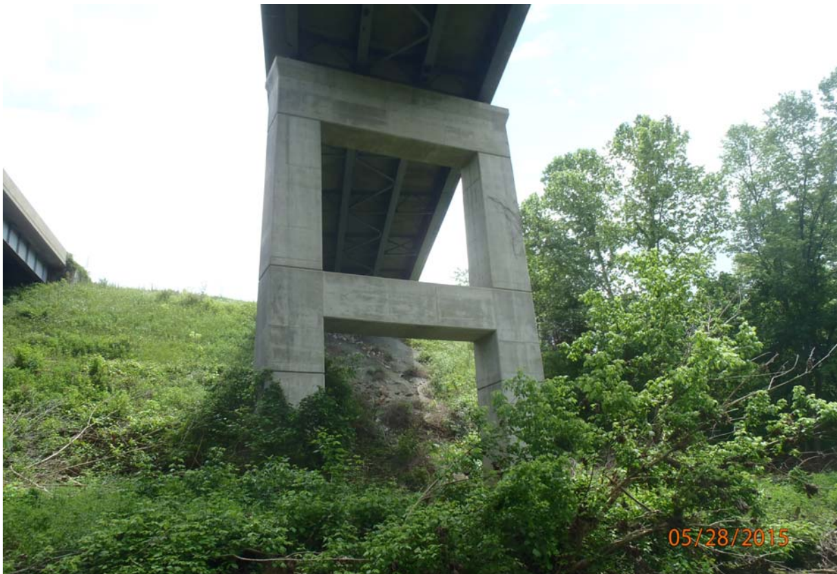
Looking at the west face of pier 4.
