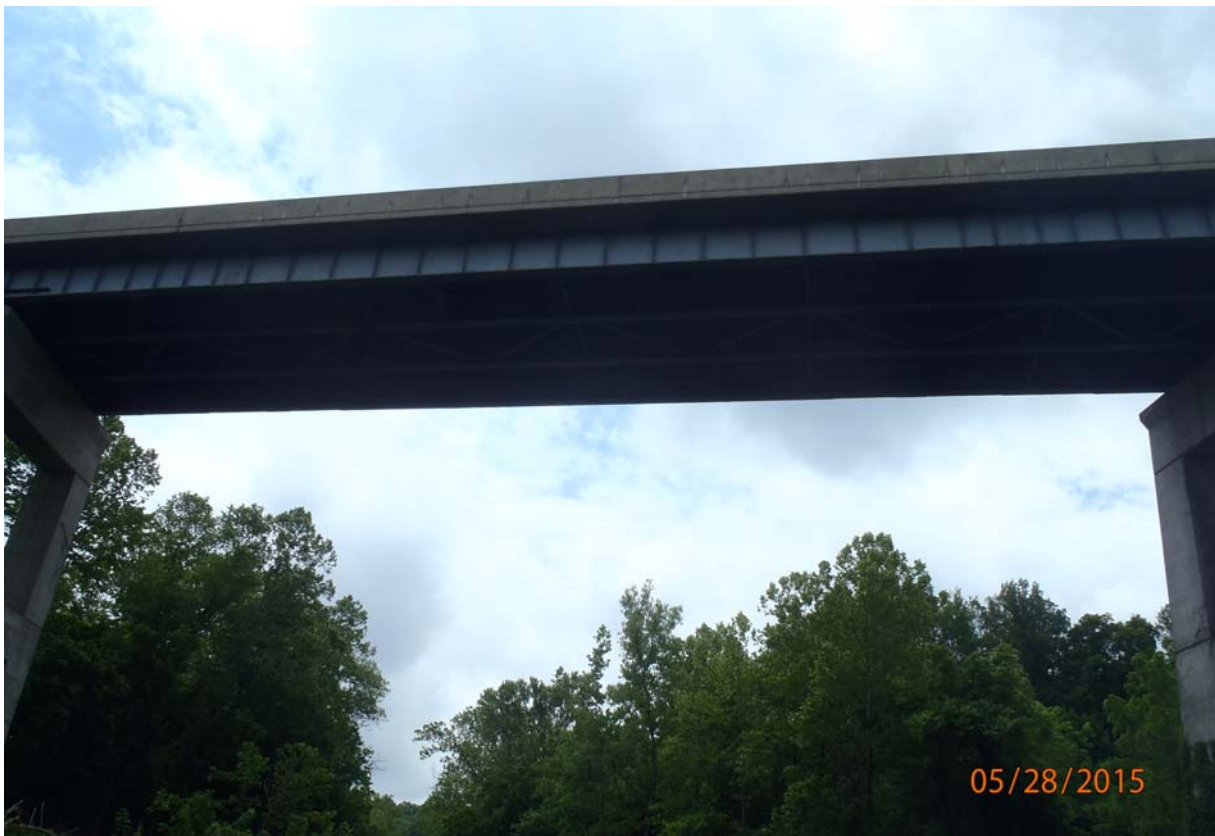
Elevation view of span 3 from upstream.
