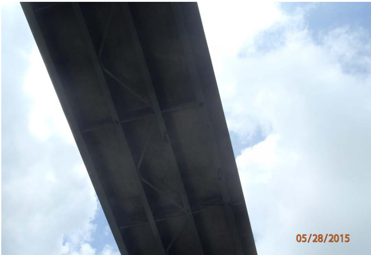
Looking up at the underside of span 3.
