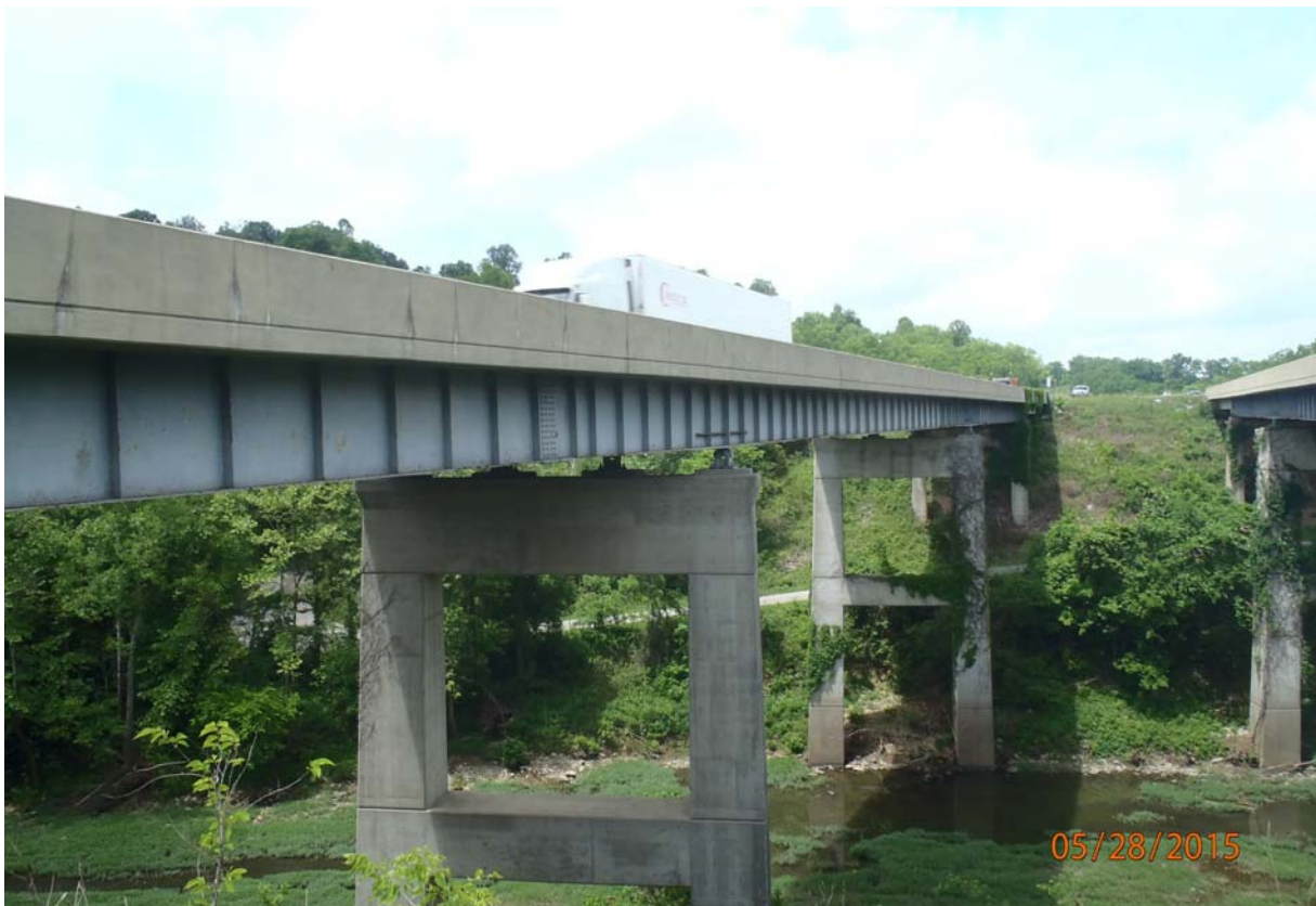
Elevation view from upstream and the east approach.
