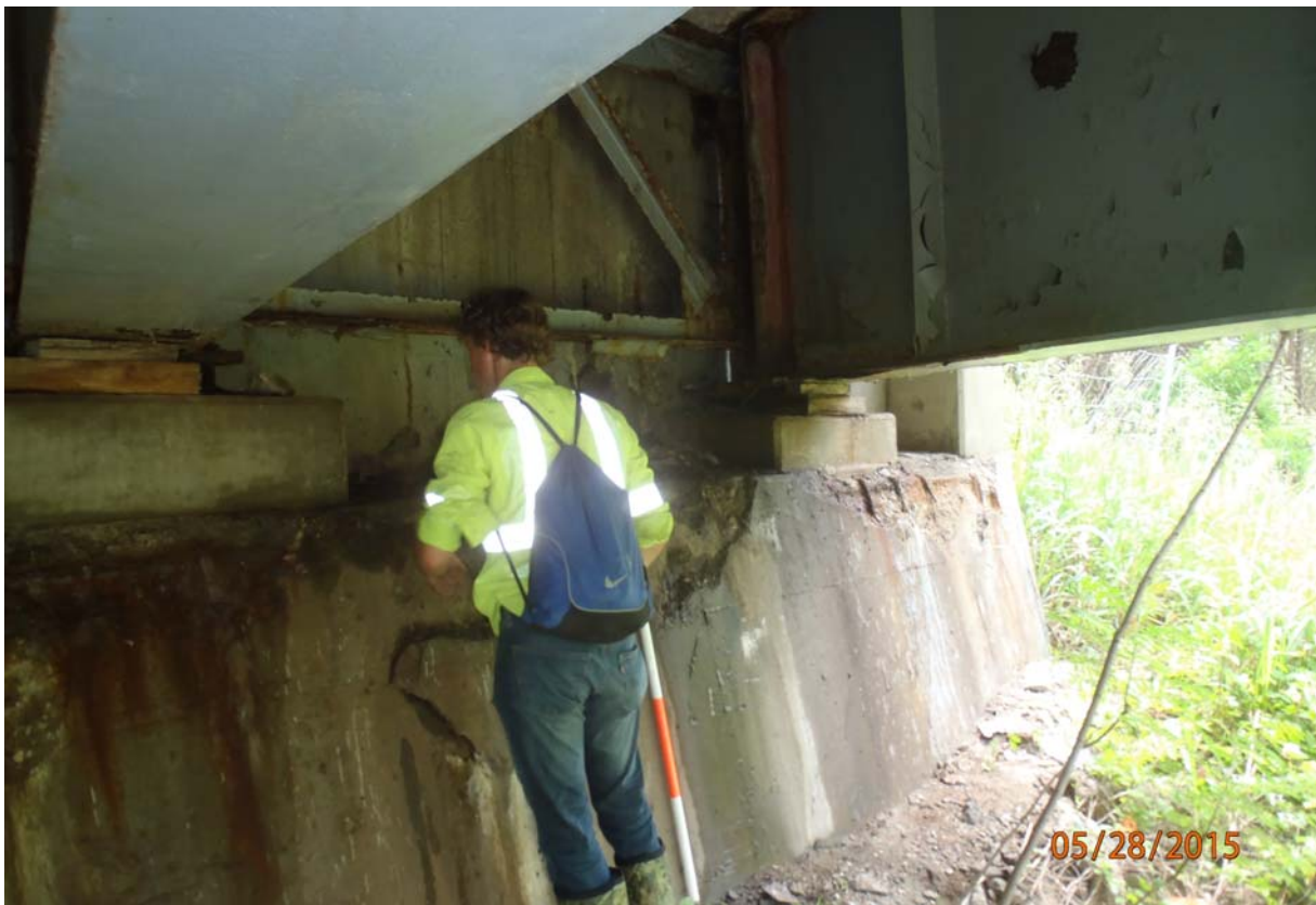
View of inspection of the bearing of beam 3 @ abutment 5.
