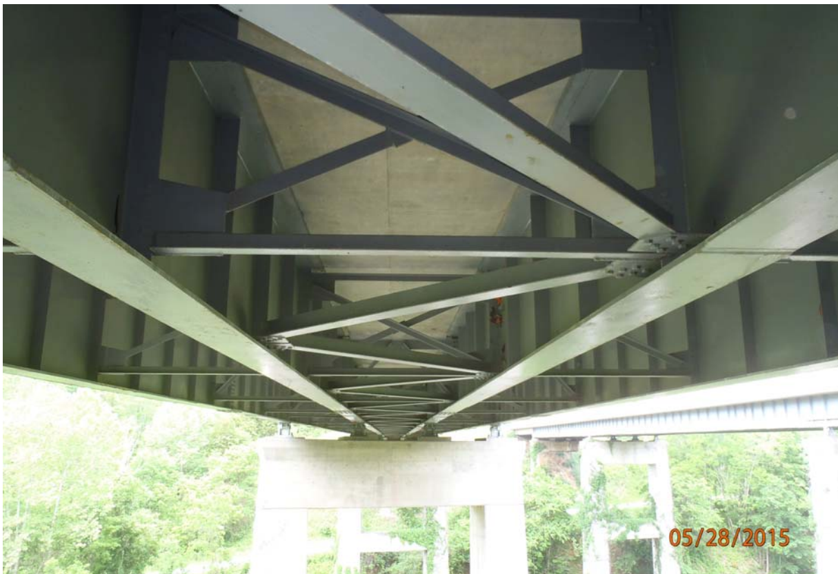
view of the underside of the superstructure in span 4.
