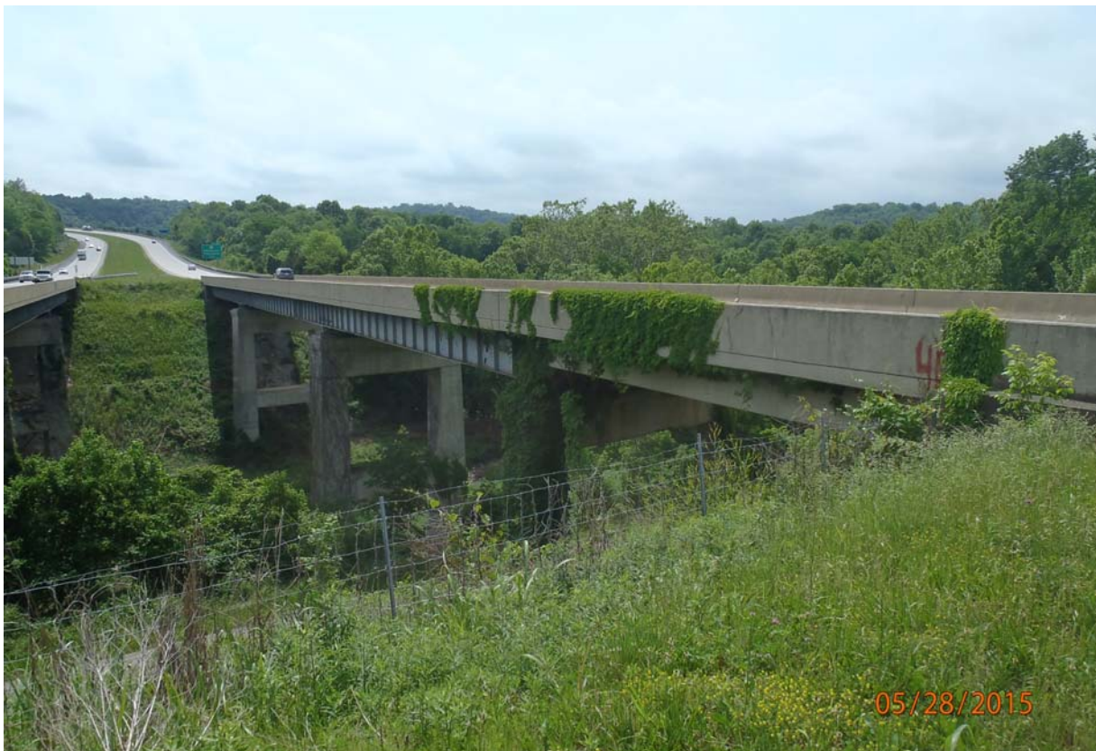
Elevation view from upstream and the west approach.
