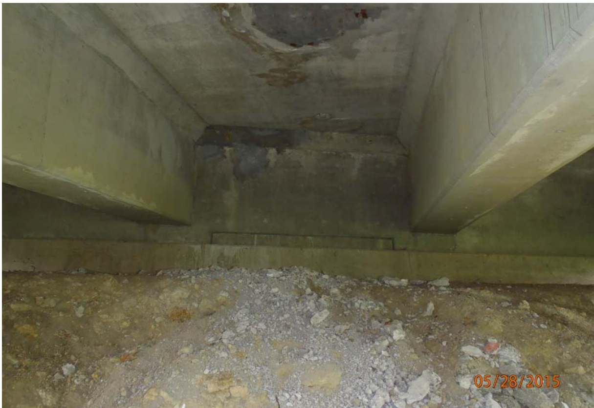
Looking at the west abutment (abutment 1) between beams 2 & 3.
