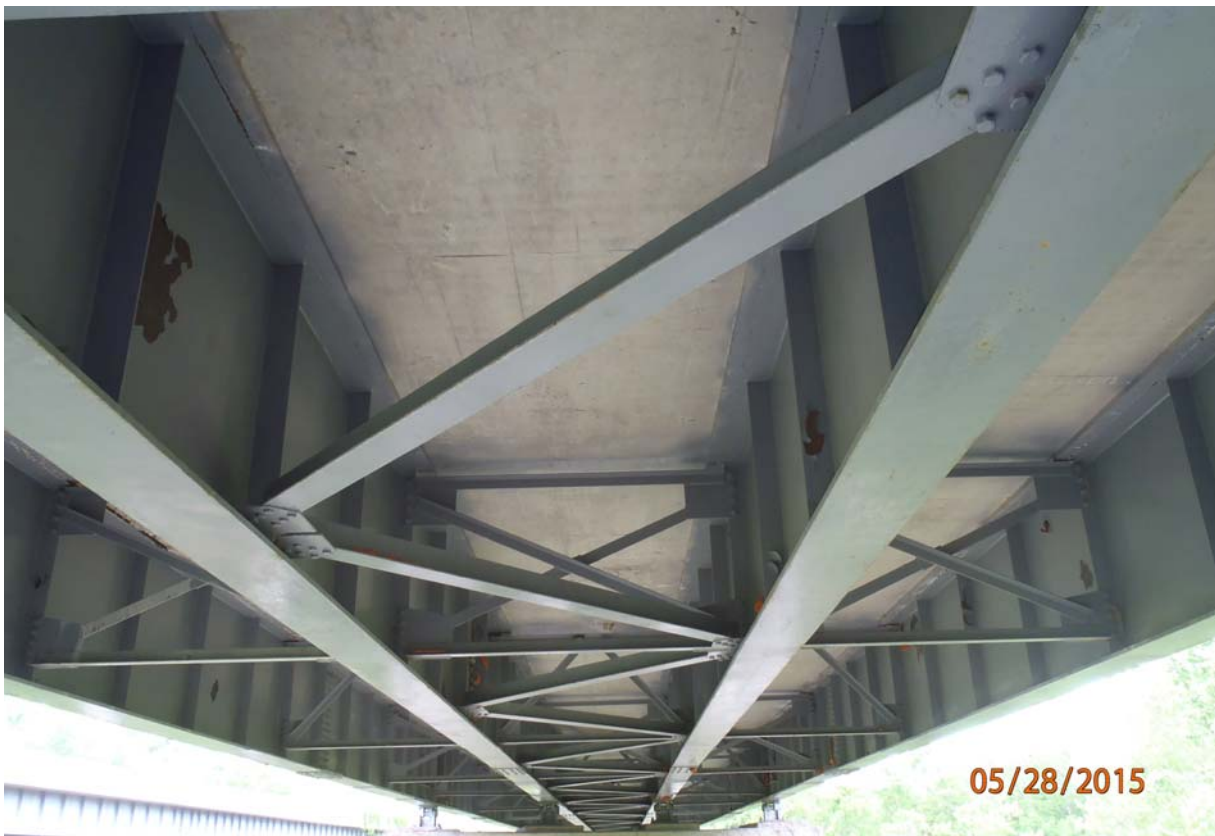
view of the underside of the superstructure in span 4.
