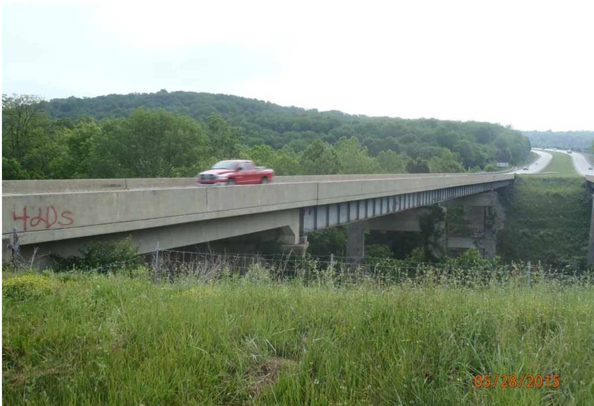
Elevation view from downstream and the west abutment.
