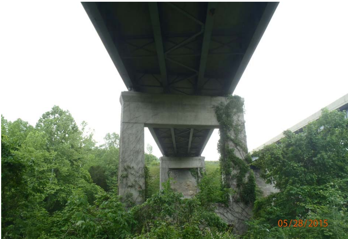
Elevation view of the west face of pier 3. Note the heavy vegetation growth.
