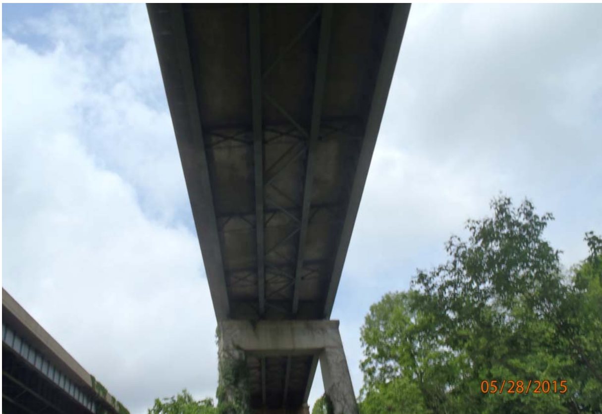
Looking up @ the underside of span 3.
