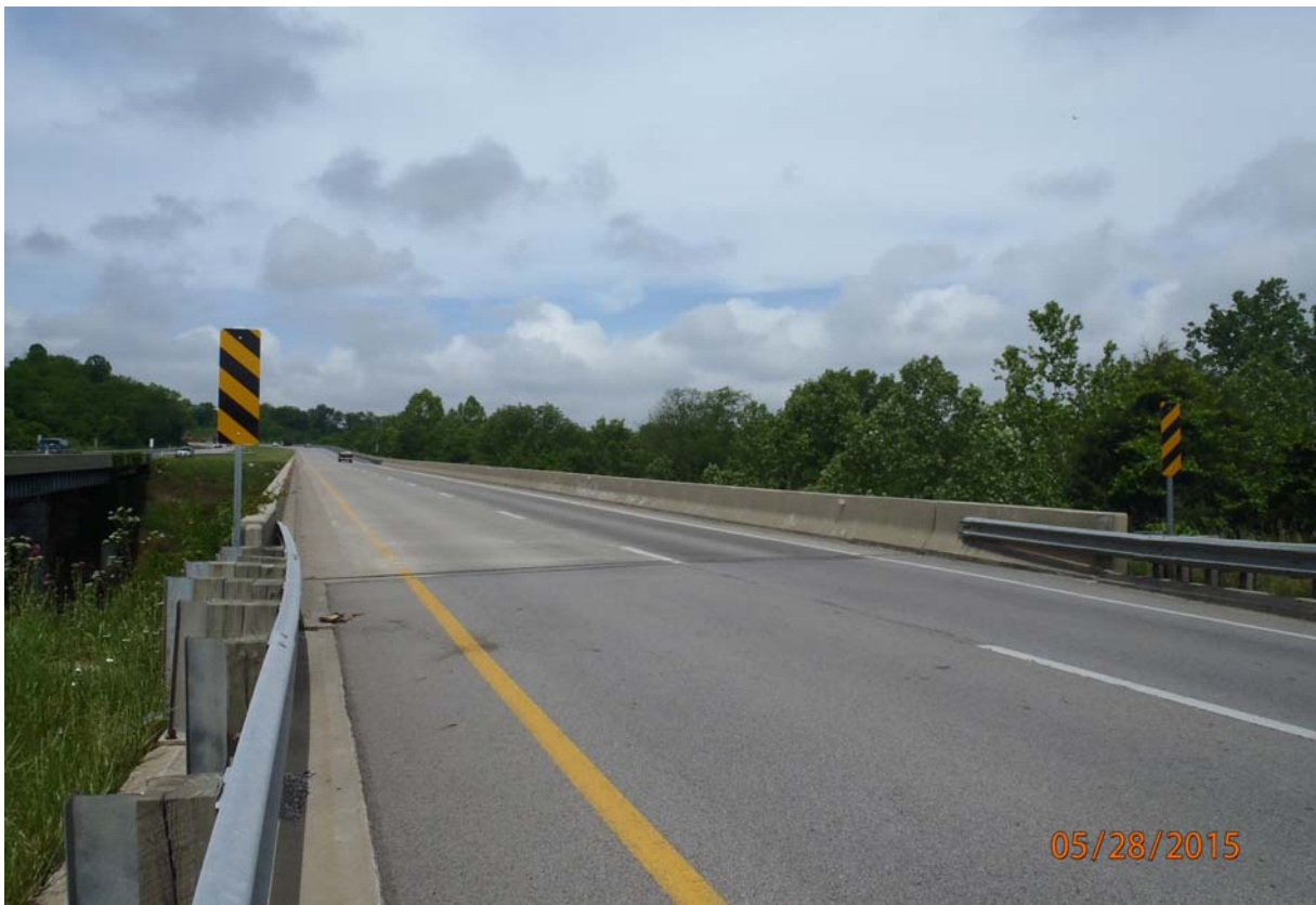
Endview from the east approach.
