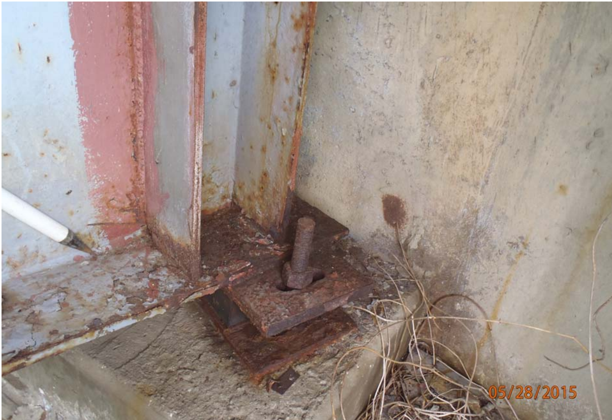
Downstream face of beam 4 @ abutment 5.
