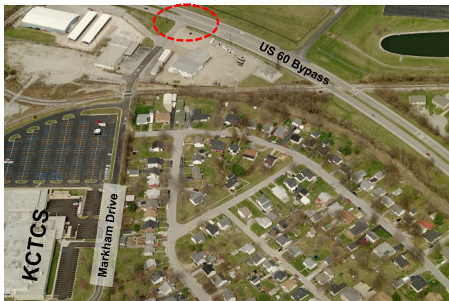
Figure VII-15. US 60 Bypass at Markham Drive
