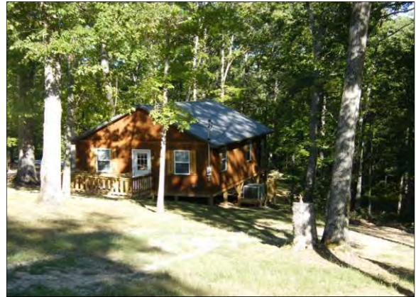
Photograph 4-19: Cabin at Lawrence County Recreation Area
