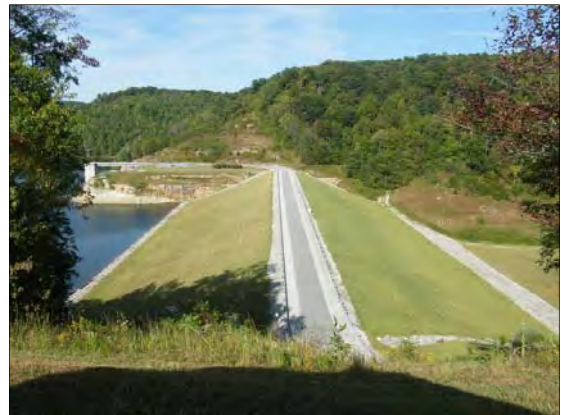
Photograph 1-1: Yatesville Lake Dam
