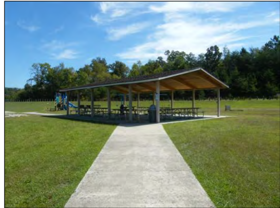
Photograph 4-21: Picnic Shelter at Barker Run Marina
