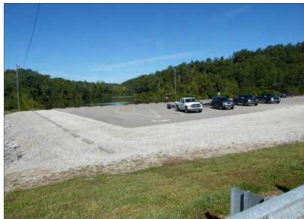
Photograph 4-4: Parking Area at Rich Creek Launch Ramp
