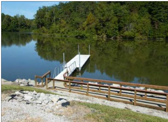
Photograph 4-3: Courtesy Dock at Rich Creek Launch Ramp
