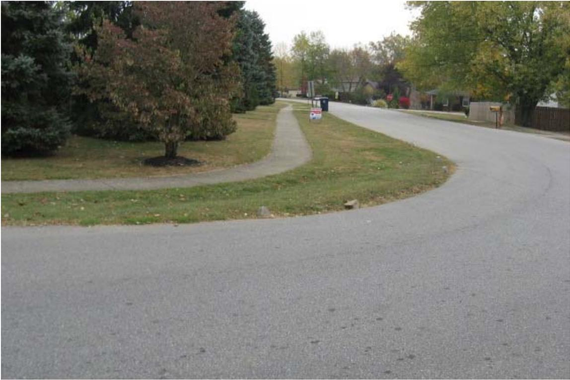
No pipes or swales to contain water at intersection of Ashbrooke Drive and Raintree Court.
