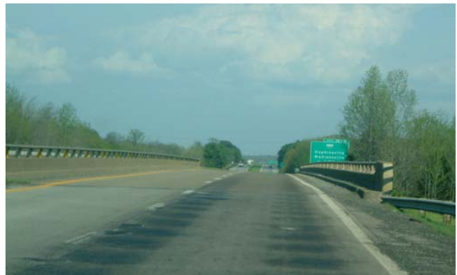
The lateral clearances (widths) of mainline bridges along the Parkways often do not meet AASHTO guidelines, which require bridge widths equal to the paved roadway plus shoulder widths.
