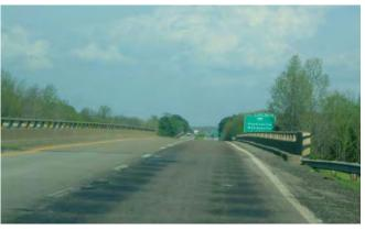
The lateral clearances (widths) of mainline bridges along the Parkways often do not meet AASHTO guidelines, which require bridge widths equal to the paved roadway plus shoulder widths.
