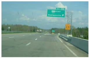
Entrance ramps and exit ramps at many interchanges along the two Parkways do not appear to meet minimum interstate guidelines for lengths and tapers.
