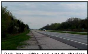
Both lane widths and outside shoulder widths along the two Parkways generally meet Interstate design guidelines.
