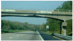
The recommended vertical clearance (height) of bridges over the Parkways is 16 feet over each of the travel lanes and the outside shoulders.
