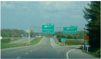
Interchanges have design guidelines for design speed, typical sections, horizontal and vertical alignment that are similar to mainline sections, along with added requirements for merge and weaving sections.
