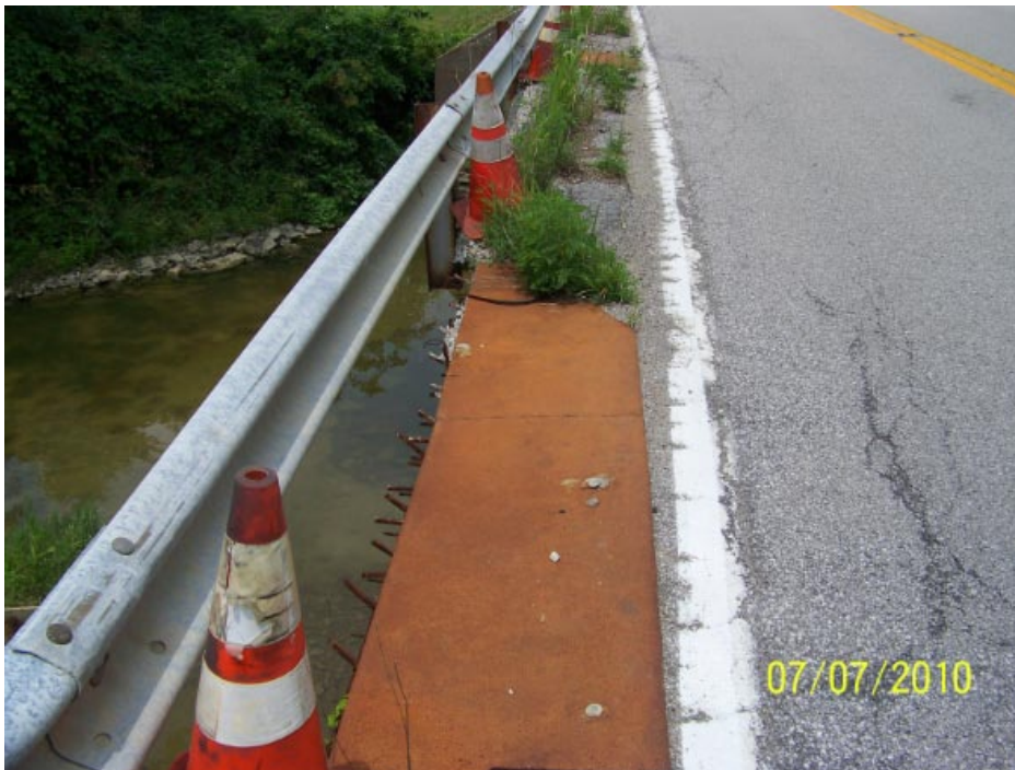
West edge supported by steel plates.
