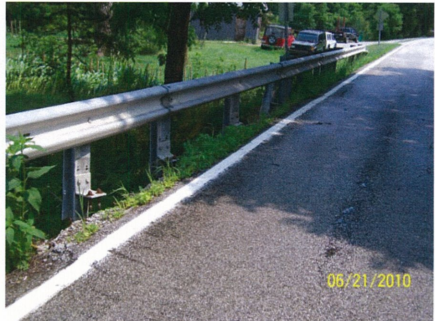
Rail posts are dangling from the railing
