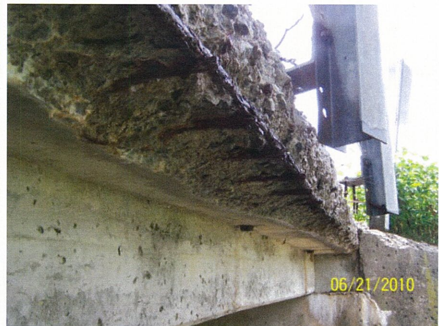
Railing posts are hanging from the rails
