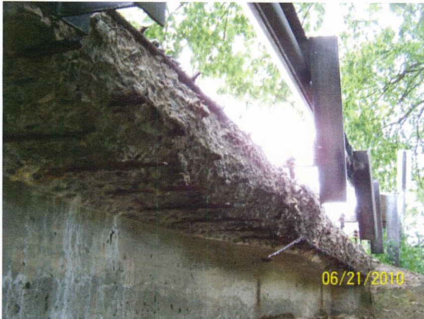
Railing posts are not attached
