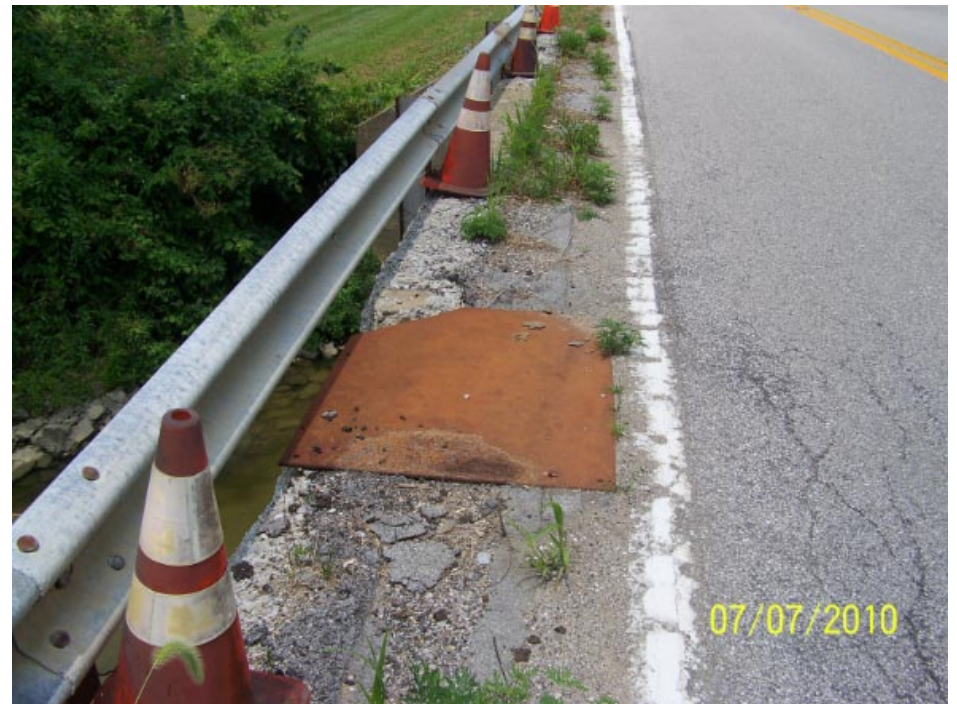
West edge supported by steel plates.
