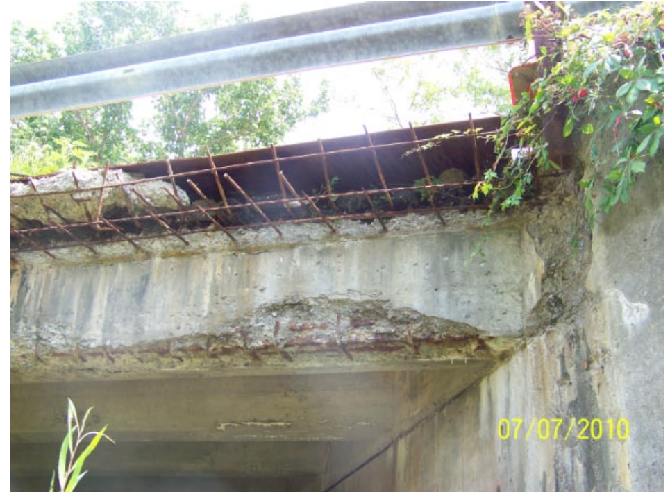
Span 1 west edge; Girder 1 spalled.
