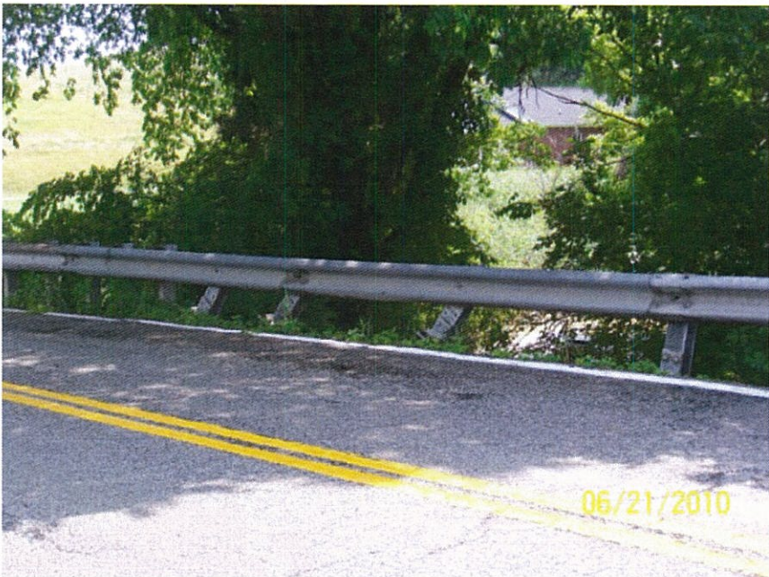
Railing posts are mis-aligned
