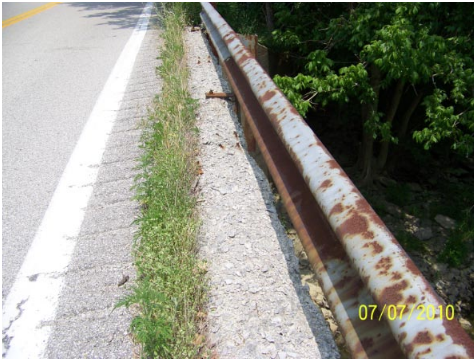
East curb spalled away.
