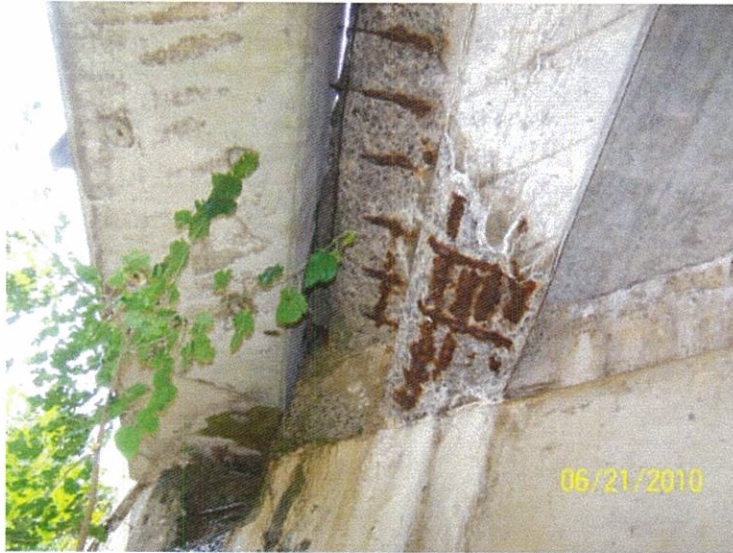
Exposed resteel in bottom of deck at west end
