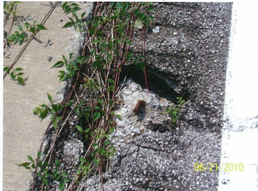
Approximate 20" X 16" hole in deck at west edge
