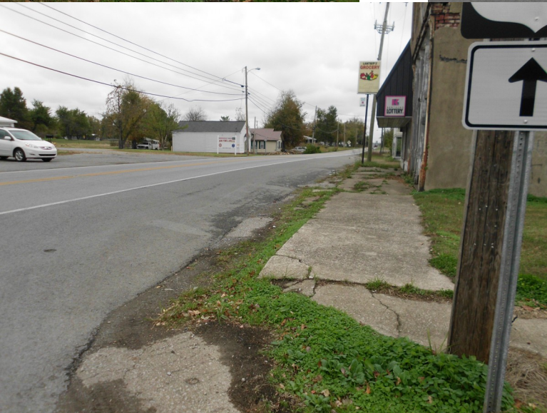
On KY 502 South how far a motorist must pull forward to gain any sight distance
