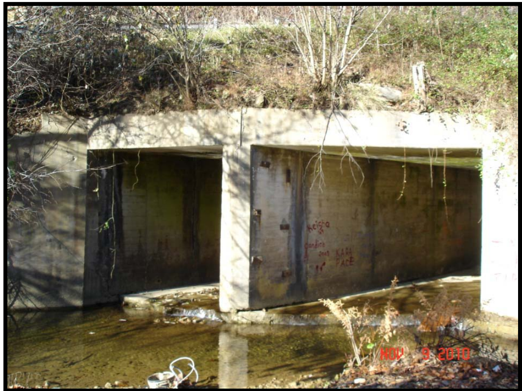
Figure 5: Culvert over Stinnett Creek
