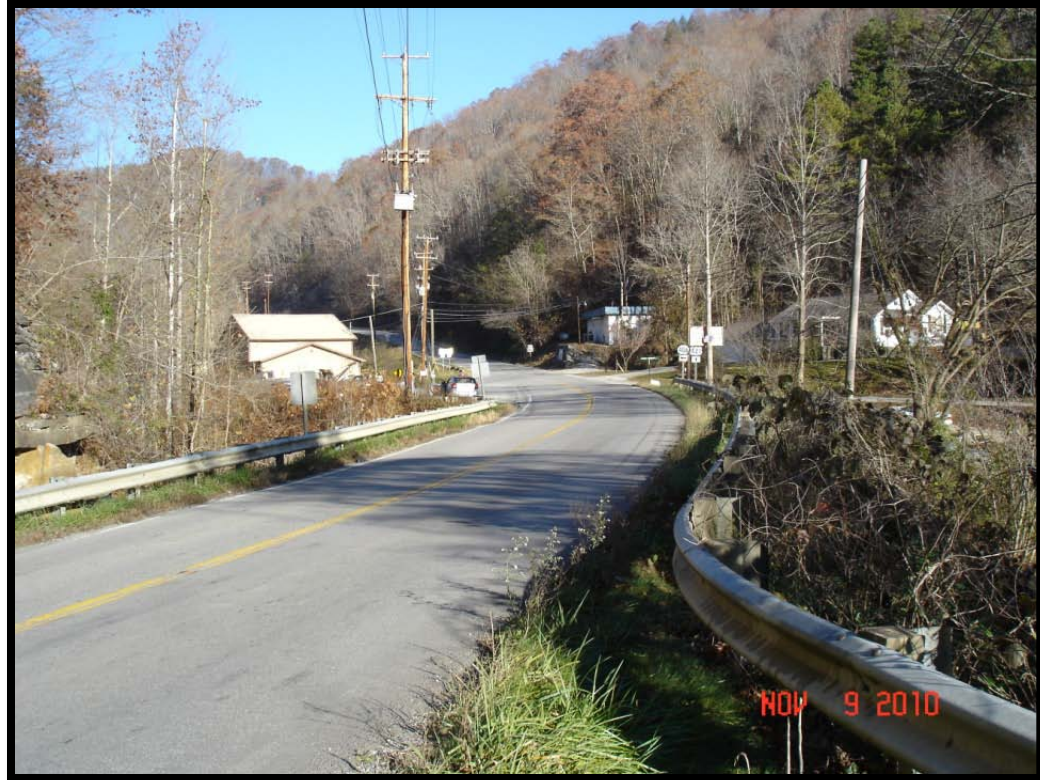
Figure 6: Culvert over Stinnett Creek
