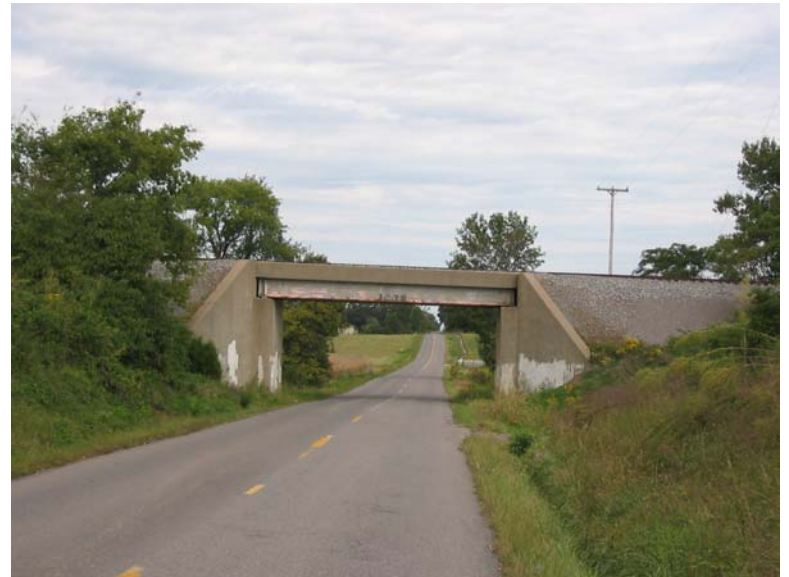
Northbound KY 373 PAL Bridge
