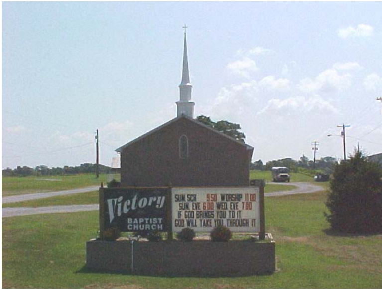
Victory Baptist Church along US 641 north of Eddyville
