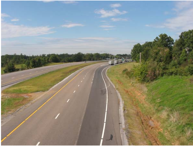
I-24 Weigh Station at Route 810
