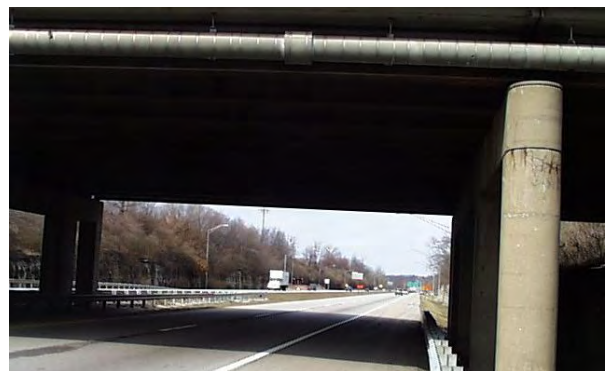
Figure 7 Existing 12" Water Main over I-264
